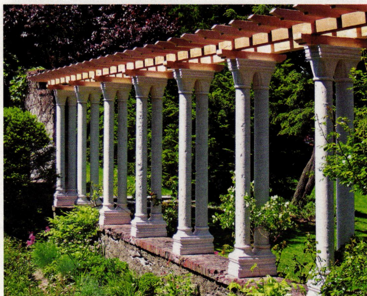
Custom fiberglass twin columns by Goodwin Associates match the originals in this restored pergola.
