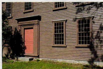
Architectural Components restored the windows, doors and reproduction 18th-century hardware for the Jacob Whittemore House at the Minuteman National Historic Park in Lexington, Mass.
