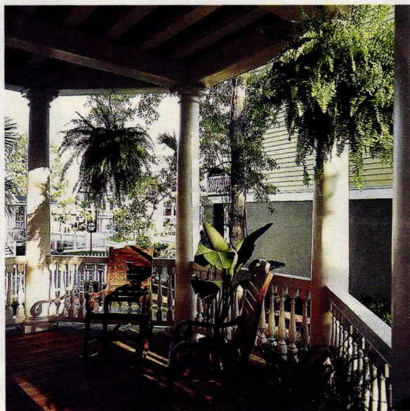
The Chadsworth PolyStone columns on this porch are mirrored in the interior of the house.
