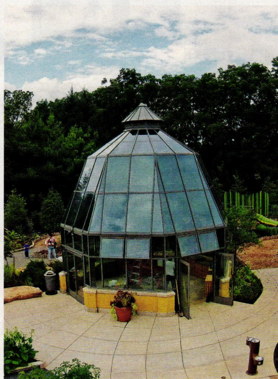
This octagonal greenhouse, fabricated by Glass House, features a custom color powder coat finish, power vented cupola, French doors and high performance glass.
