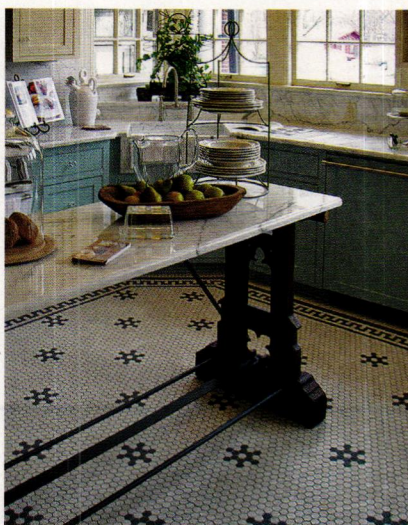
This historically accurate floor was created using 1-in. hexagon unglazed porcelain tile and 3/4-in. square border tile from American Restoration Tile.
