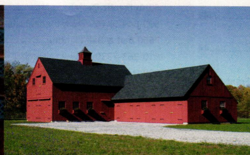
This 1 1/2 story, 22x36-ft. barn and attached 22x36-ft. carriage house were built with a post-and-beam kit from Country Carpenters.
