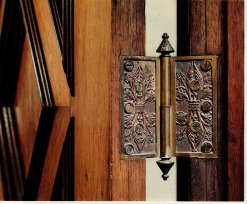
Engraved door hardware original to the building, such as this door hinge and escutcheon plate and knob, were restored.
