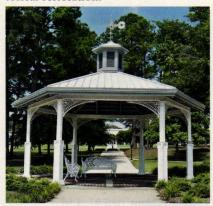
Robinson Iron designed and installed this custom gazebo of cast iron and fabricated waterjetcut steel for the Central Alabama Community College in Alexander, City, AL.
