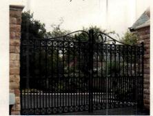
This iron gate for a 12-ft. opening was cast in one piece by Wiemann Metalcraft; it was installed on in-ground hydraulic operators.
