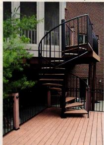
Goddard's custom spiral stairs are available in wood, steel or a combination of both; steel stairs are of welded one-piece construction.
