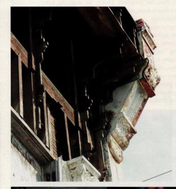
In the Mesker system, sheet metal sections attached to a wood backup. Some areas are specially constructed to support large elements and protruding features. The wood backup on the host Stewardson building was carefully retained as a model, then re-created anew for use on the recipient building in Arcola.
