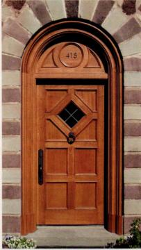
HeartWood Fine Windows & Doors fabricated this 2¼-in. thick mortise-and-tenon solid-wood door out of sawn white oak to replicate the original door made 100 years ago.
