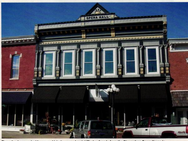
Through a happy coincidence, an historic pressed-metal Mesker façade from the Stewardson Opera House in Stewardson, IL, a building slated to be torn down, found a new home on this historic building in Arcola, IL. The reinstalled Mesker façade is a near-perfect fit on the top half of the Arcola building and an ideal cap to the new period storefront below. All Mesker photos: courtesy of Illinois State Historic Preservation Agency
