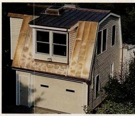
NIKO Contracting installed the copper standing-seam roof on this carriage house.
