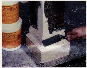
WoodEpox from Abatron can be used to repair wood elements.
