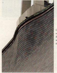
Composite slate roofing from InSpire Roofing was used on this roof.
