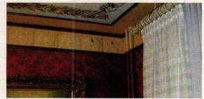
Unico's small-duct, high-velocity HVAC system takes less than ¼ the space of a traditional system, making it ideal for historic buildings.
