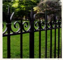
This custom fence was designed and fabricated by Wiemann Metalcraft using solid-bar steel; to ensure longevity, it was galvanized before urethane coating was applied.
