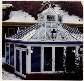
This lantern-roof conservatory by Glass House has an aluminum-clad exterior, which provides a weatherproof barrier for the wood frame.
