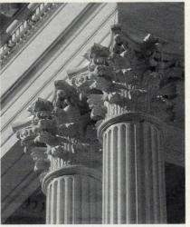
**DeAngelis Iron Wor**k, Inc. supplied and installed 12 cast-iron capitals for the exterior restoration of the Massachusetts State House. *Click on No. 1023*
