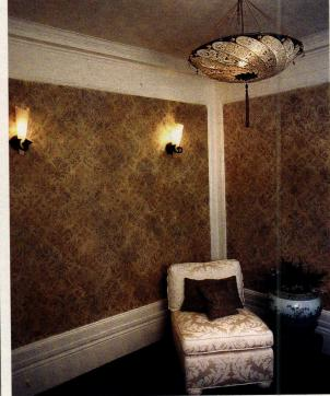
This design by Lynne Rutter, derived from Venetian fabric patterns, was stenciled with metallic powders and overglazed with several different colors of paint.
