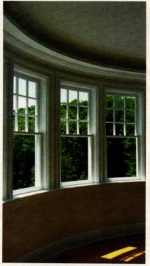
Wood Window Workshop manufactured these custom bent double-hung wood windows with true divided lights and radiused glass for a building in Connecticut. Click on No. 9640
