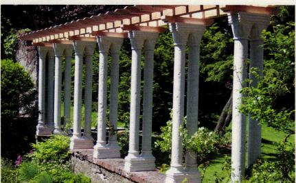
Custom fiberglass twin columns by Goodwin Associates match the originals in this restored pergola. Click on No. 806
