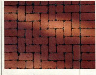
The RainPave brick pattern from **Pine Hall Brick** is made of a rumbled clay paver that allows rain water to filter down to the soil.
