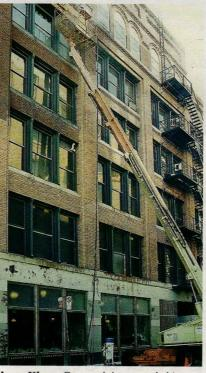
**ArmaKleen Co.** used Armex, a baking soda-based media, to clean the Boydel Building in Detroit, MI. *Key in no. 406*
