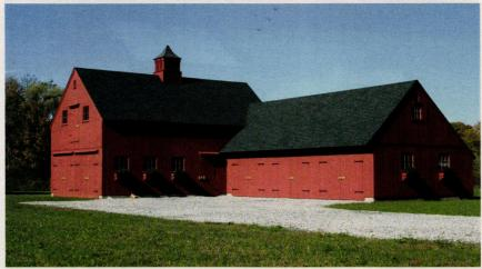
This 11/2 story, 22x36-ft. barn and attached 22x36-ft. carriage house were built with a postand-beam kit from Country Carpenters. Key in. no. 1439
