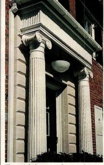
The capitals that crown these exterior columns were fabricated by **Fischer & Jirouch**. *Key in no. 1960*
