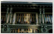
Allen Architectural Metals replicated and restored the cast-iron facade and railings for this 140,000-sq.ft. 1909 Beaux-Arts landmark building in New York City.
