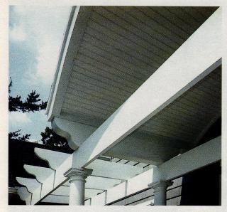
This custom pergola from **Goodwin Associates** uses girders and cross rafters of reinforced board that is maintenance-free and rot-resistant. *Key in no. 806*
