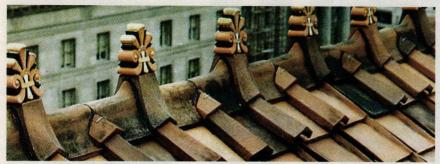
**Boston Valley Terra Cotta** restored and replicated the roof tile for the Department of Justice Building in Washington, DC. *Key in no. 160*
