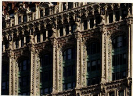
Boston Valley Terra Cotta repaired and restored the terra-cotta facade at 90 West St. in New York City after it was damaged during 9/11. Key in no. 160
