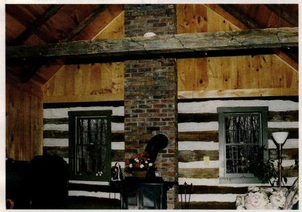
This 45x34-ft. barn was constructed by Sylvan Brandt using four bents and eight major outside posts, most of which are hand-hewn hardwood. Key in no. 3950
