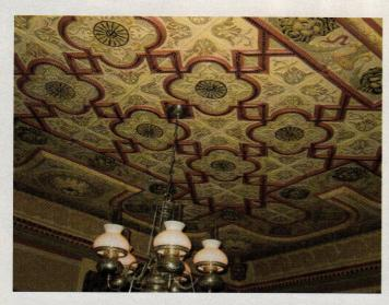
This Orientalstyle ceiling was created using pressed-tin panels from **W.F. Norman Corp.** *Key in no. 520*
