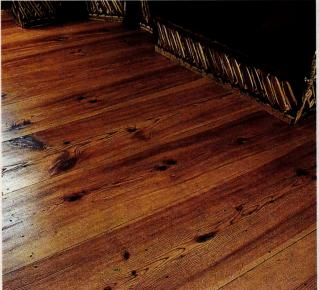
**Craftsman Lumber** manufactured this wide-plank red pine flooring, which was dried and machined onsite. *Key in no. 4320*
