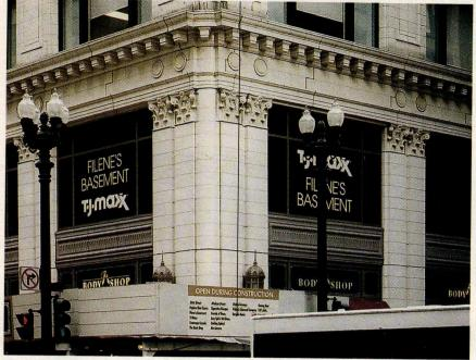
The terra-cotta elements on this commercial building in Chicago were replicated with GFRC elements with technology provided by **Ball Consulting**. *Key in no.* 7260
