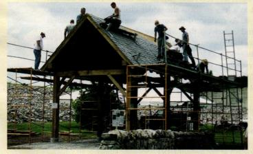
Members of the Slate Roof Contractors Association apply handshapped "fish scale" slates to the timber-frame shelter constructed during the 2009 Preservation Rendezvous in Frankfort, Kentucky.
