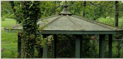
This gazebo features **W.F. Norman Corp.**'s Style "A" shingles with its continuous hip finish and a custom-made finial on top. *Key in no. 520*
