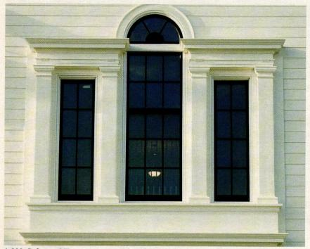
**1.800. Columns'** Tuscan non-tapered Architectural Polystone pilasters frame this Serliana window. *Key in no. 1580 for PolyStone; 180 for wood*
