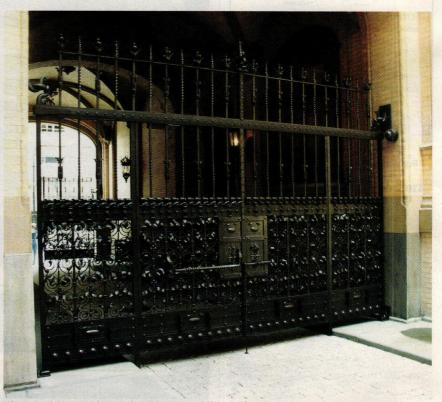
Fine Architectural Metalsmiths created this 10-ft. tall double-pedestrian gate with side panels for a landmark building in New York City. Key in no. 2640
