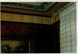
**Unico**'s small-duct, high-velocity HVAC system takes less than ¼ the space of a traditional system, making it ideal for historic buildings. *Key in no.* 1779
