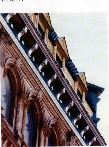
This stamped-sheet-metal cornice was fabricated by **W.F. Norman**. Write in No. 520
