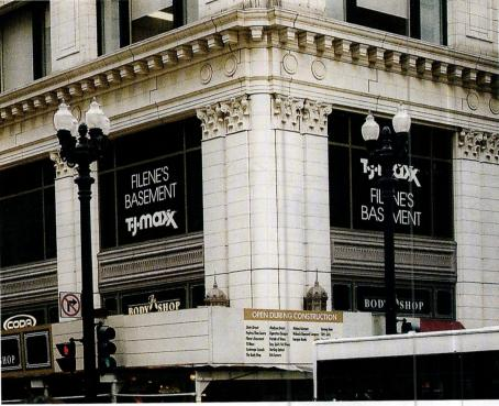
The terra-cotta elements on this commercial building in Chicago were replicated with GFRC elements with technology provided by **Ball Consulting**. Write in No. 7260
