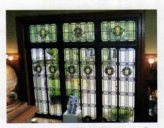
An interior storm from **Climate Seal** provides insulation while protecting the appearance of this historic window.
