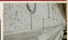
Low visibility Post & Wire systems are an effective barrier deterrent for pigeons on narrow ledges.
