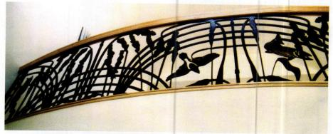
This elaborate railing was made of ½-in. steel panels cut by Colorado Waterjet.
