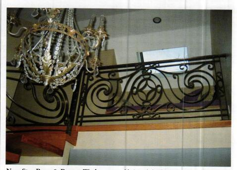
New Star Brass & Bronze Works custom fabricated this hand-forged bronze stair and balcony railing for a building in Long Island, NY. Write in No. 3051
