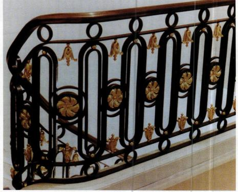
This stair balustrade, fabricated by Schwartz's Forge & Metalworks, has gilded repousse leaf work and a custom bronze cap rail. Write in No. 1218
