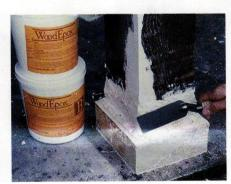
WoodEpox from **Abatron** can be used to repair wood elements such as this column. Write in No. 1300
