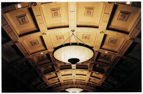
**Flex Moulding** used polyester resin to create this ornate barrel-vaulted ceiling. *Write in No. 4900*
