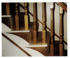
These balusters and stair-tread brackets are examples of the wide variety of architectural millwork fabricated in premium hardwoods by **Cumberland Woodcraft**. *Write in No. 1310*
