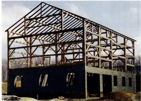
This ca. 1830 timber frame was relocated by **Eagle Creek Designs** from Ohio to Pennsylvania for use as a horse barn. *Write in No. 529*
