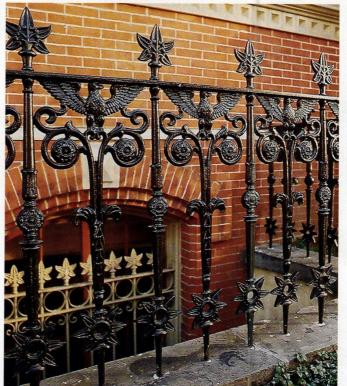
This 2-ft.-tall railing in cast iron was created for a building in Washington, DC, by Historical Arts & Casting. Write in No. 1210
