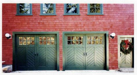
Hahn's Woodworking custom manufactured these overhead motorized garage doors, which give the appearance of swing-out carriage-house doors, and the complementary door (right). Write in No. 6640
