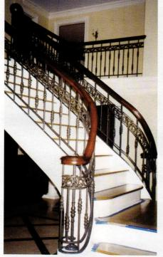
This cast-iron and cherry stair railing is the work of John F. Graney Metal Design. Write in No. 4840
