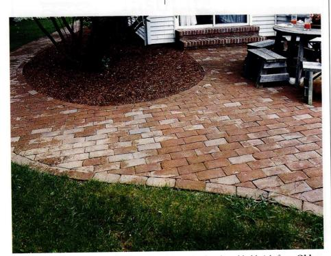
This running-bond-style paving was created by using hand-molded brick from **Old Carolina Brick**. Write in No. 3130
