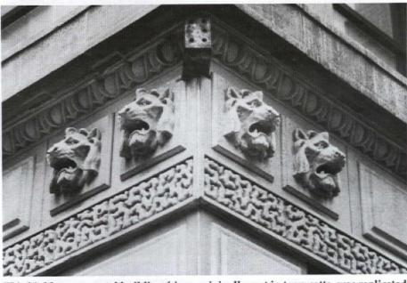
This highly ornamental building frieze, originally cast in terra cotta, was replicated in GFRC panels by GFRC, INC. Write in No. 663
