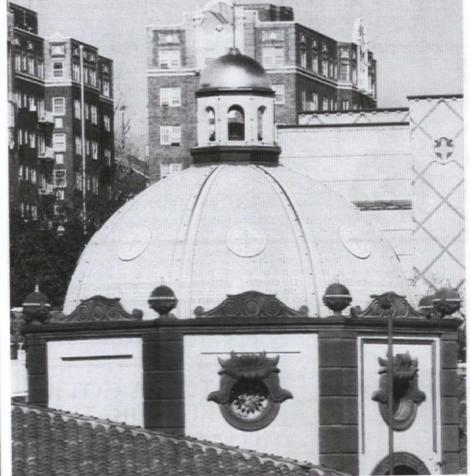
The ornament for this elaborately detailed facade in Kansas City, Mo., was fabricated in cast stone by TERRA COTTA & CAST STONE. Write in No. 187
