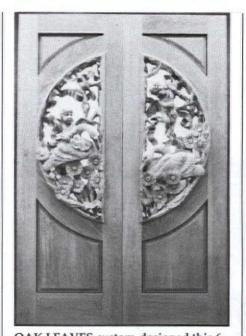
OAK LEAVES custom-designed this 6-ft. 8-in. H. x 4-ft. 6-in. W. x 6-in. D. limed white oak doors for a client who liked cherubs, swans, and daisies. Details include a stained glass window in back of the carving, cut and polished geodes (at the bottom), bells with goldleaf balls ring when the doors are opened and closed, English wrought iron doorknobs, and an abraded gold leaf finish. Write in No. 122
