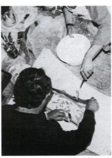
RORY BRENNAN, a specialist in restoring plaster and other molded ornament, is shown here creating a mold from a section of historic molded plaster. Write in No. 298
