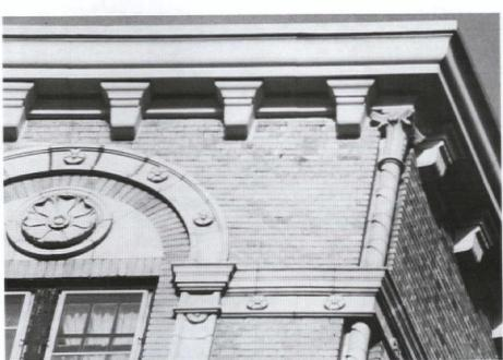
This fiberglass replication of a terra cotta cornice on a New York City building was engineered and fabricated by ARCHITECTURAL FIBERGLASS CORP. Write in No. 640
