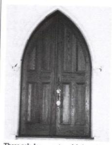
These oak doors, custom-fabricated by LAMSON-TAYLOR DOORS, are 5 ft. W x 9 ft. H. x 2-1/4 in. D. with raised moldings, flat panels, Ian Eddy hardware, and astragal jamb. Write in No.
