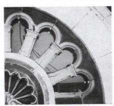
Custom System 45 from EDISON CHEMICAL SYSTEMS was used to restore these severely cracked and spalled terra cotta columns on a half-round window in the facade of Bank-center South, Savannah, Ga. The material was used for patches, to rebond broken pieces, and to cast missing elements. Write in No. 215
