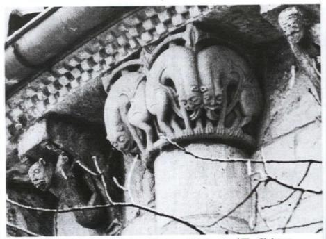
For the apse of the Chapel from Fuentideuna, which is part of The Cloisters, Fort Tryon Park, N.Y., LANDMARK STUDIOS created cast-stone replicas of the deteriorated original capitals for replacement and record. Write in No. 190
