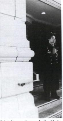
Painted terra cotta reproduction blocks for this hotel entry in Portland, Ore., were molded by ARCHITECTURAL REPRODUCTIONS as individual units using Forton MG, a polymer-modified glass-fiber reinforced gypsum (GRG). Write in No. 613
