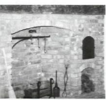
Company designs and builds Rumford fireplaces, the shallow, heat-reflective units developed by Count Rumford in the 1790's. Supplies parts, plans, and consultations. Shown is a Rumford cooking fireplace with working bread oven.
