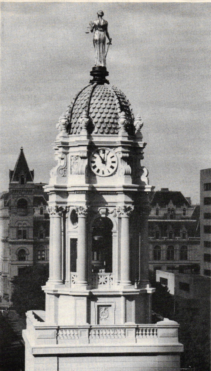
The restored dome of Brooklyn Borough Hall rests securely under its helmet of 650 new handmade patinated copper shingles.
