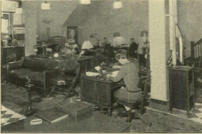
IN A PUBLIC UTILITY . . . Brooklyn (N. Y.) Edison Co. One of nine public utility installations. When handling high voltage lines. "Men at work" has special significance. Pneumatic Tubes swiftly carry vital orders.
