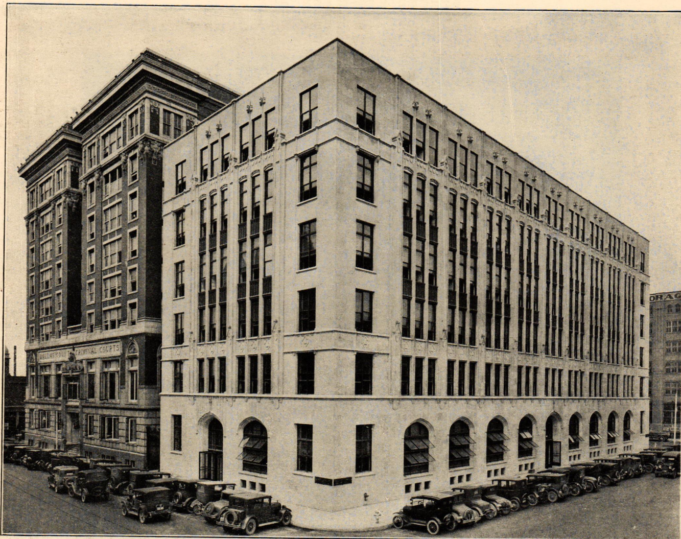
County Hall of Records, Dallas, Texas. Lang & Witchell, Architects. C. L. Shaw, Builder. Built of Gray Indiana Limestone.
