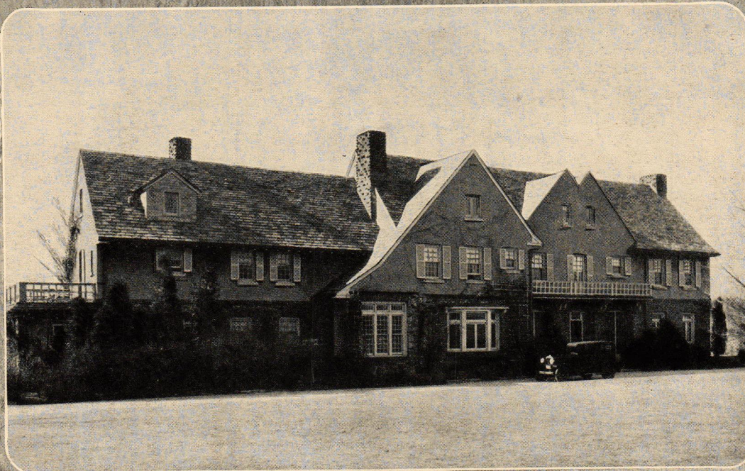
Residence at Rye, New York, Reroofed with Tudor Stone Henry Toombs, Architect for renovations
