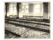
Showing how the Underfloor Duct grid provides wireways to all parts of the floor.
