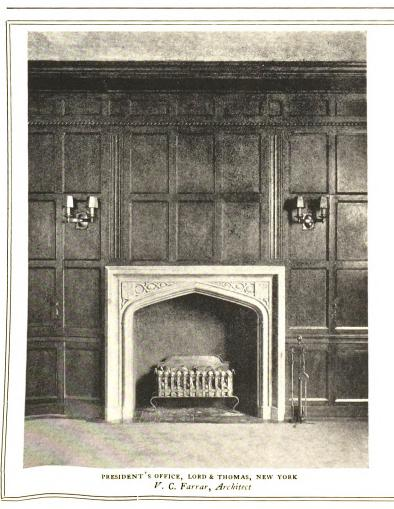
This illustration is an example of the range and versatility of our services. The wainscoting is executed in Duretta, an exact, fireproof reproduction of wood. Duretta may also be used as a substitute for metal in making radiator grilles and other objects.
