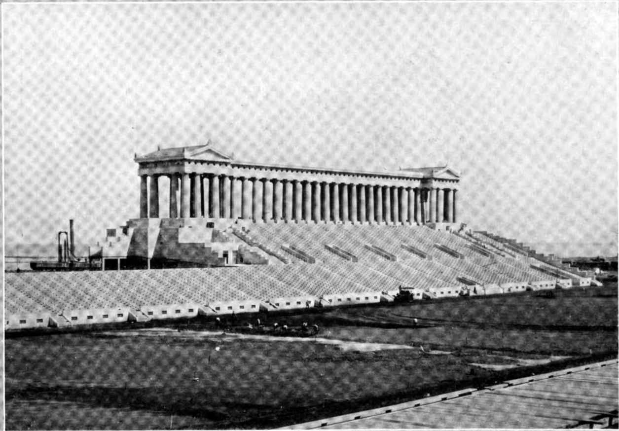
Grant Park Stadium, Chicago. Holabird & Roche, Architects
