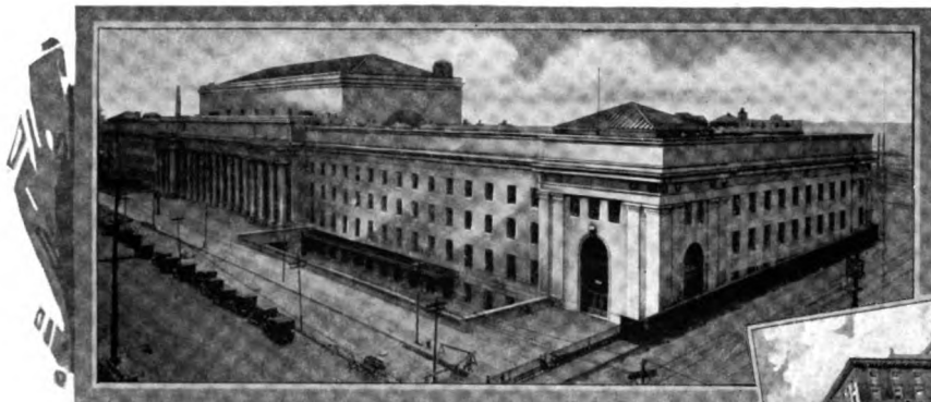
Toronto Union Station, Ross & MacDonald, Architects
