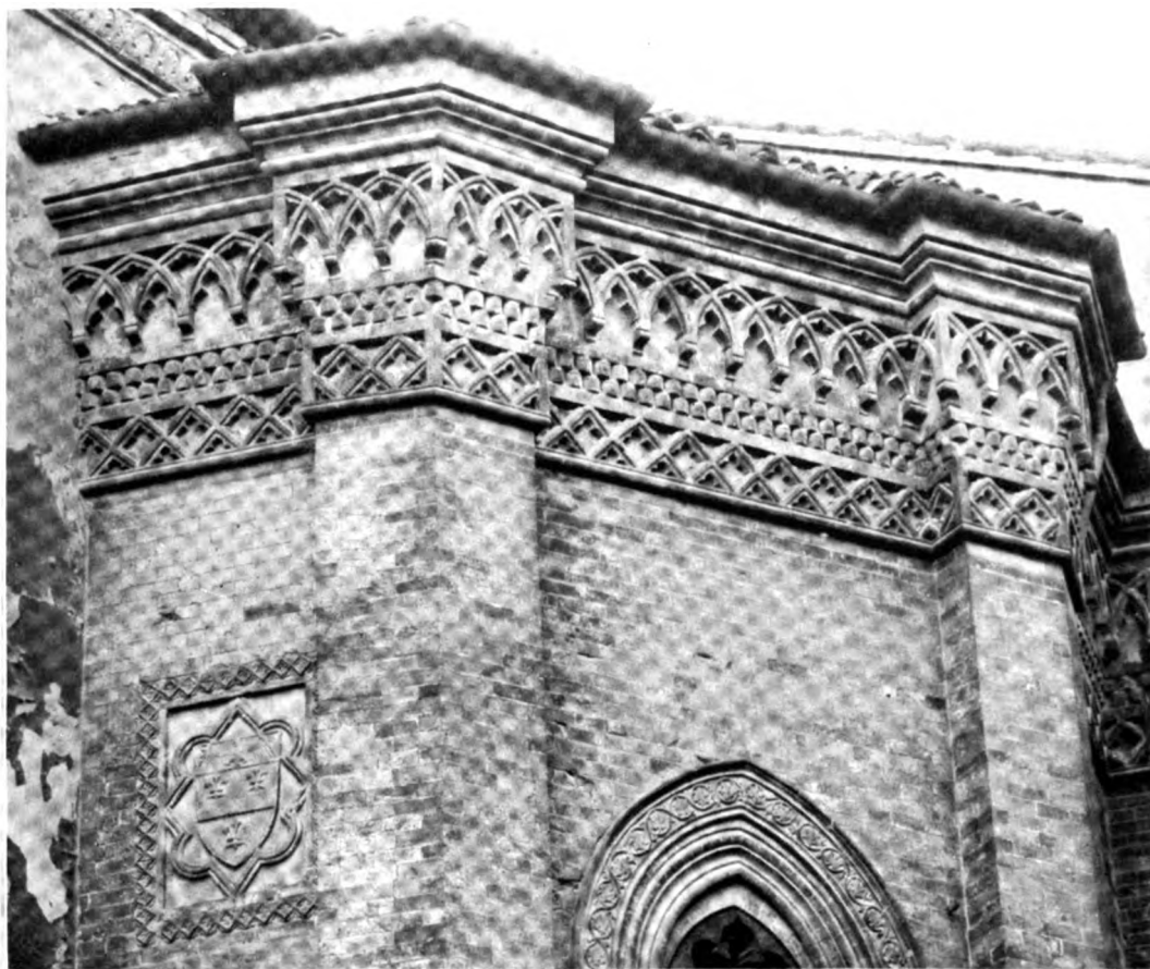
Terra Cotta Cornice of Small Chapel, Cathedral at Parma, Italy (From a revised and enlarged edition of "Color in Architecture" published by the National Terra Cotta Society)
