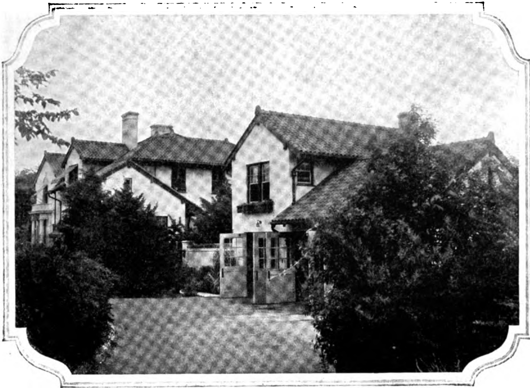
Residence of Mrs. C. P. Adams, Dallas, Texas—H. B. Thompson, Architect
