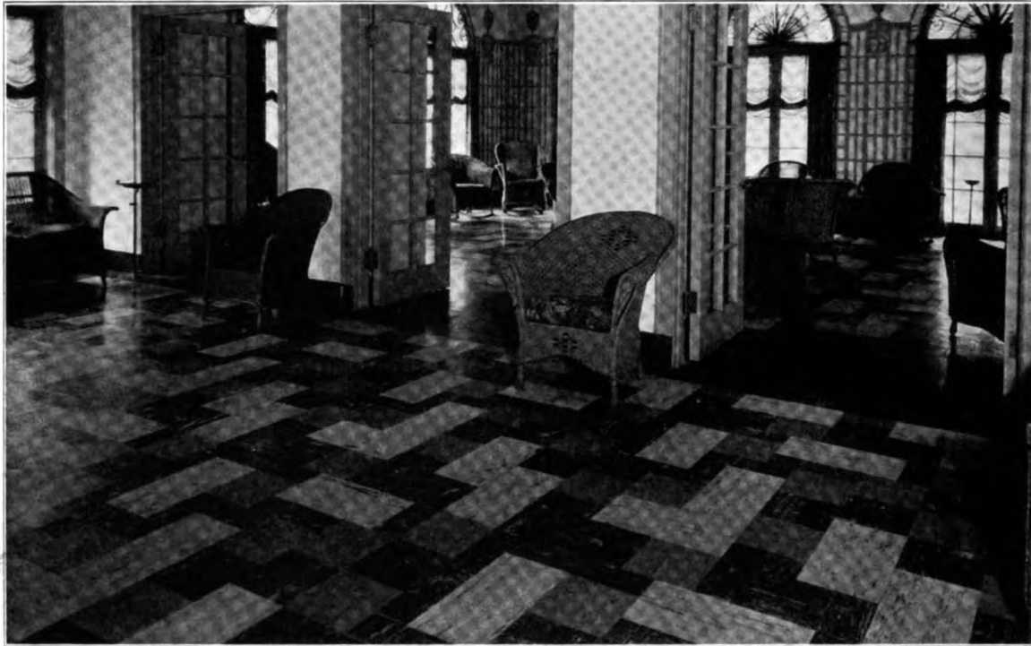
Wright Rubber Tile Floor installed in The Grenada, Chicago Olsen and Urbain, Architects
