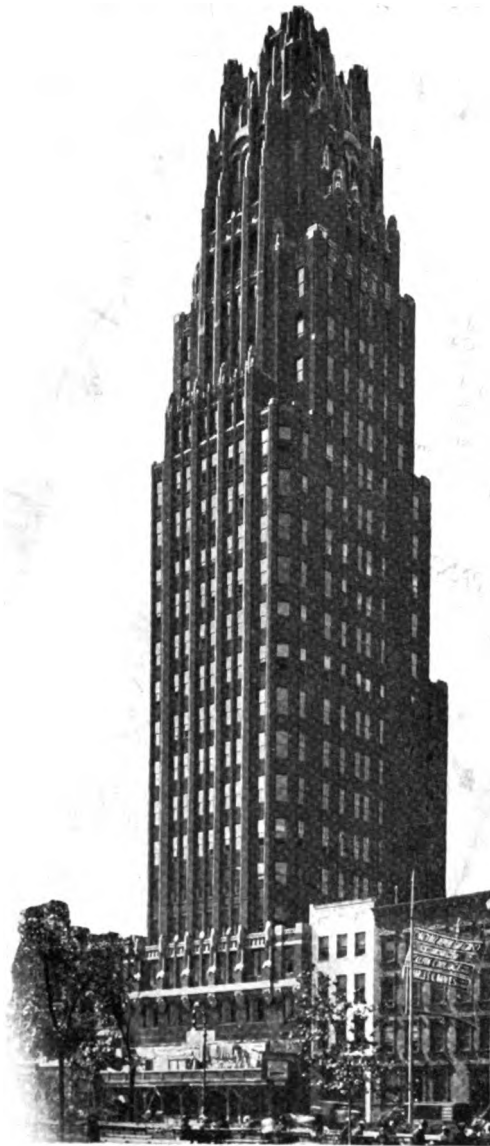
American Radiator Building Raymond M. Hood, Architect Gunn & Borgo, Painters
