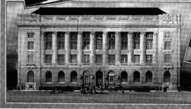
Public Library of City of Cleveland Walker & Weeks, Architects
