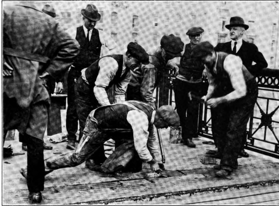
Wright Rubber Sidewalk being laid on Michigan Boulevard Bridge, Chicago, Ill.
