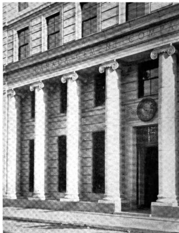
CANADA CEMENT COMPANY BUILDING MONTREAL
