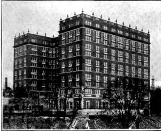
Wade Park Manor, Cleveland (Above) (G. B. Posts & Sons, Architects— W. G. Cornell & Co., Plumbers) Equipped throughout with Whale-Bone- Ite: 262 of type 16-9; 21 of type 23-9.
