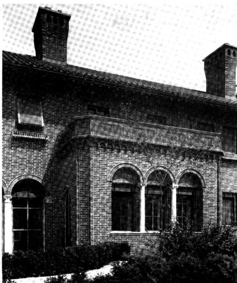
Detail, House, Mr. Isaac Guggenheim, Port Washington, L. I. H. Van Buren Magonigle, Architect
