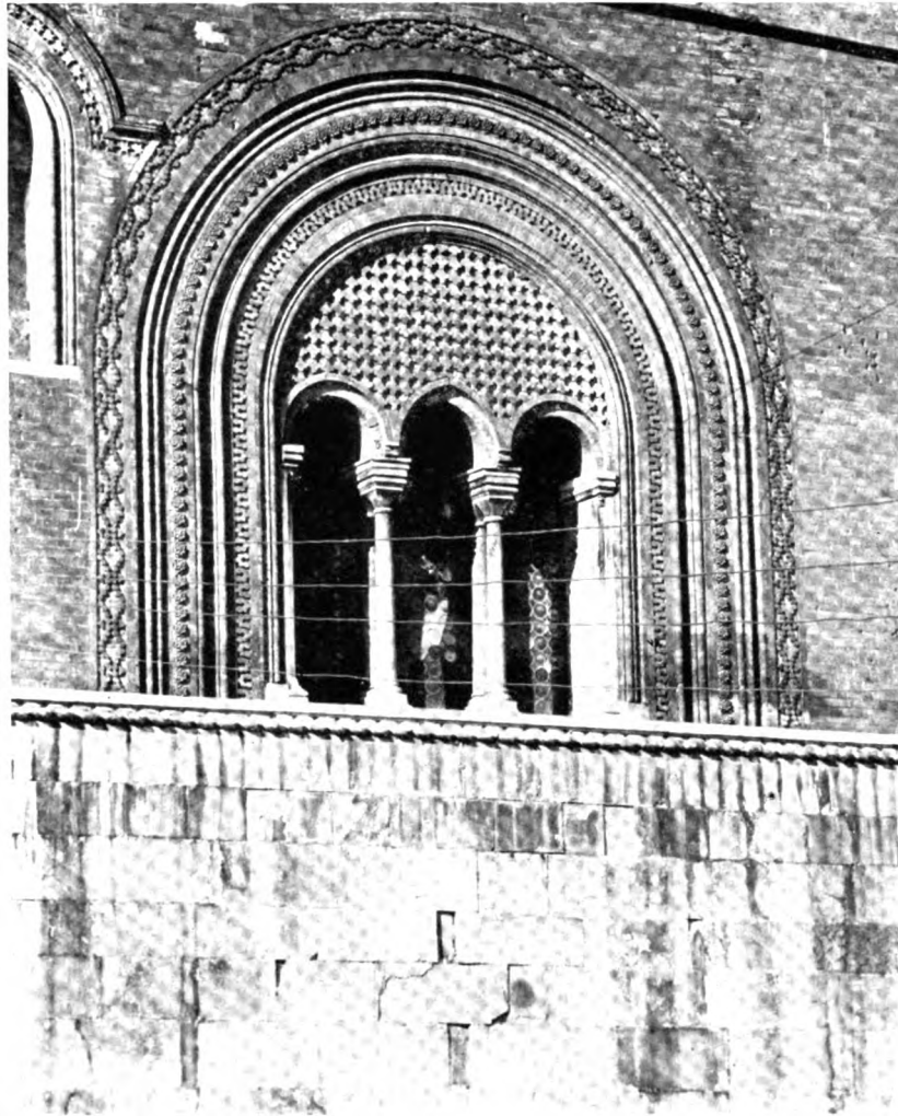
Detail of Terra Cotta windows, Palazzo Municipale, Piacenza, Italy, erected in 1281 A.D.
