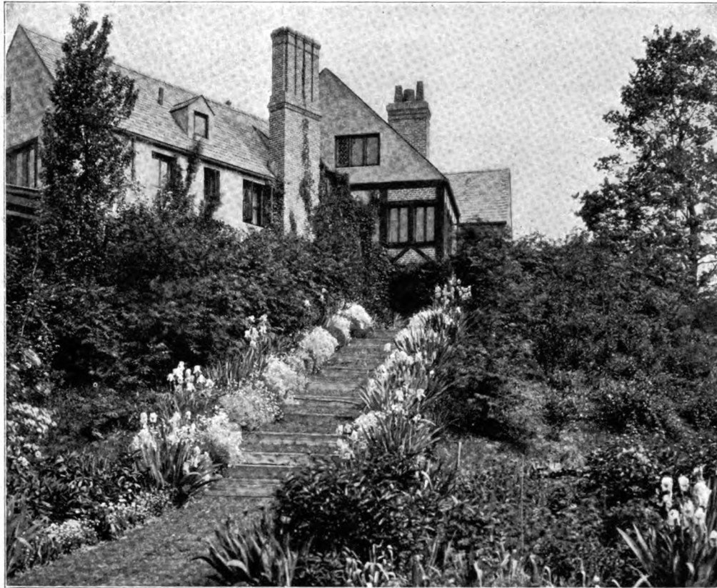
J. R. Thomas Residence, Charleston, West Virginia
