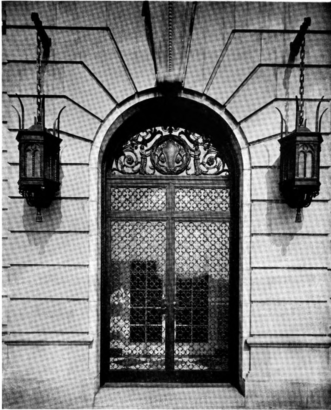
Wrought Iron Entrance and Lanterns, Andrew Freedman Home, New York Joseph H. Freedlander and Harry Allan Jacobs, Associate Architects (See Plates LIII - LVI)
