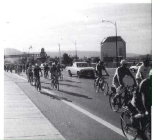
Reconfigured span of Burnside Bridge, with added bicycle lanes.
