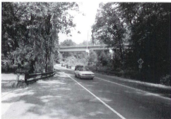
Cresheim Valley Road is part of a network of streets that provide convenient access to Center City, draining ridership from commuter rail lines (one of which runs on the viaduct that crosses the road).
