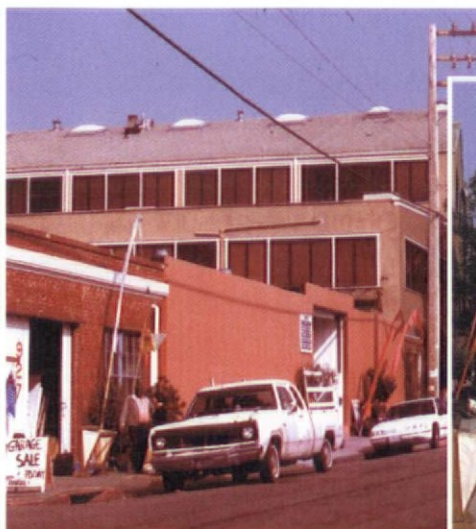
New investment on Tenth Street, in West Berkeley's "mixed use-light industrial district" — live-work units to the left and Nolo Press offices and retail at the right. The Fantasy Records building, behind Nolo Press, was developed earlier.
