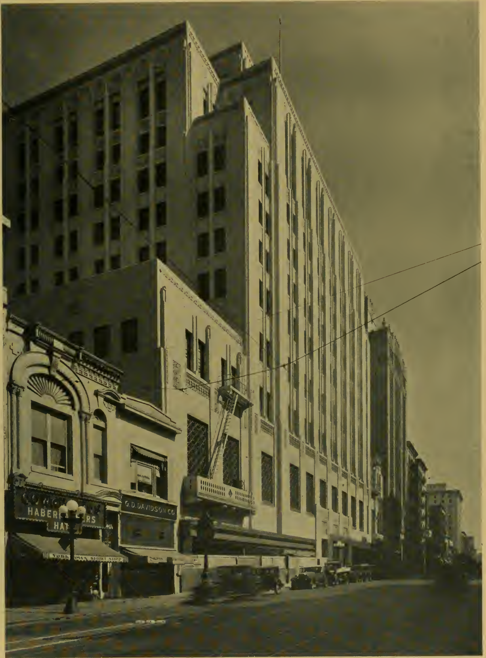
TITLE INSURANCE BUILDING, LOS ANGELES, CALIFORNIA JOHN AND DONALD PARKINSON, ARCHITECTS
