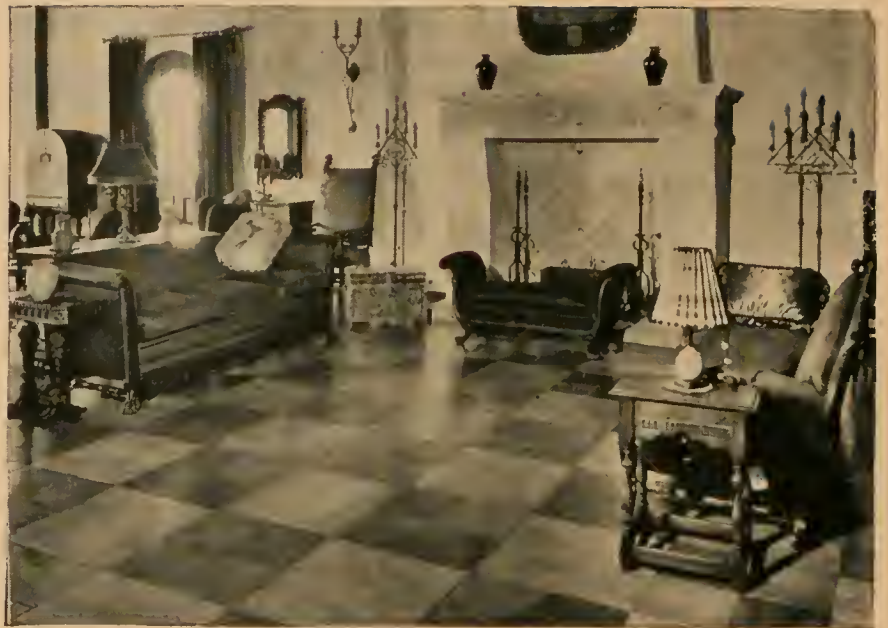
UNRETOUCHED PHOTOGRAPH OF A LAM-ART UNILASTIC FLOOR laid over concrete without the use of a single nail. The large blocks are \frac{1}{2} " thick by 24" square, and the sets of four smaller blocks \frac{1}{2} " x 12" square. Only by lamination is it possible to use blocks of this size with unbroken faces.
