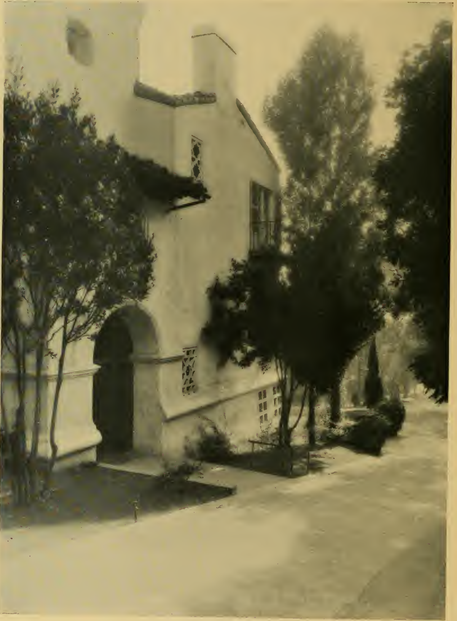
MAIN ENTRANCE, ALPHA PHI SORORITY HOUSE, BERKELEY, CALIFORNIA. W. H. RATCLIFF, ARCHITECT
