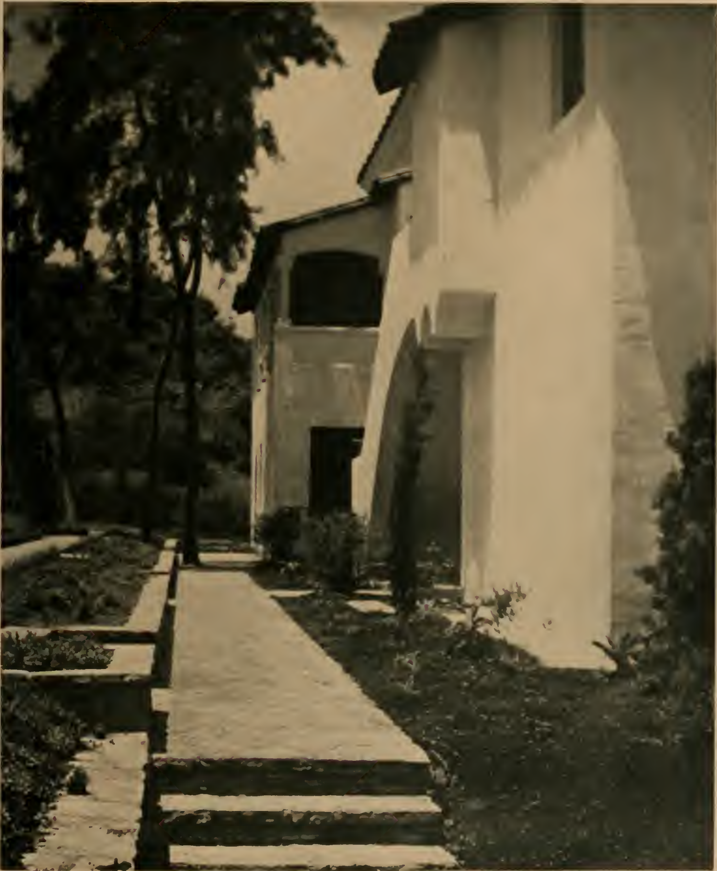
DETAIL, ADMINISTRATION BUILDING, BEL-AIR, CALIFORNIA. DESIGNED BY MARK DANIELS
