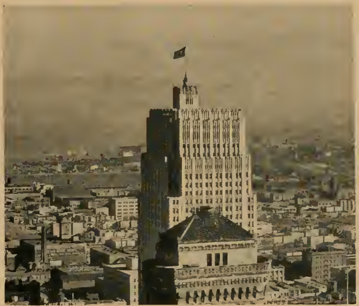
A steel flag pole arises from the top of the Pacific Telephone and Telegraph Building, San Francisco. Miller and Pflueger, Architects
