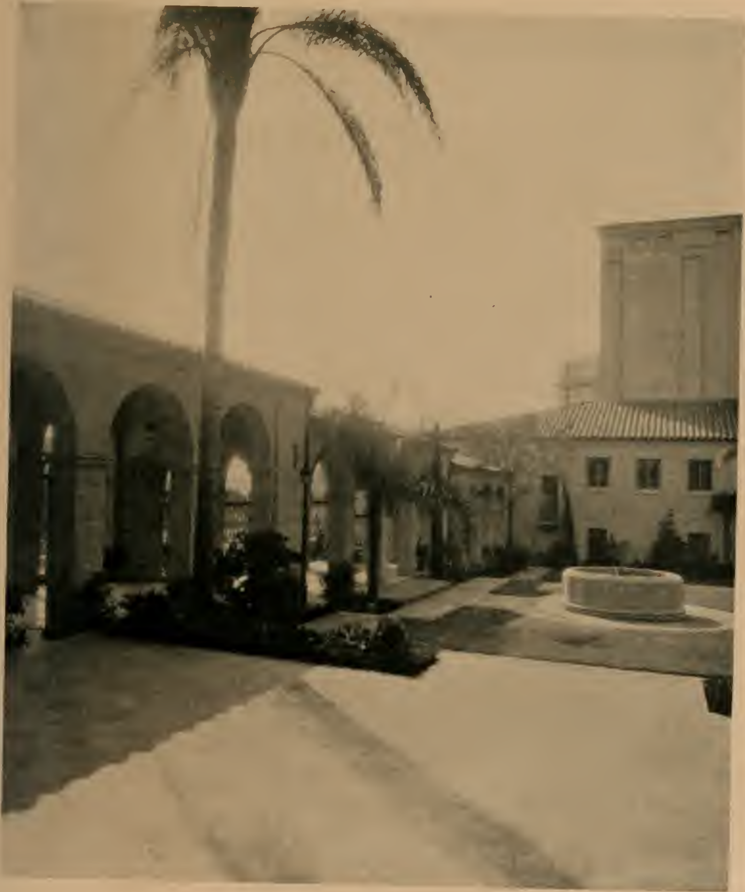
ARCADE FROM PATIO, EBELL CLUB, LOS ANGELES, CALIFORNIA HUNT AND BURNS, ARCHITECTS
