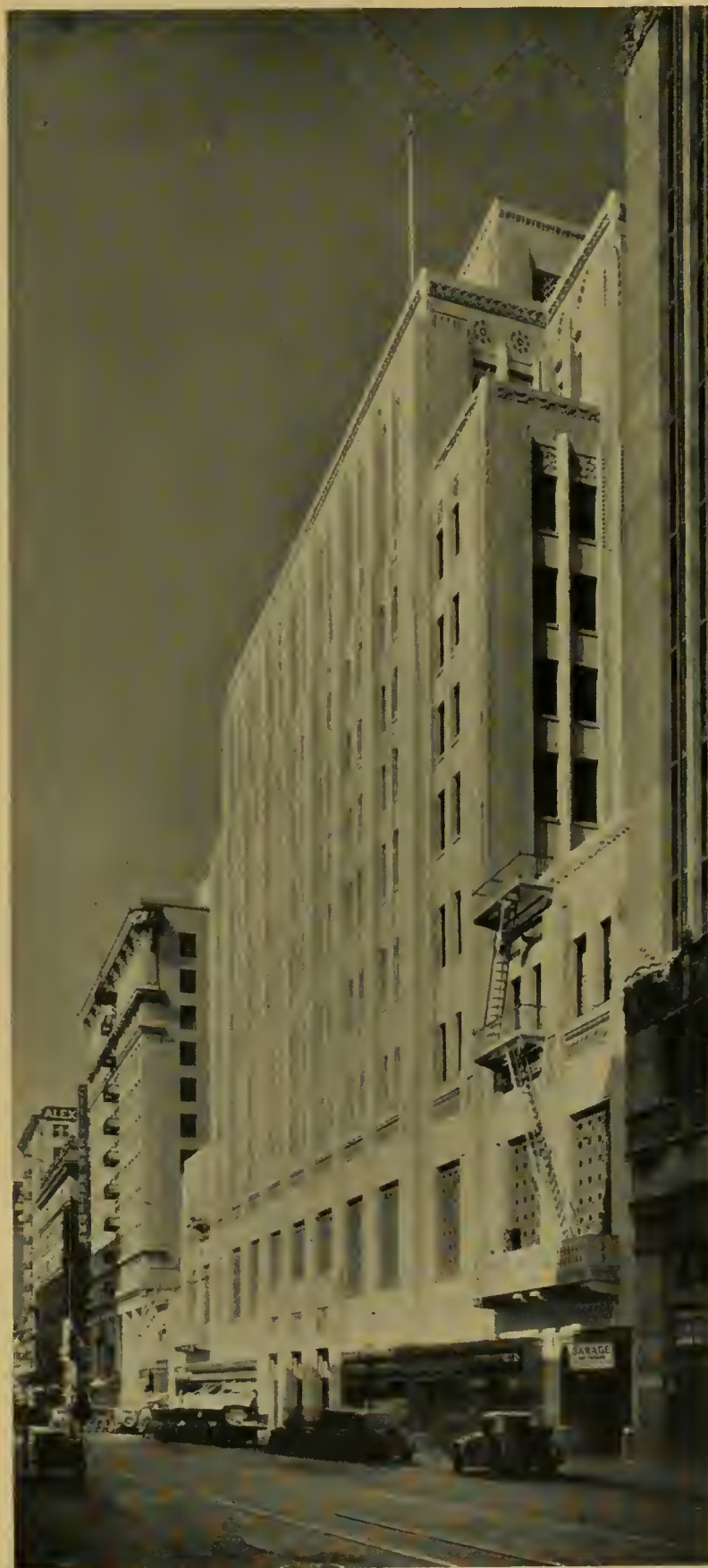
Title Insurance Building, Los Angeles, California John and Donald Parkinson, Architects
