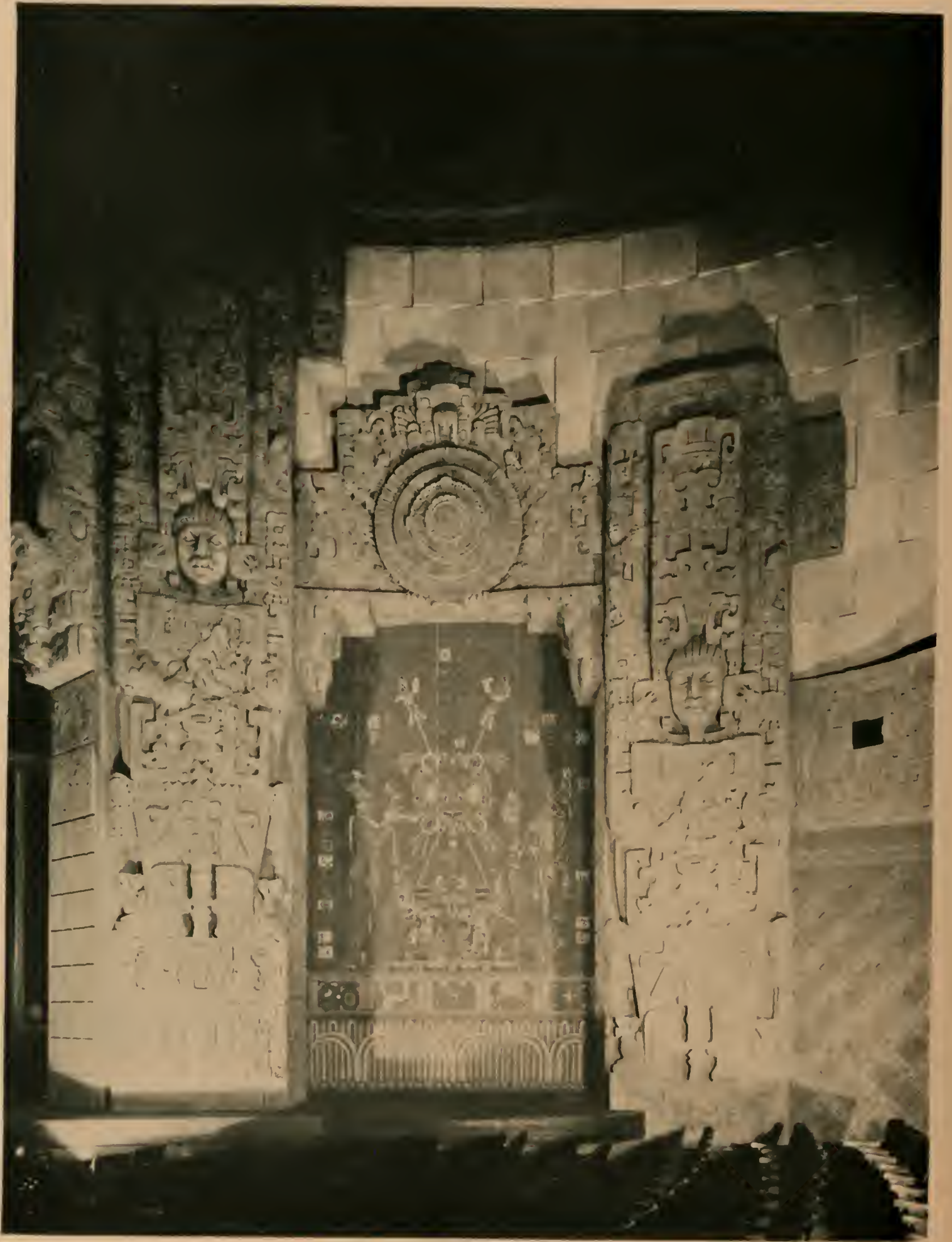
SIDE STAGE DETAIL, MAYAN THEATRE, LOS ANGELES, CALIFORNIA MORGAN, WALLS AND CLEMENTS, ARCHITECTS
