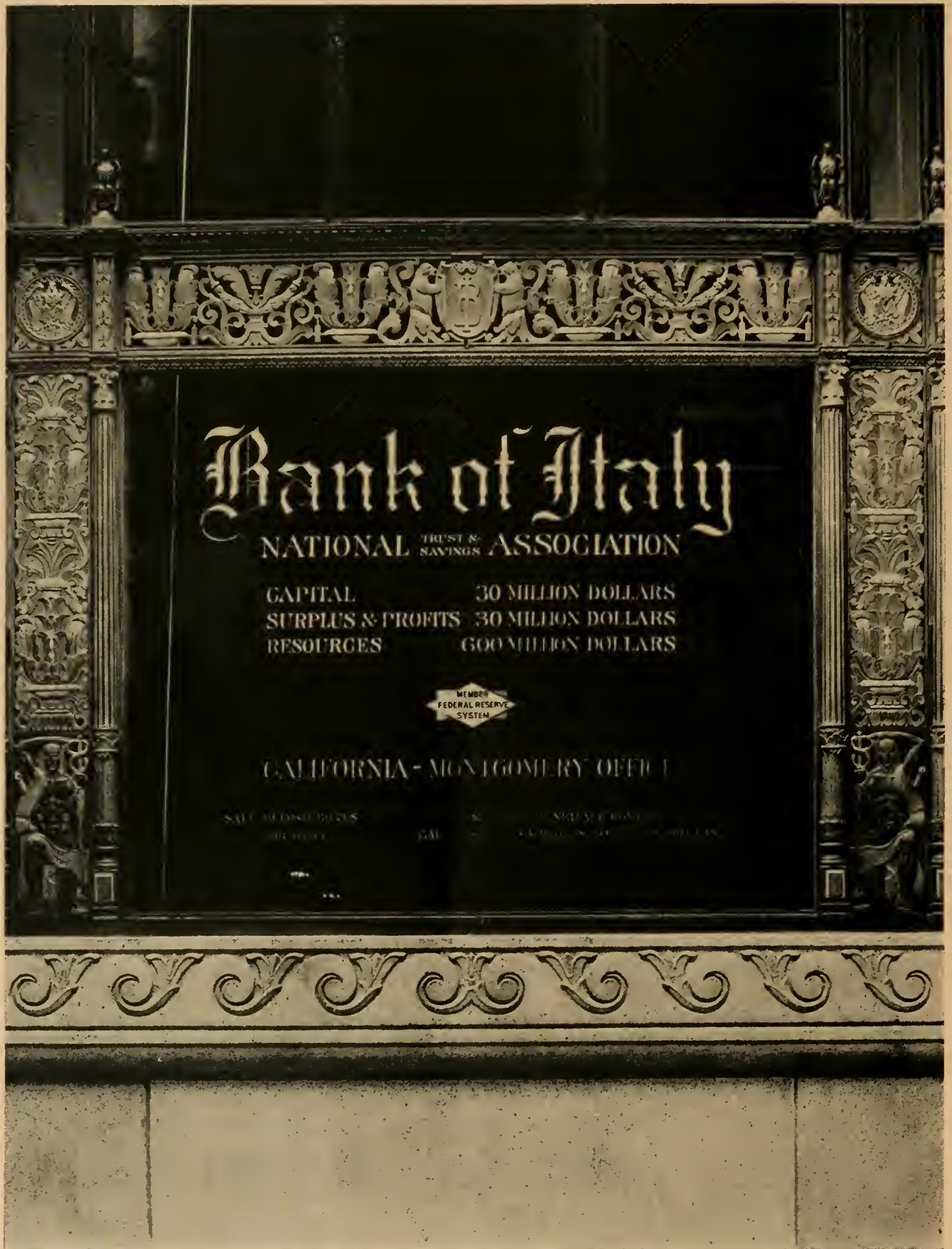
WINDOW DETAIL, BANK OF ITALY, SAN FRANCISCO. H. A. MINTON, ARCHITECT.
