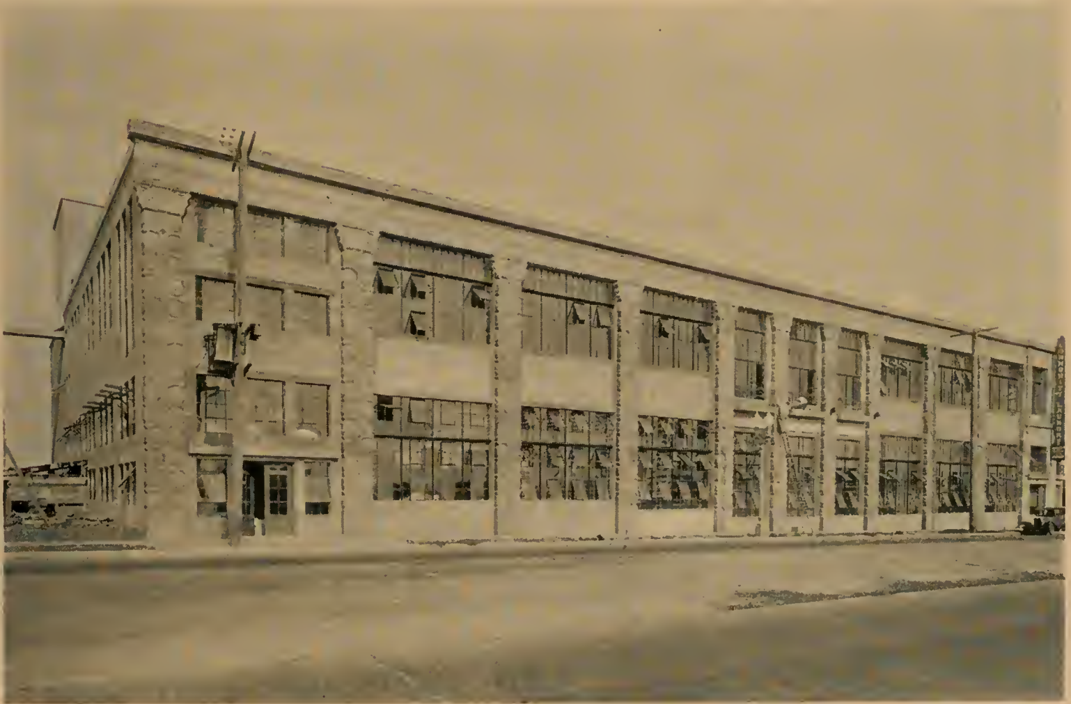
COMMUNITY LAUNDRY, LOS ANGELES, CALIFORNIA. W. J. SAUNDERS, ARCHITECT
