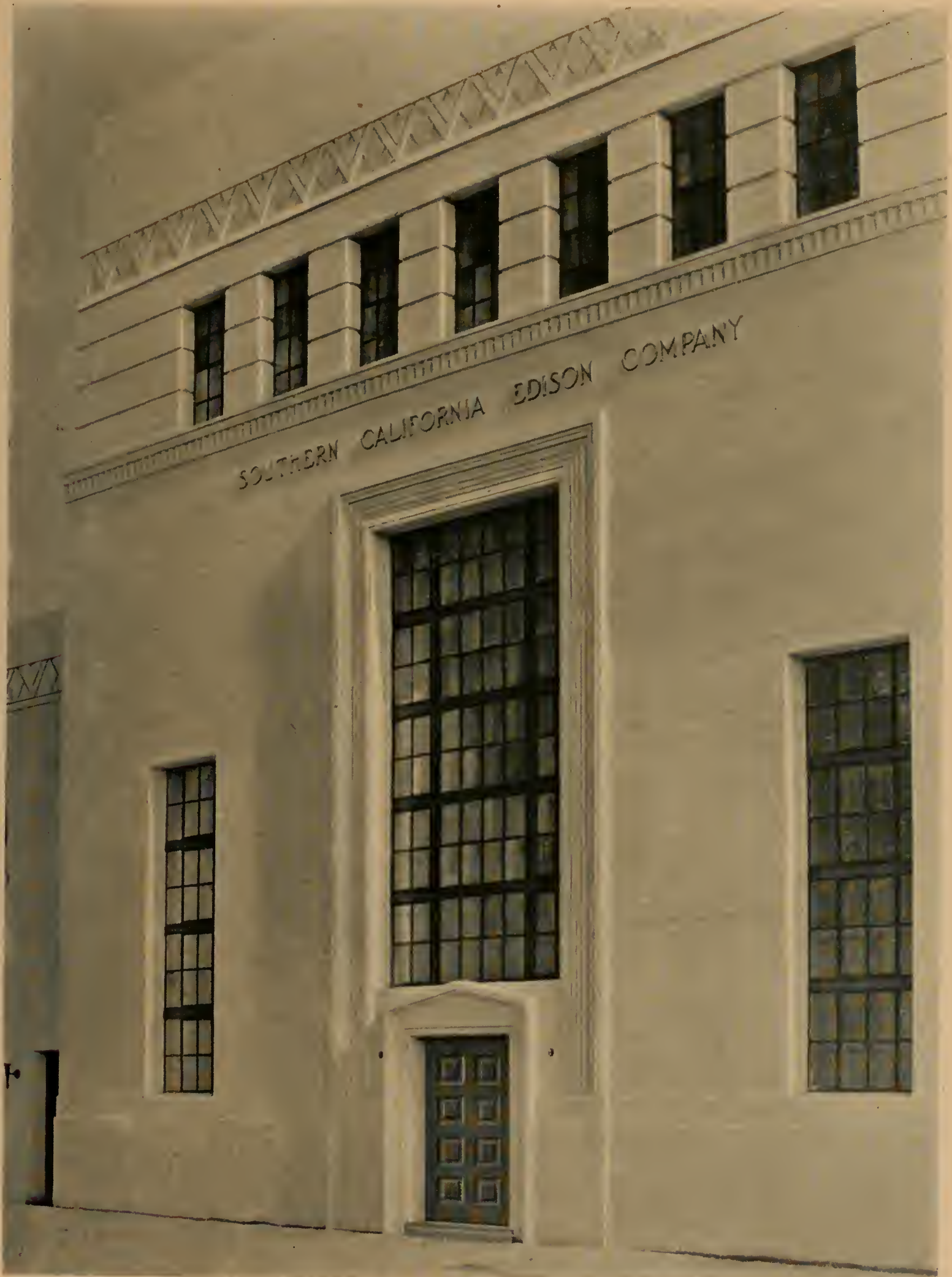
SUB-STATION, SOUTHERN CALIFORNIA EDISON COMPANY, LOS ANGELES, CALIFORNIA HUNT AND BURNS, ARCHITECTS
