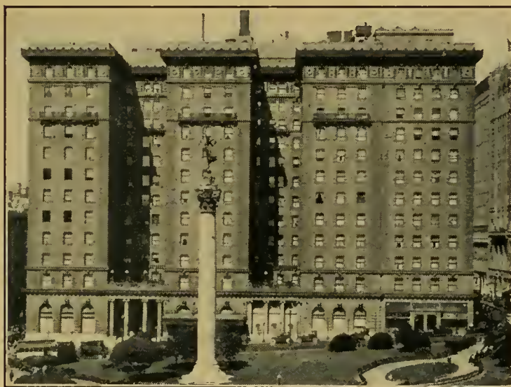
St. Francis Hotel, San Francisco — comfortably, economically heated with oil and uses Johnson oil burning equipment in its kitchen. Where comfort and efficiency is paramount you find Johnson installations.
