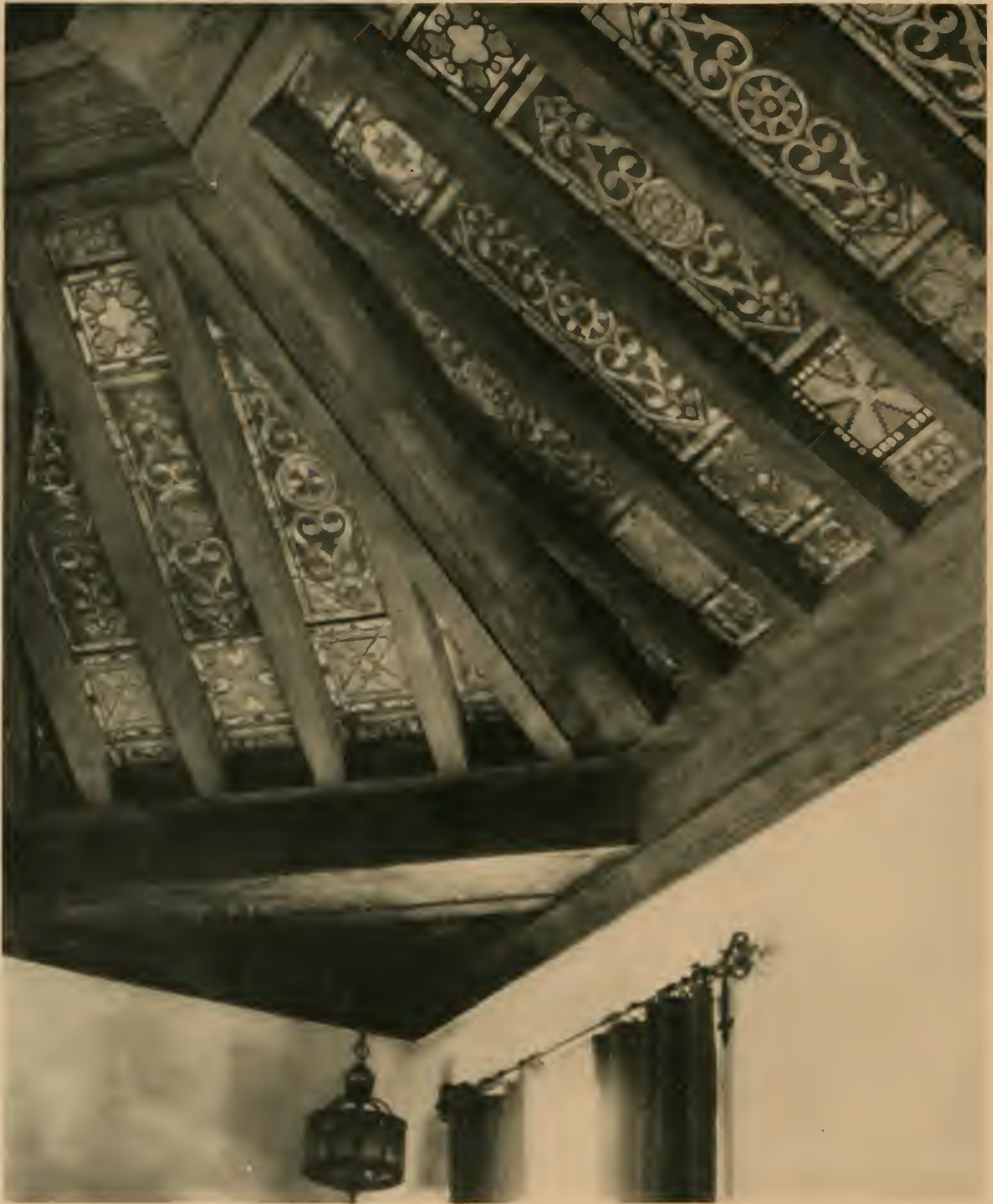
CEILING IN ADMINISTRATION BUILDING, BEL-AIR, CALIFORNIA. DESIGNED BY MARK DANIELS
