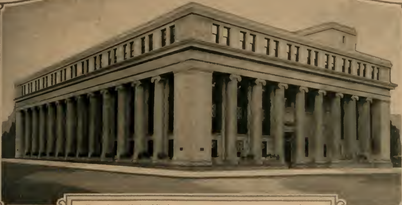
The Colorado National Bank . . . . . Denver Wm. E. and Arthur A. Fisher and M. H. Hoyt . . . . . Architects
