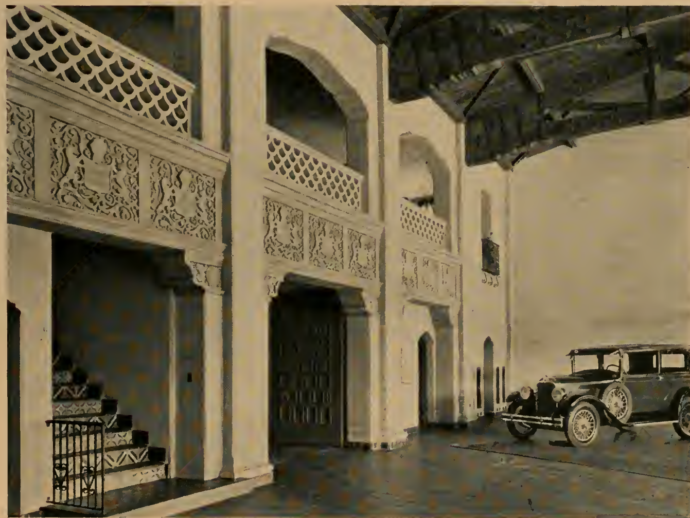
HOWARD MOTOR COMPANY BUILDING, PASADENA, CALIFORNIA DESIGNED BY AUSTIN COMPANY
