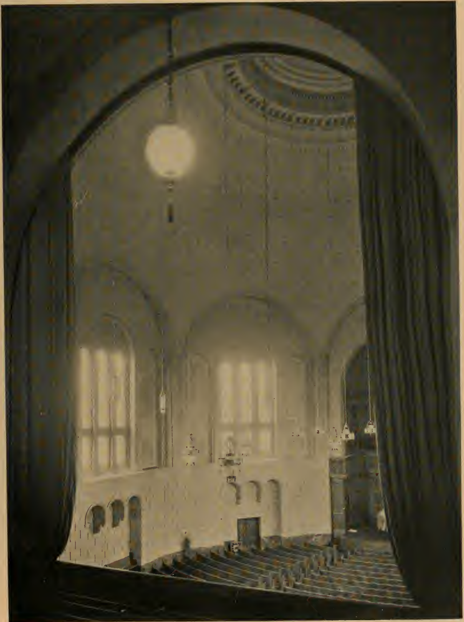
AUDITORIUM FROM BALCONY, TEMPLE BETH ISRAEL, PORTLAND, OREGON. MORRIS H. WHITEHOUSE AND HERMAN BROOKMAN, ASSOCIATE ARCHITECTS; JOHN V. BENNES AND HARRY HERZOG, CONSULTING ARCHITECTS.
