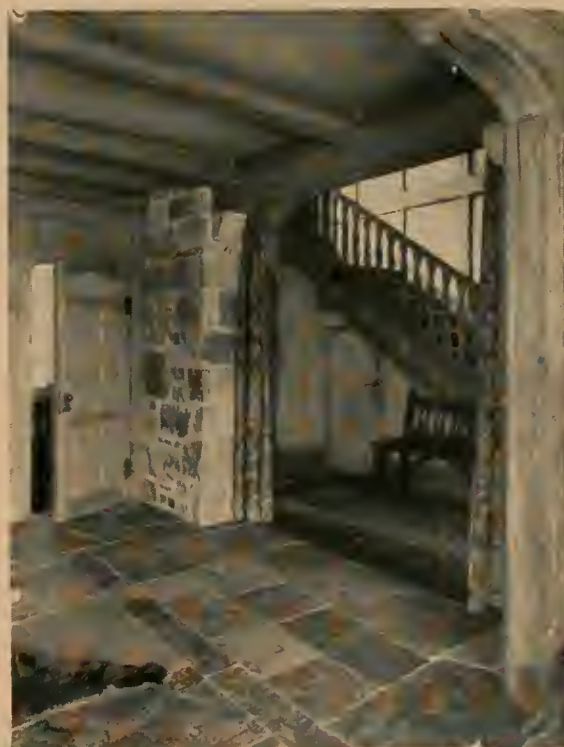
Slate Floor for a Hallway
