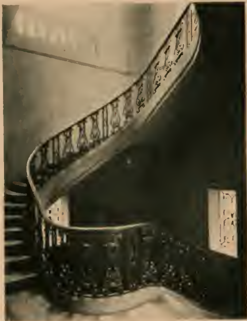
ORNAMENTAL IRON STAIR RAILS PASADENA CITY HALL
