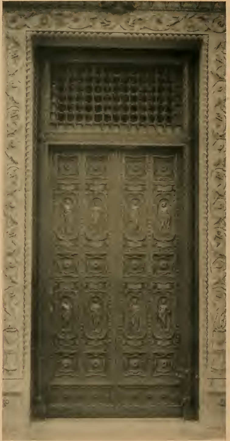
THE BRONZE DOOR WHICH FORMS THE ENTRANCE TO THE HELLMAN BANK, SEVENTH AND SPRING STS., LOS ANGELES
