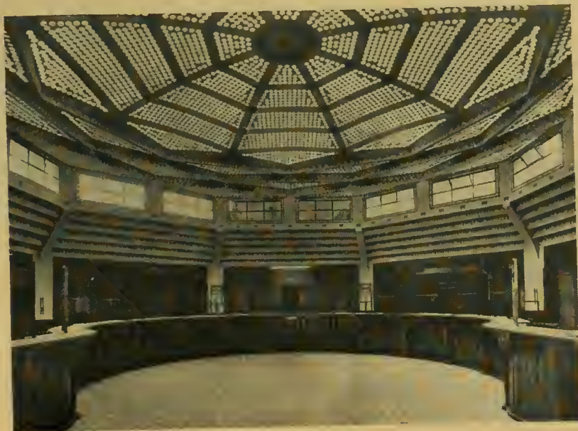
Paris Post-office with glass-stone-ferro-concrete ceiling. Architect F. LeCoeur.
