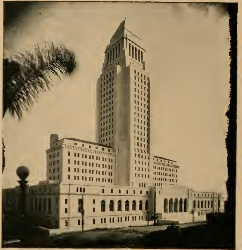
LOS ANGELES CITY HALL, ECONOMICALLY, EFFICIENTLY HEATED BY FOUR No. 5½ JOHNSON ROTARY OIL BURNERS INSTALLED BY ENGLISH & LAUER, OIL BURNER SPECIALISTS
