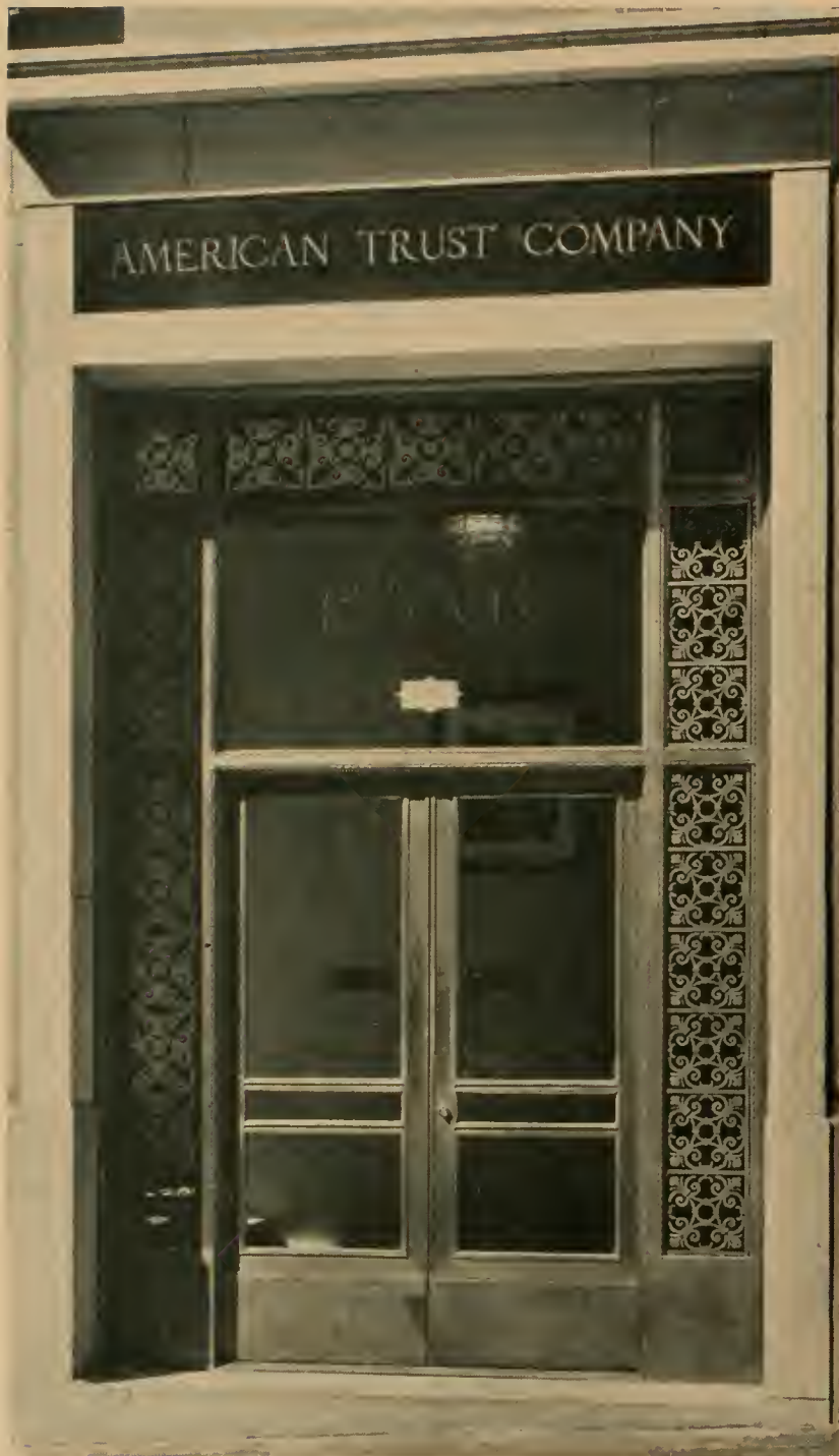
BRONZE ENTRANCE DOORS Palace Hotel Branch, American Trust Company San Francisco
