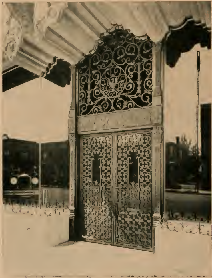
WROUGHT IRON AND CAST IRON ENTRANCE FOR THE HOWARD MOTOR CAR CO., PASADENA, CALIFORNIA
