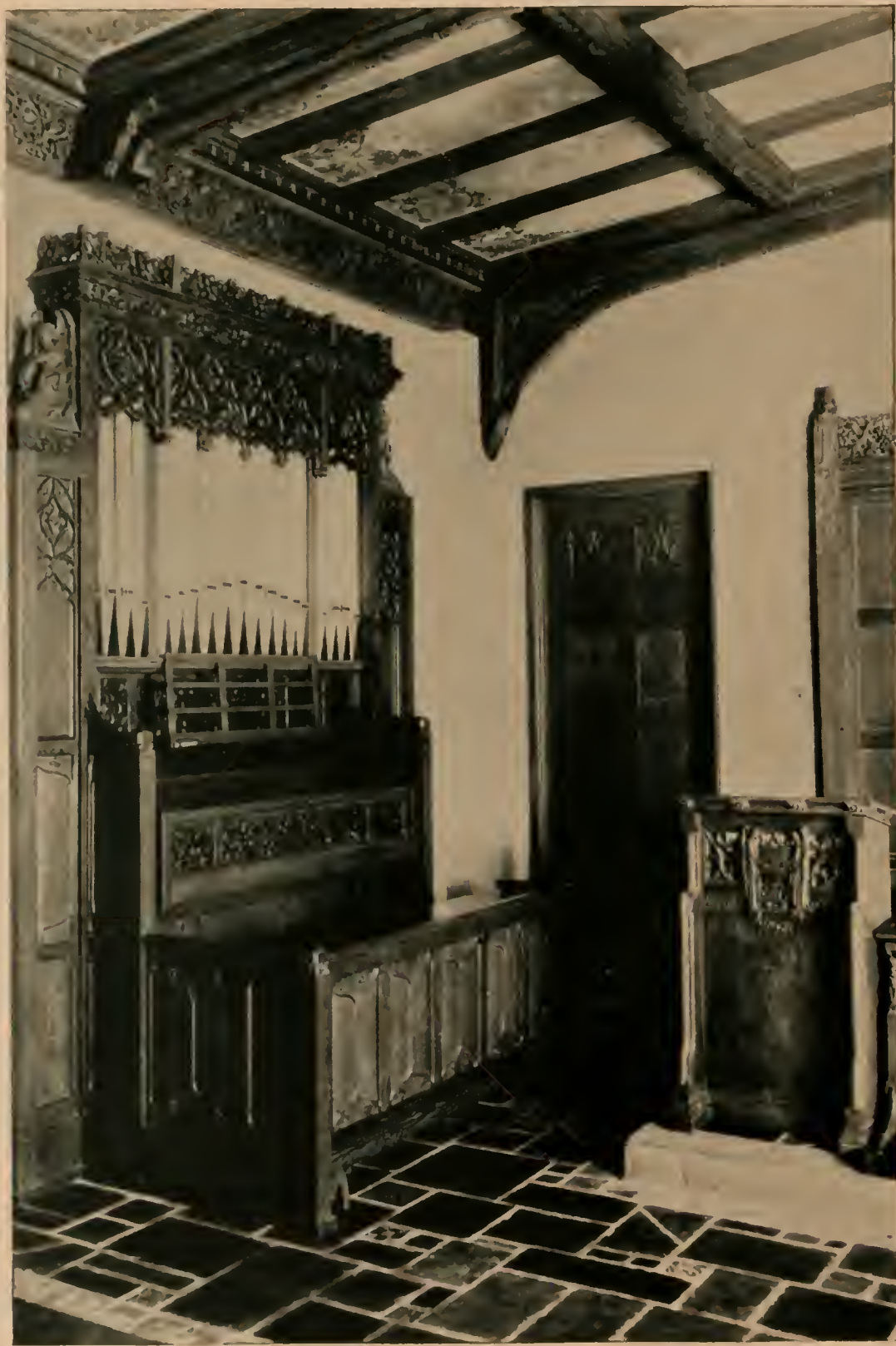
Wesley Chapel Metropolitan M. E. Church Detroit, Michigan W. E. N. HUNTER, ARCHITECT
