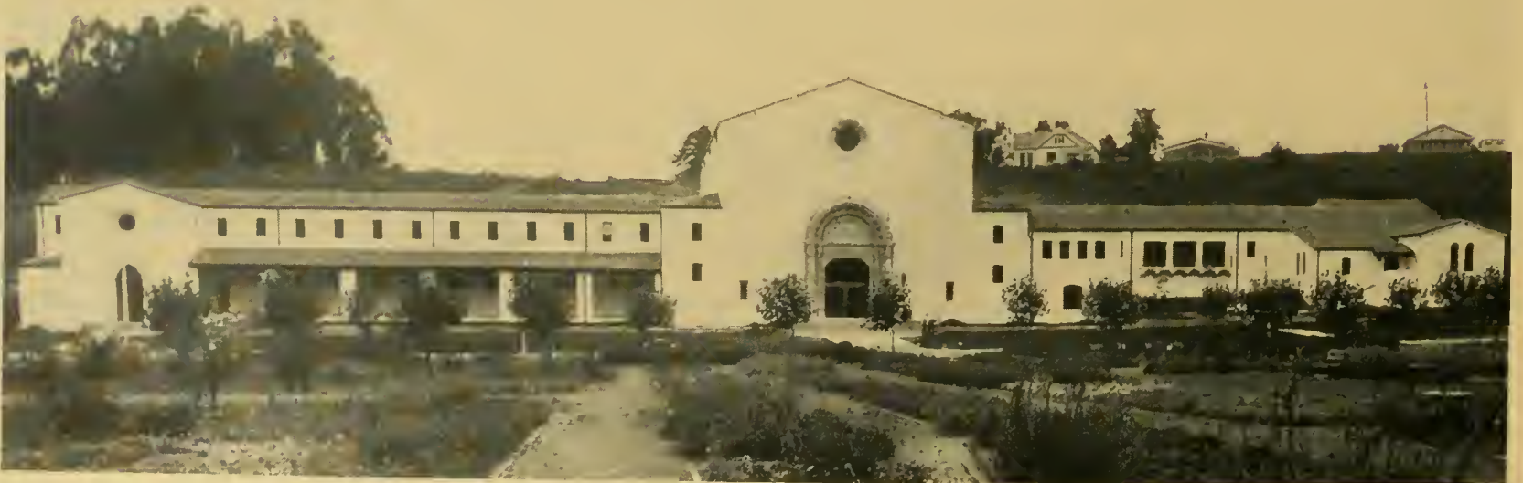
MUSIC BUILDING, MILLS COLLEGE. W. H. RATCLIFF, ARCHITECT
