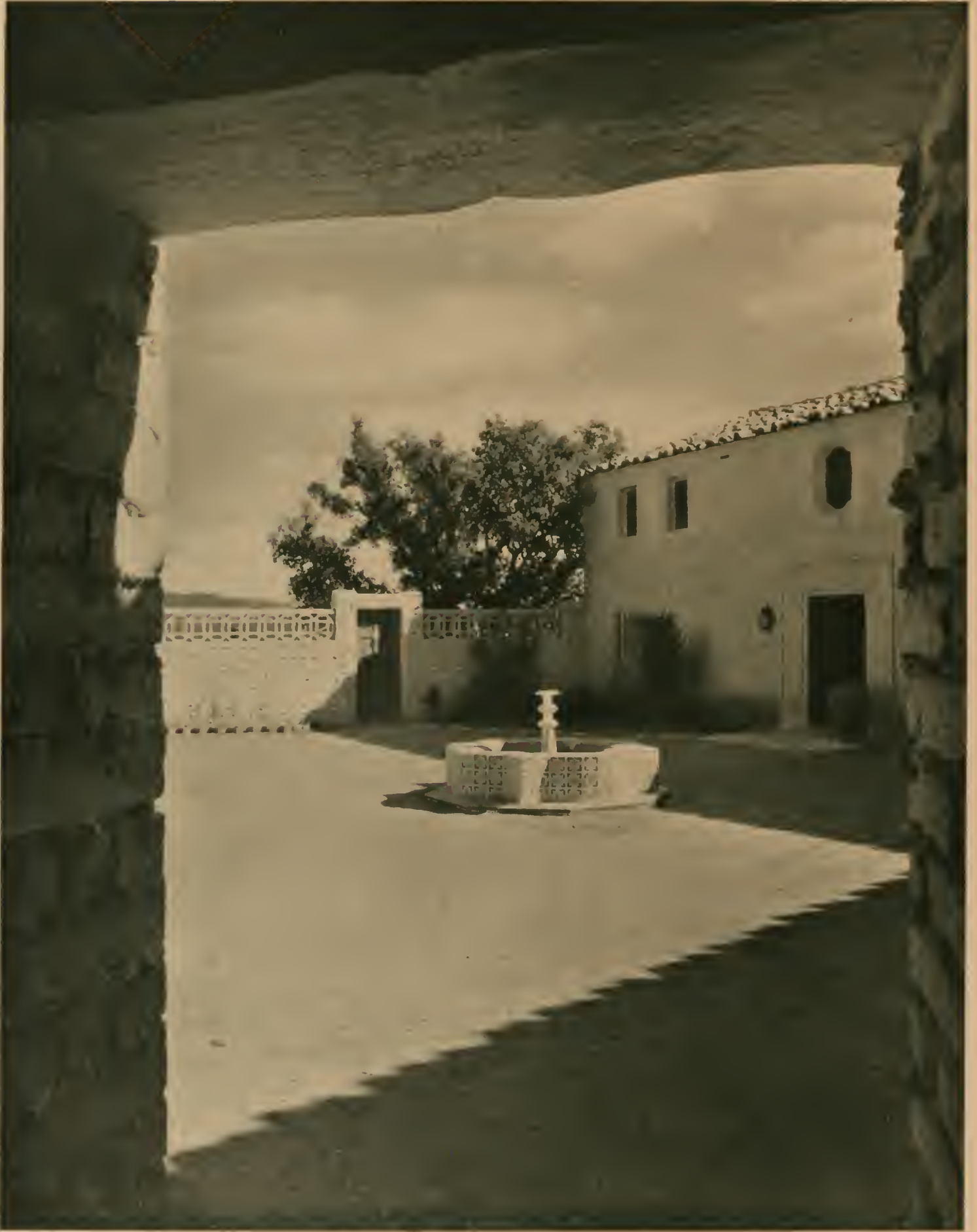
FORECOURT, RESIDENCE OF ALEXANDER CURLETT, ARCHITECT, BEL-AIR, CALIFORNIA
