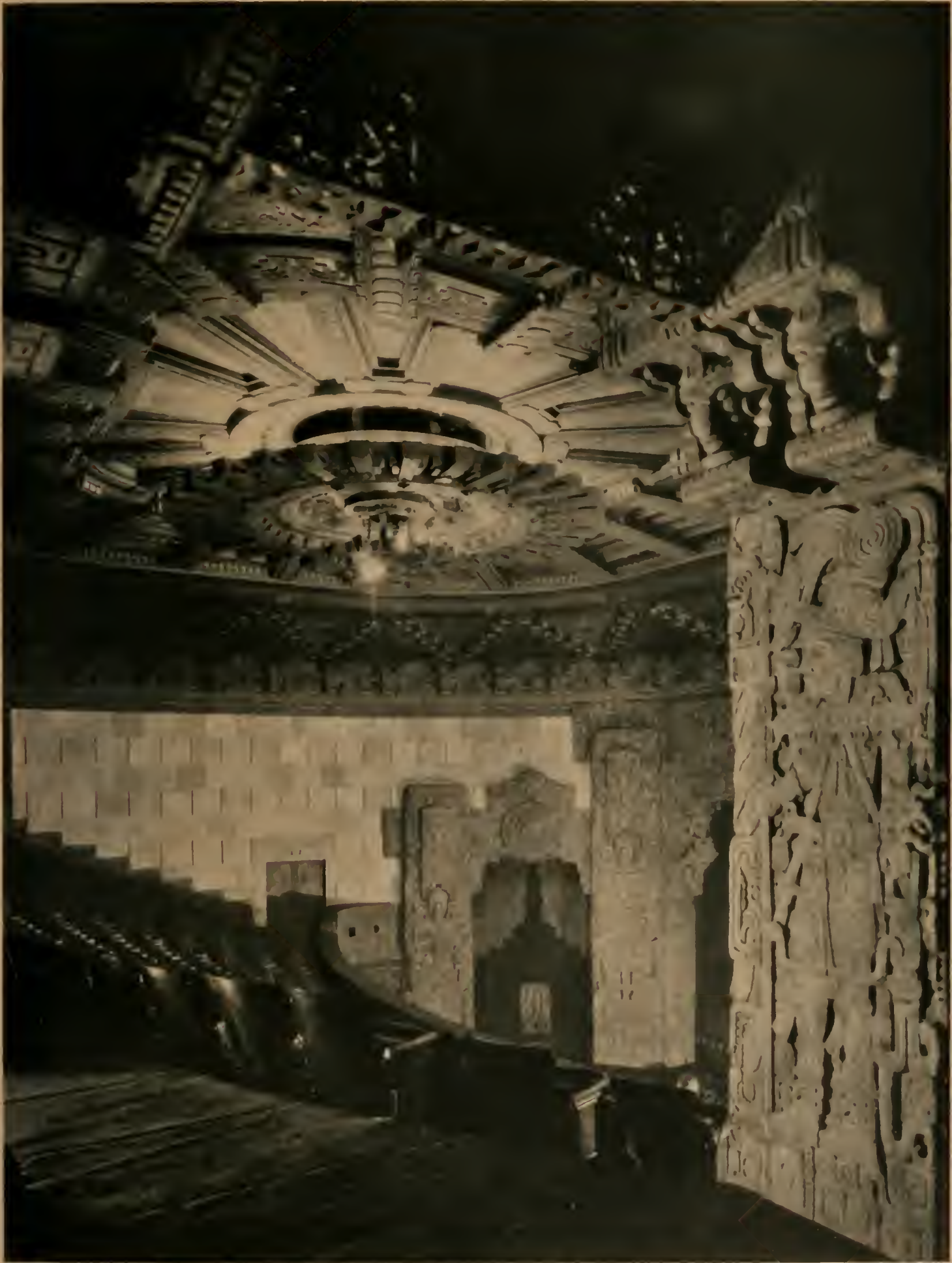
AUDITORIUM CEILING, MAYAN THEATRE, LOS ANGELES, CALIFORNIA MORGAN, WALLS AND CLEMENTS, ARCHITECTS
