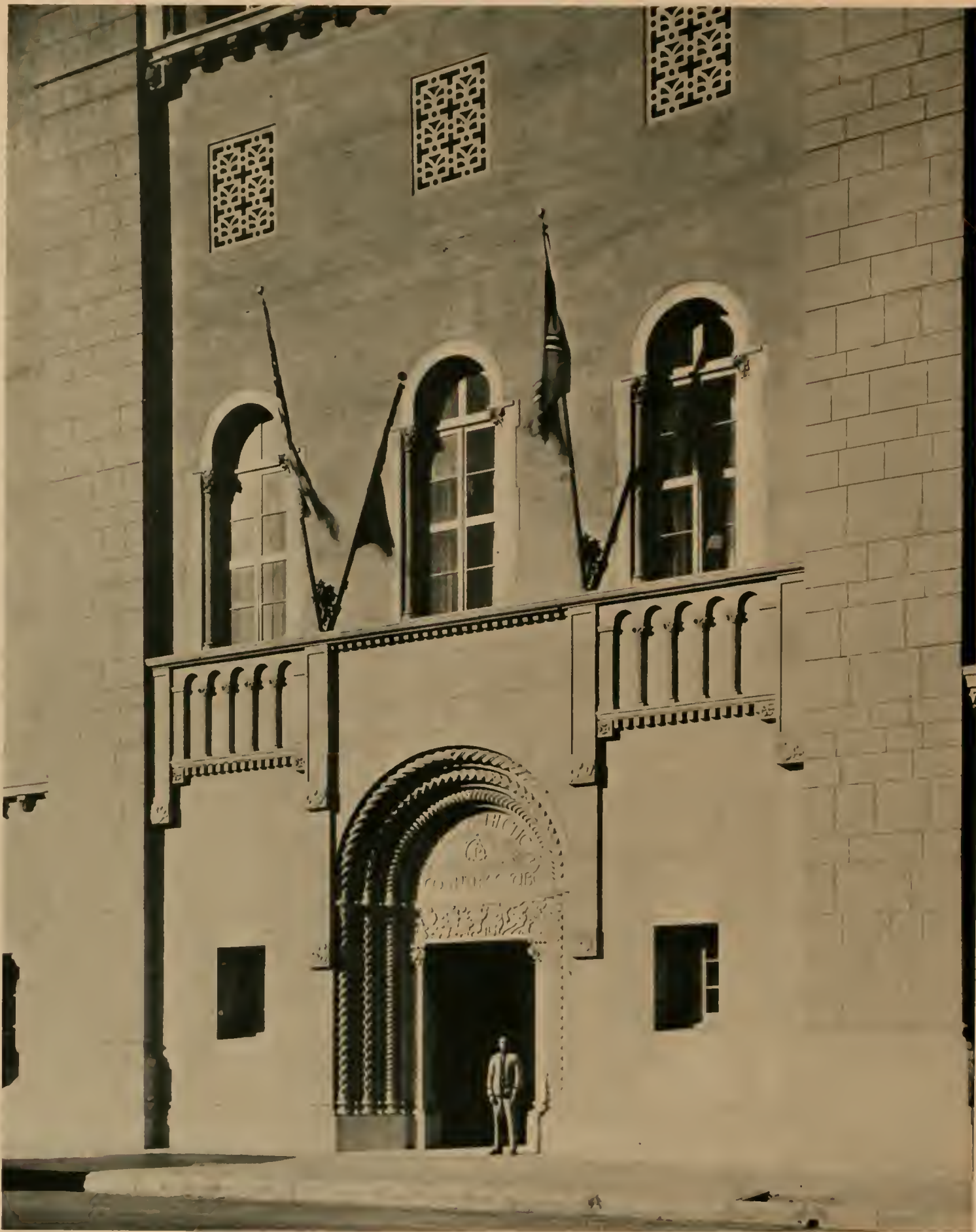
ENTRANCE DETAIL, PASADENA ATHLETIC AND COUNTRY CLUB, PASADENA, CALIFORNIA MARSTON, VAN PELT AND MAYBURY, ARCHITECTS
