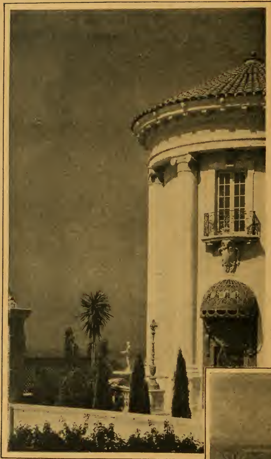
Kenneth MacDonald, Jr., Architect, Los Angeles H. W. Baum Co., General Contractors, Los Angeles
