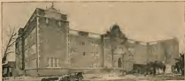
La Fayette School, New Orleans, La. E. A. Christy, Architect
