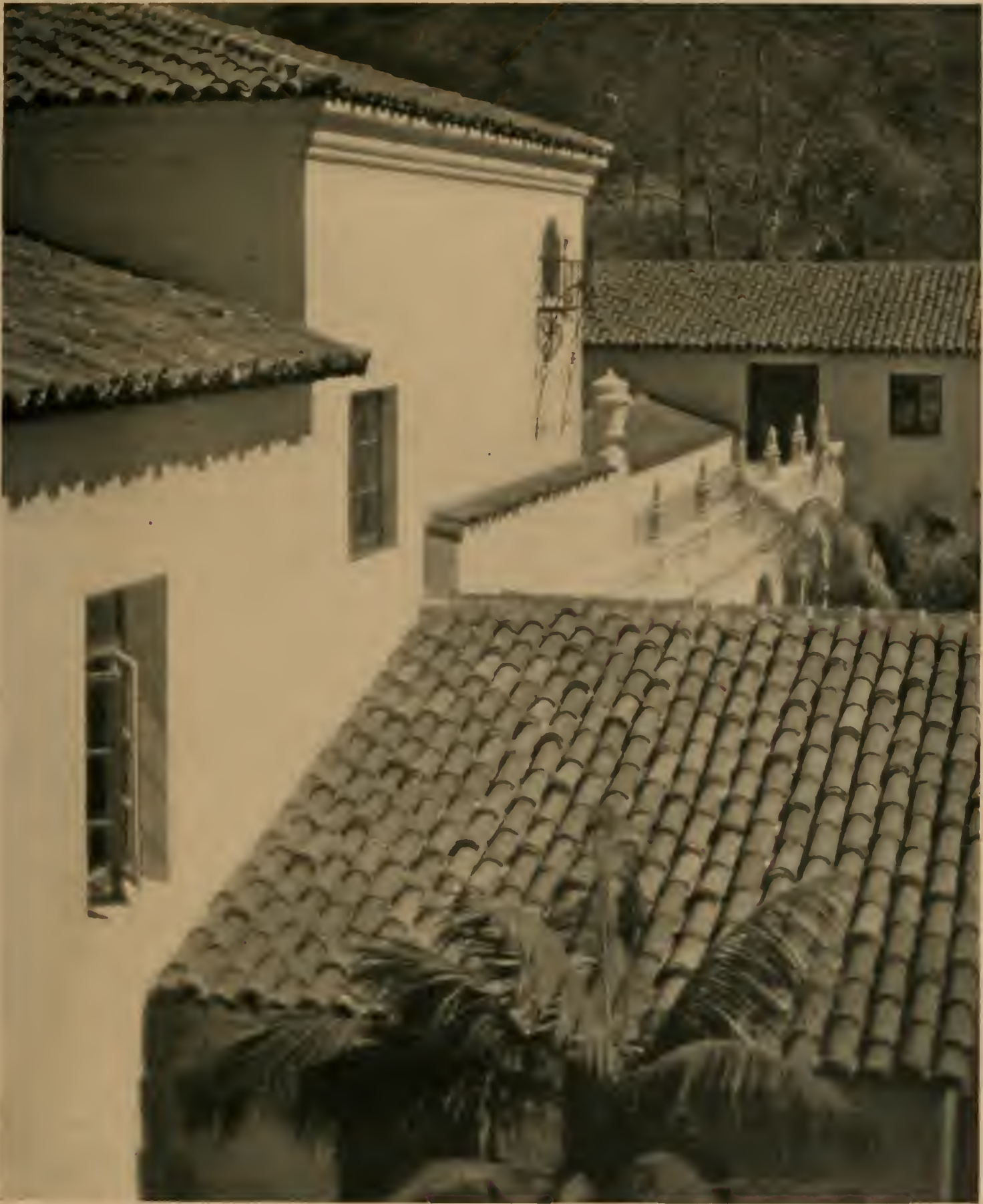
PATIO ROOFS, ADMINISTRATION BUILDING, BEL-AIR, CALIFORNIA. DESIGNED BY MARK DANIELS
