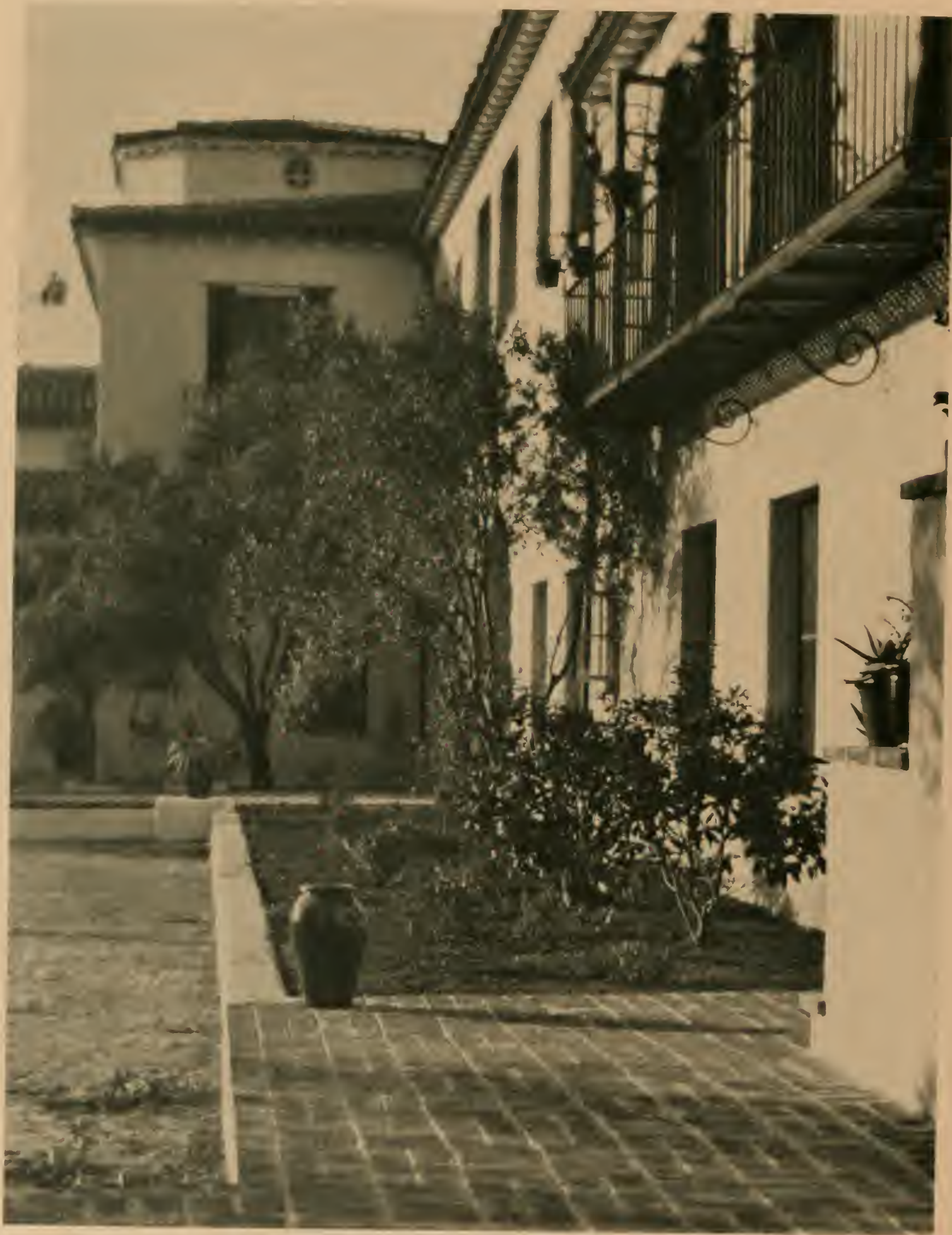
DETAIL, MAIN FACADE, THE BILTMORE, SANTA BARBARA, CALIFORNIA REGINALD D. JOHNSON, ARCHITECT
