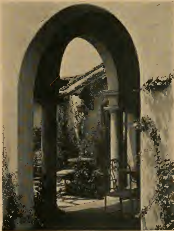
Residence, Mrs. M. Martindale, Pasadena, California J. J. Kucera, Architect
