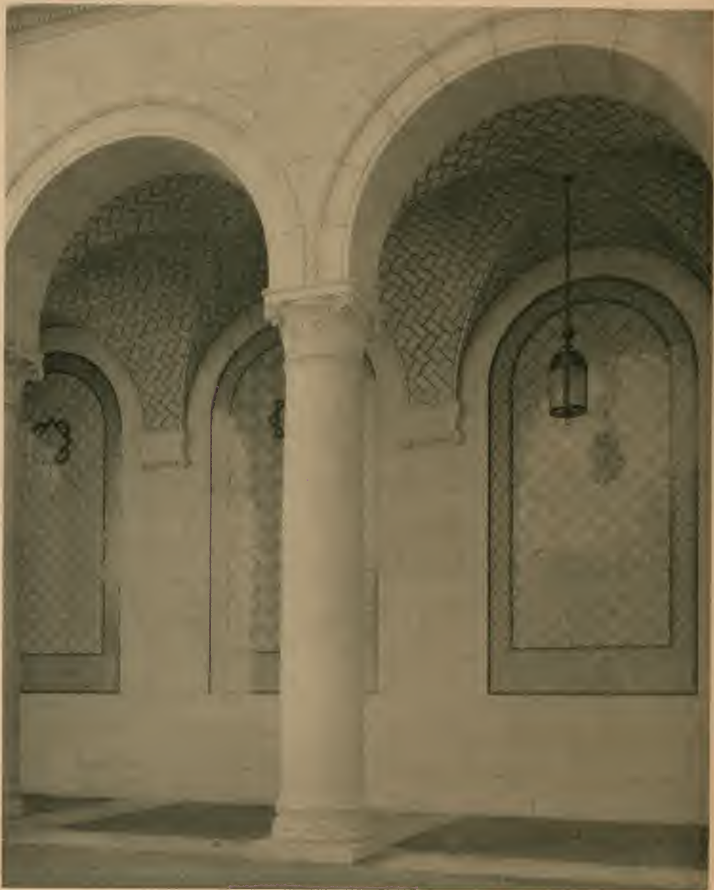
Arcade in Forecourt, Los Angeles City Hall
