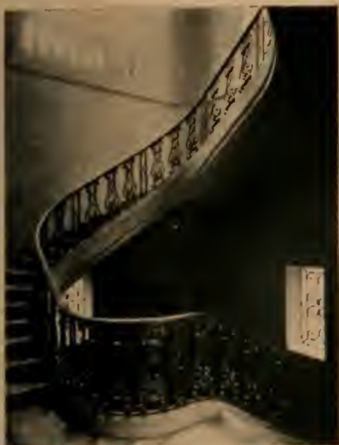
ORNAMENTAL IRON STAIR RAILS PASADENA CITY HALL
