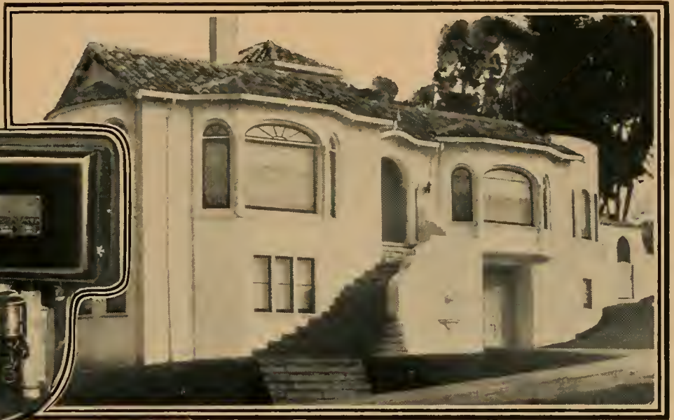
Installed in the Wilms Home, Monterey Heights, San Francisco
