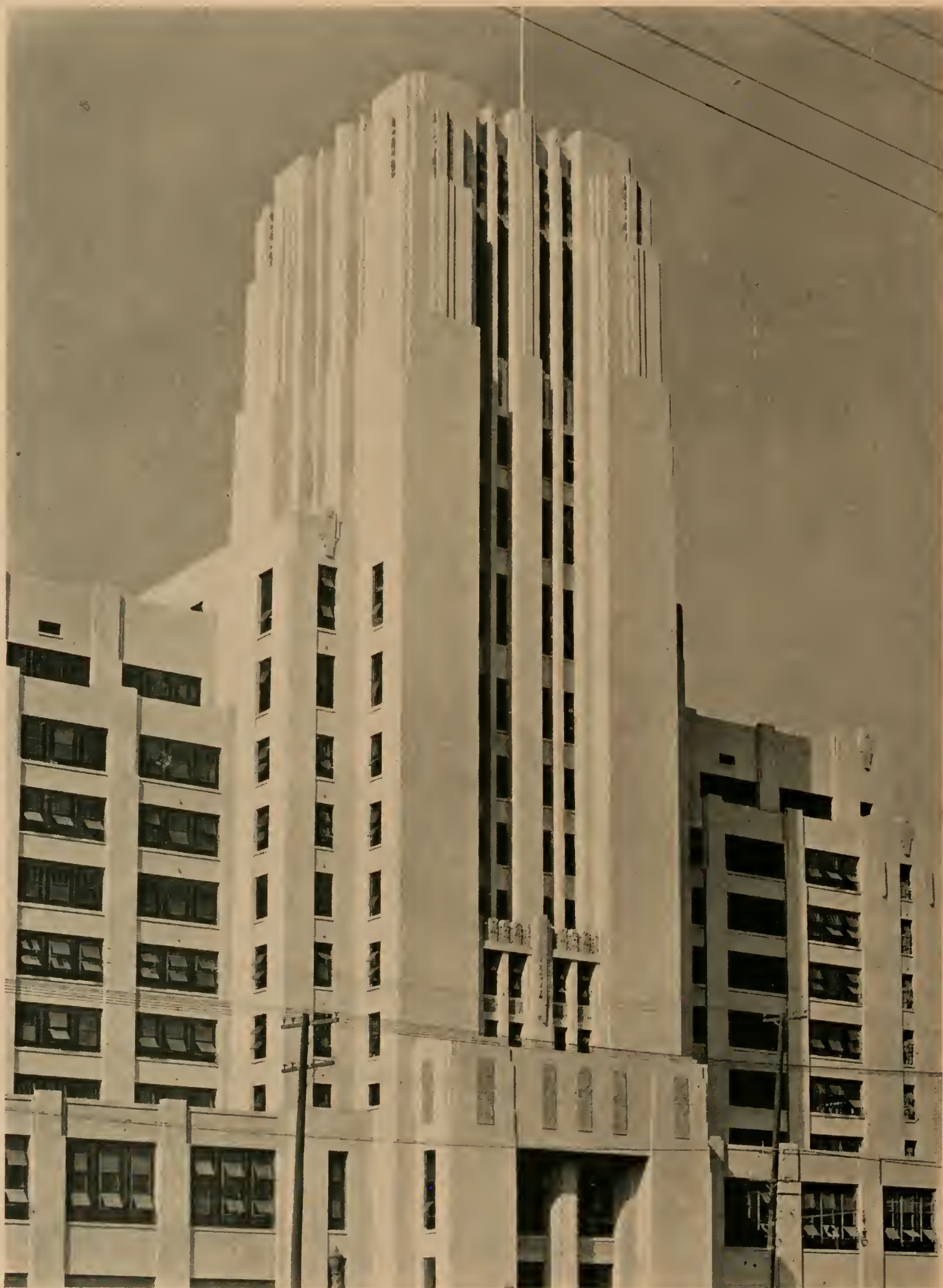
TOWER DETAIL, SEARS, ROEBUCK & CO. BUILDING, LOS ANGELES, CALIFORNIA GEO. C. NIMMONS & CO., ARCHITECTS
