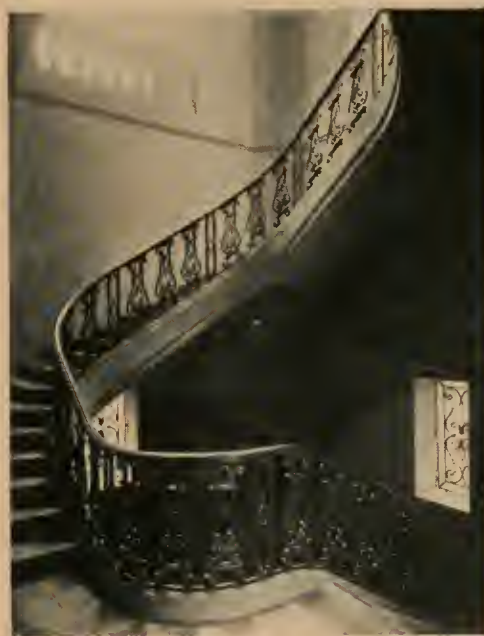
ORNAMENTAL IRON STAIR RAILS PASADENA CITY HALL
