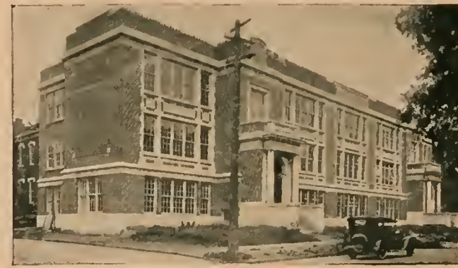
High School, Greenville, S. C. J. E. Serrine & Co., Architects
