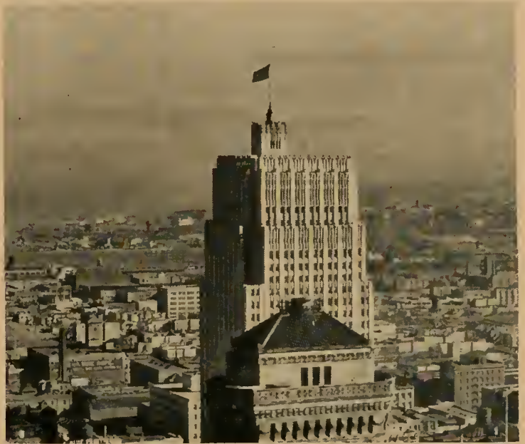
A steel flag pole arises from the top of the Pacific Telephone and Telegraph Building, San Francisco. Miller and Pflueger, Architects
