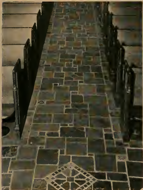
Slate Floor of a Church
