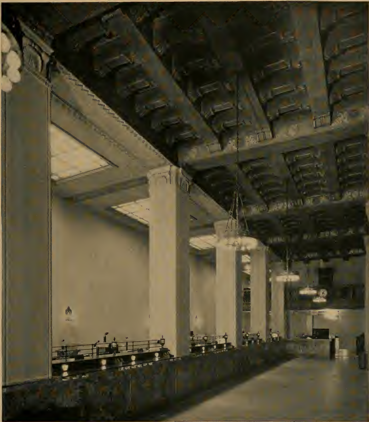
Walker & Eisen, Architects
