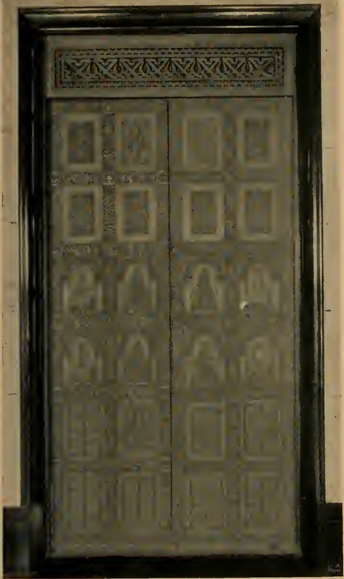
CAST BRONZE ELEVATOR DOORS John D. Spreckels Building, San Diego, Calif. John Parkinson and Donald B. Parkinson, Architects
