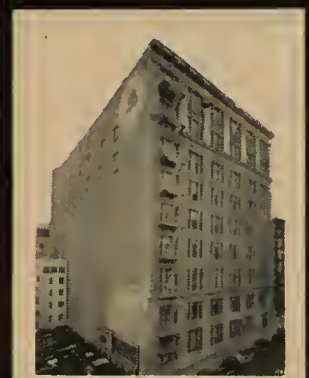
So. Cal. Telephone Co.
