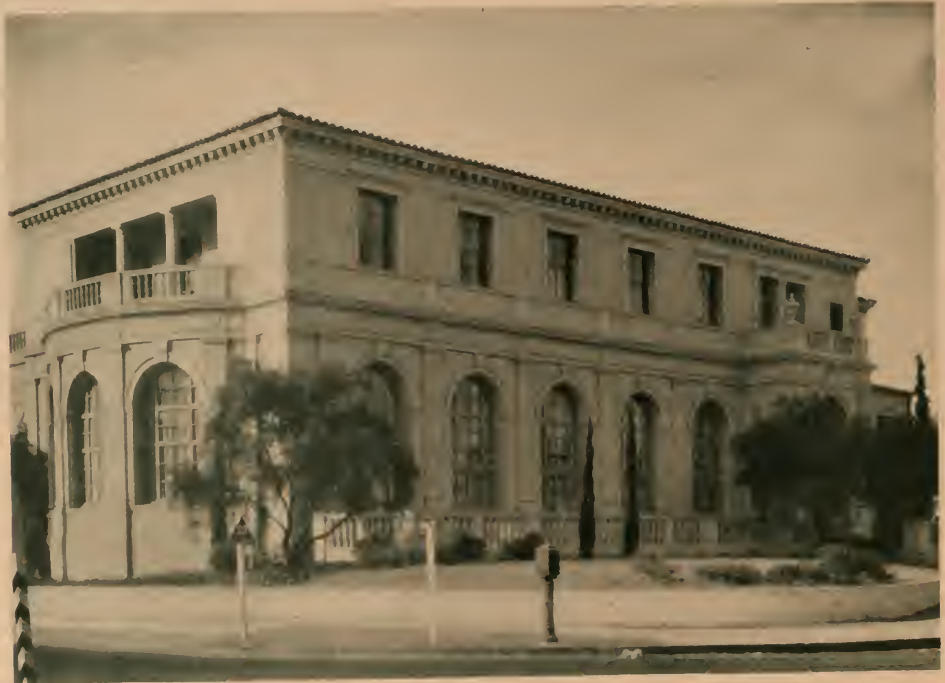
ABOVE—THEATER WING; BELOW—CLUB WING; EBELL CLUB, LOS ANGELES, CALIFORNIA HUNT AND BURNS, ARCHITECTS
