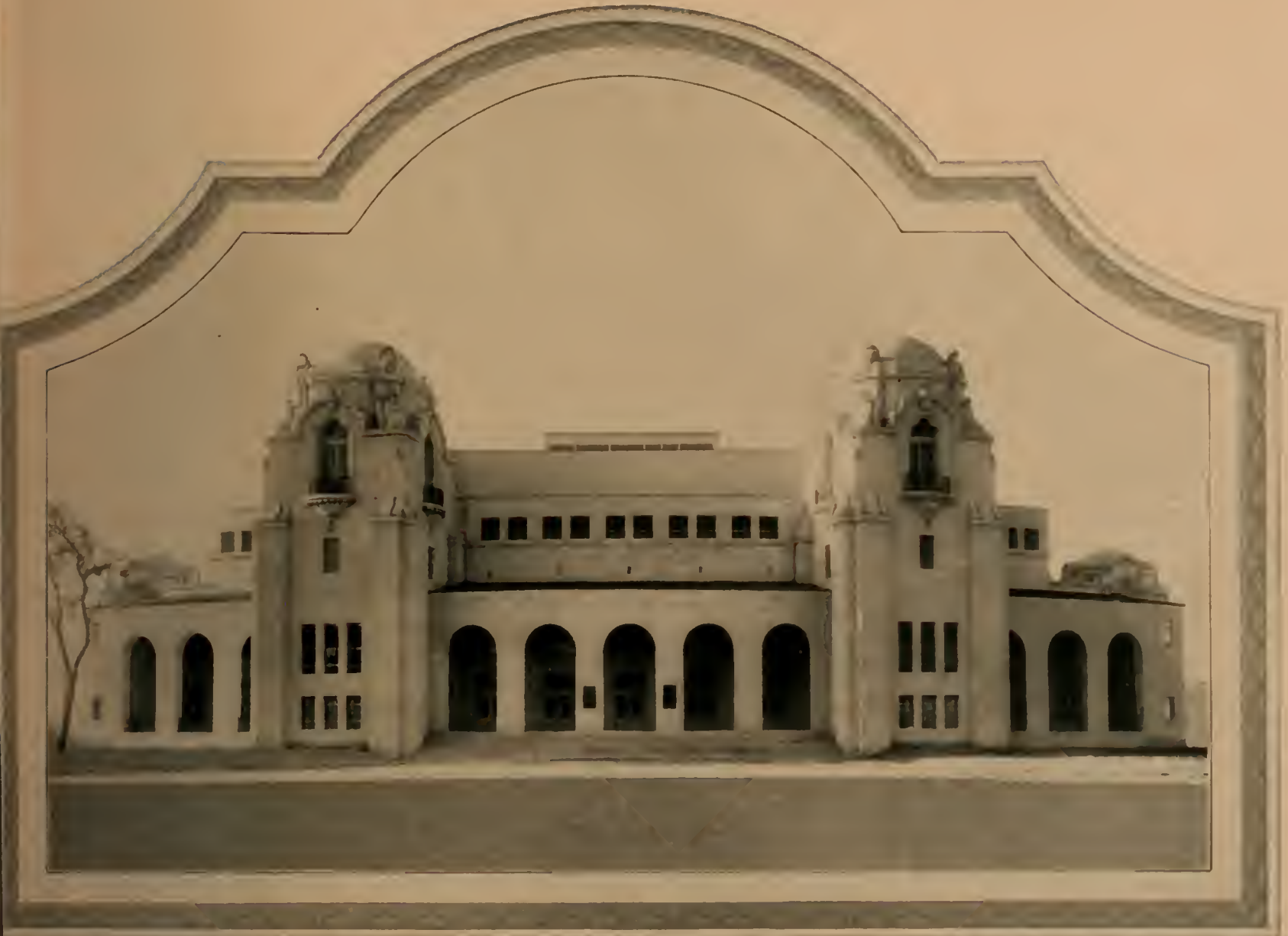
IR PARK AUDITORIUM, DALLAS, TEXAS . . . . LANG & WITCHELL, ARCHITECTS . . . . EQUIPPED WITH JOHNSON HEAT CONTROL
