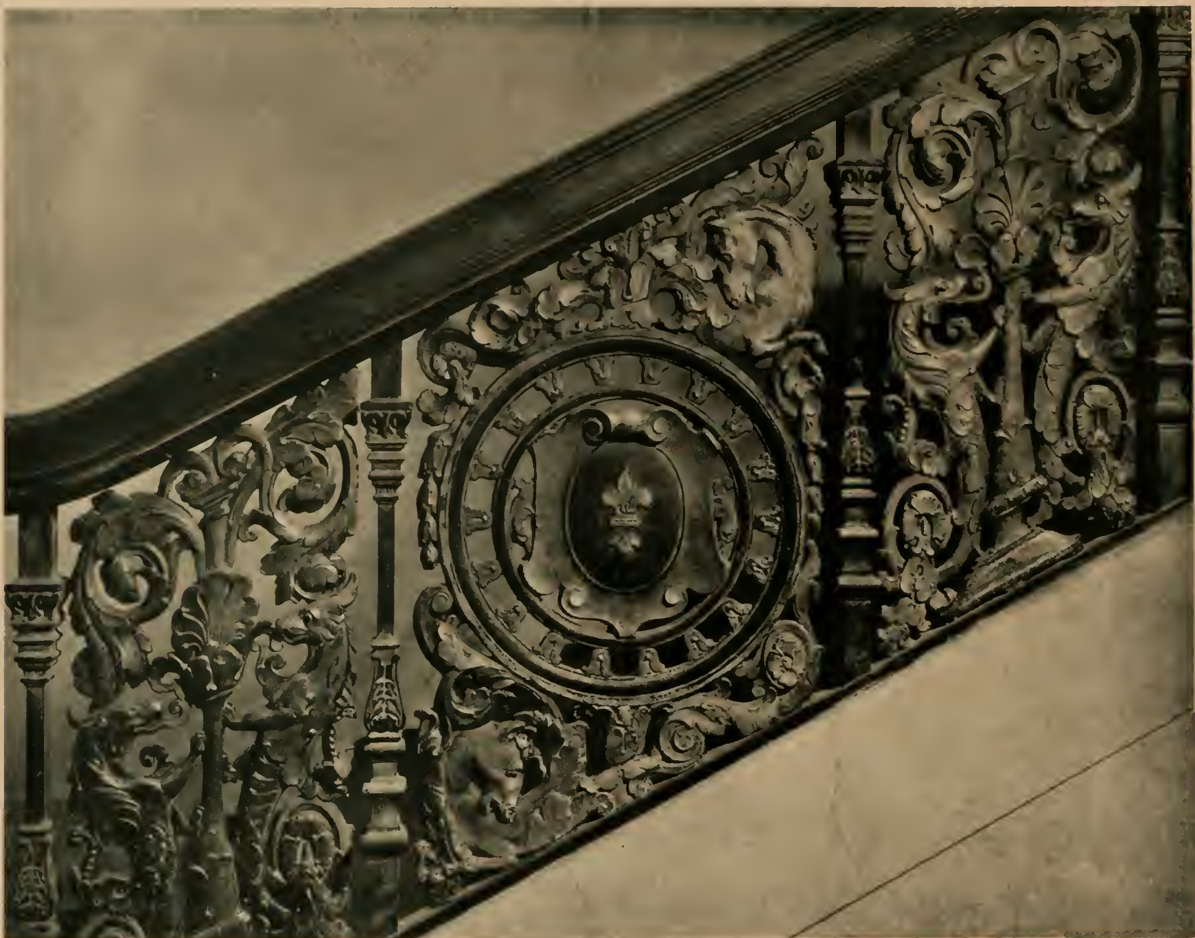
CAST IRON STAIR RAILING, HOTEL MARK HOPKINS
