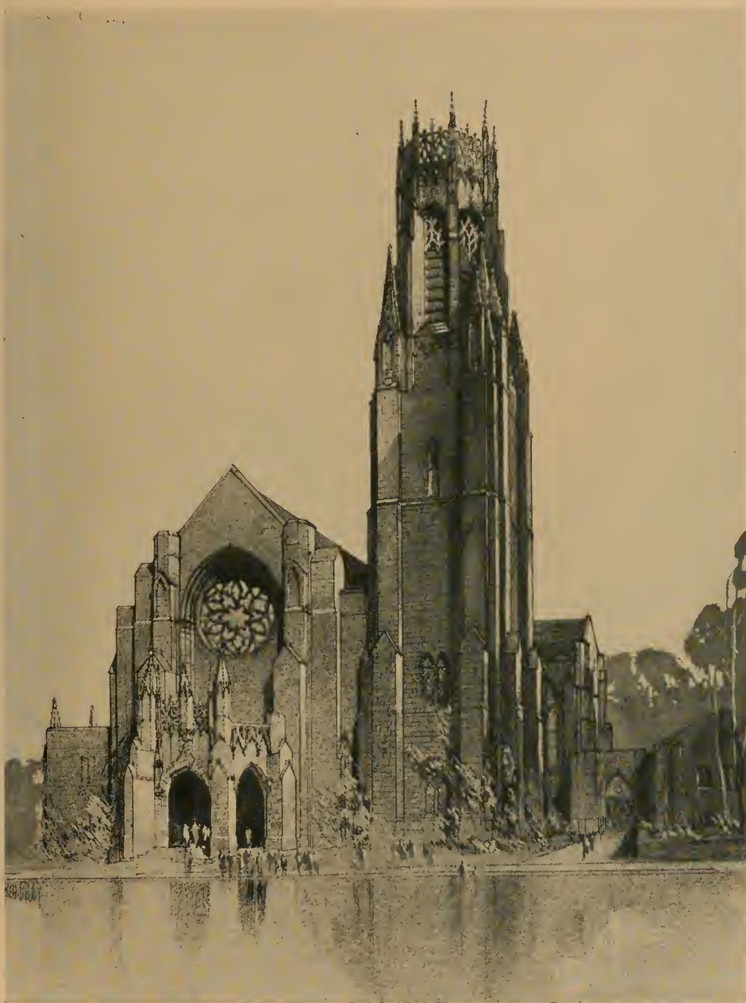
WESTMINSTER PRESBYTERIAN CHURCH, PASADENA, CALIFORNIA. MARSTON, VAN PELT AND MAYBURY, ARCHITECTS.
