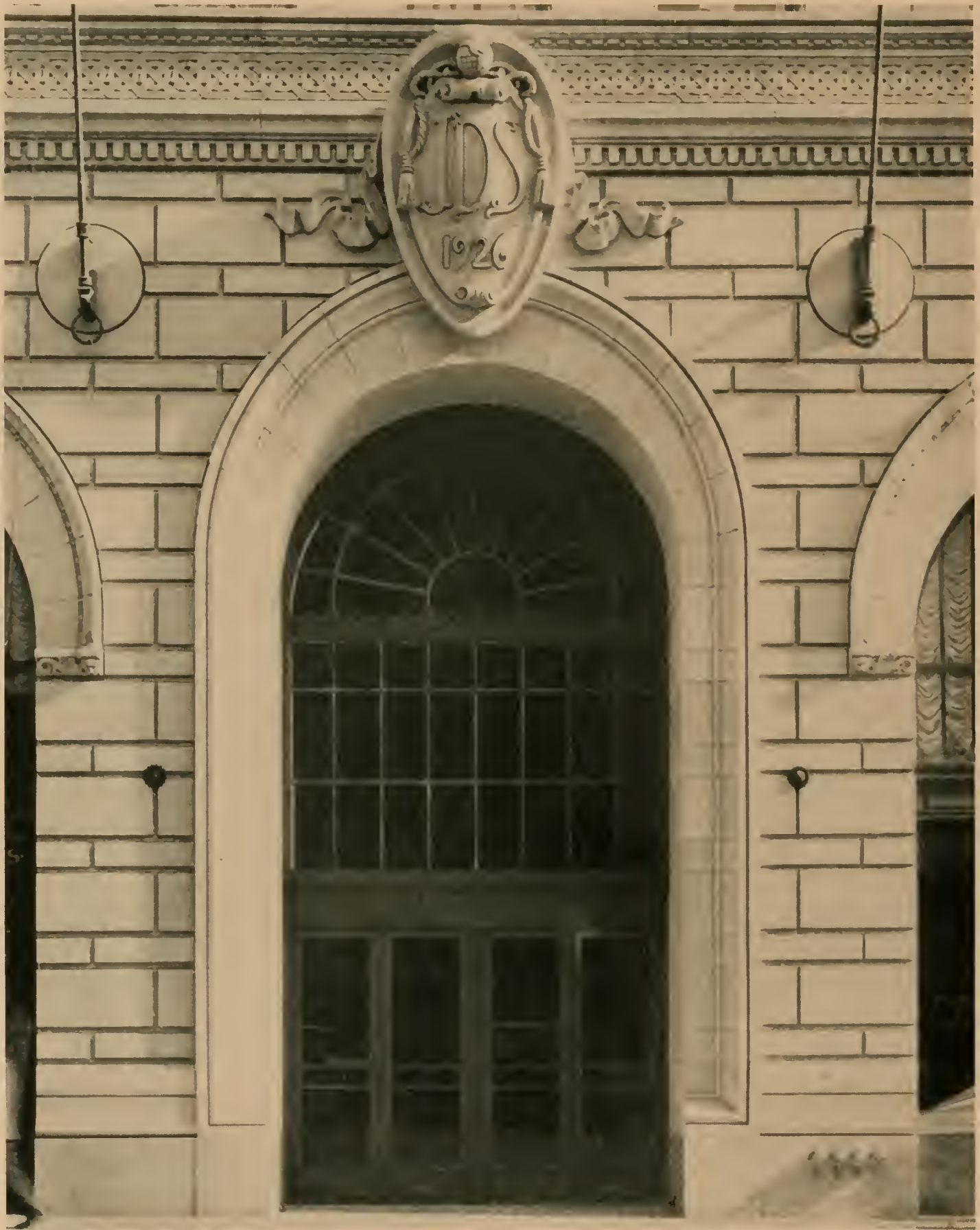
Entrance Detail, John D. Spreckels Building, San Diego.
