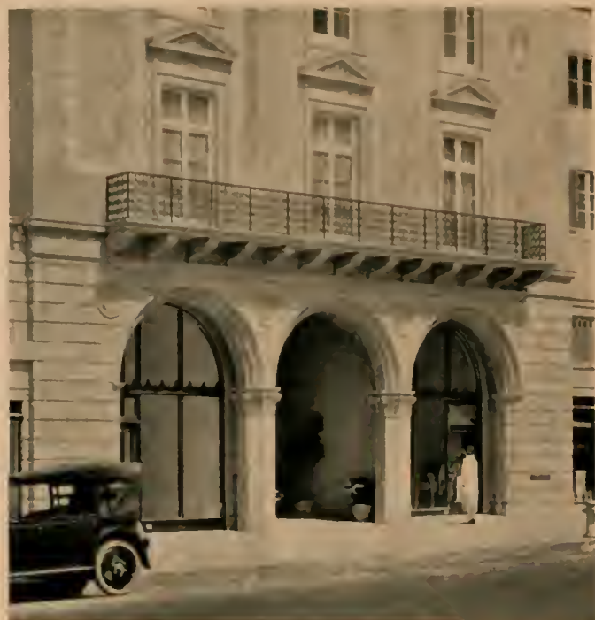
Balcony Railing Women's Athletic Club, Los Angeles Allison & Allison, Architects
