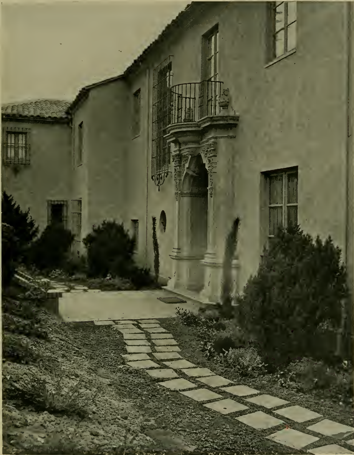
RESIDENCE OF MRS. J. H. BALSDON, CLAREMONT, CALIFORNIA. CLARENCE A. TANTAU, ARCHITECT
