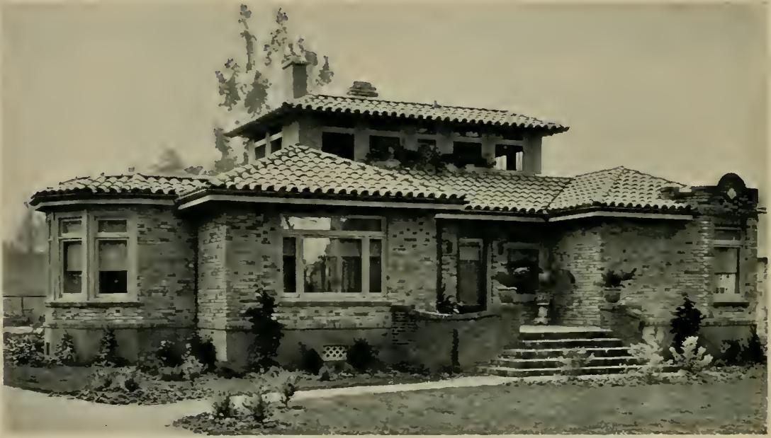
BURLINGAME RESIDENCE OF CHARLES HOCK OF HOCK & HOFFMEYER DICKEY FACE BRICK BACKED WITH DICKEY MASTERTILE
