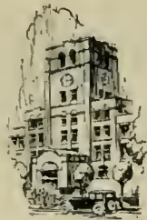
Bell Tower Kohler Administration Building
