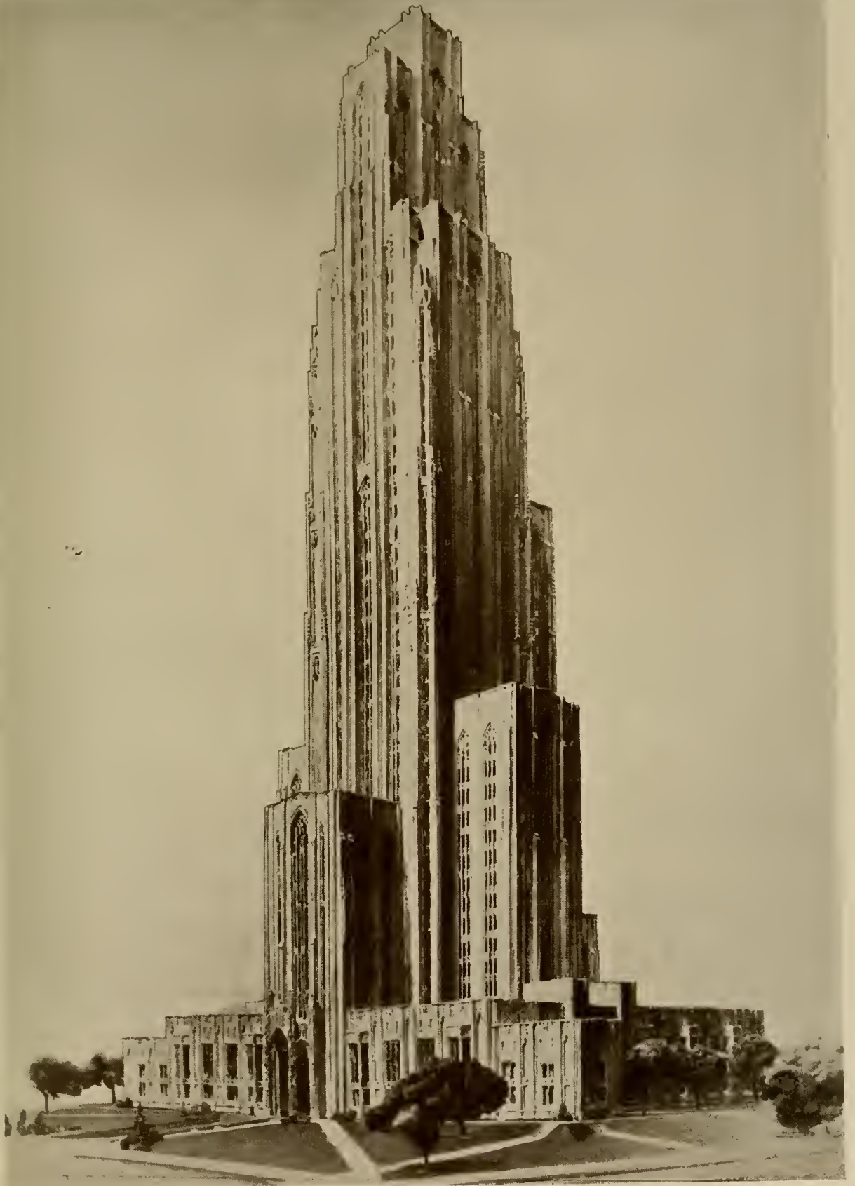
THE "CATHEDRAL OF LEARNING," UNIVERSITY OF PITTSBURGH, PENNSYLVANIA. CHARLES Z. KLAUDER, ARCHITECT
