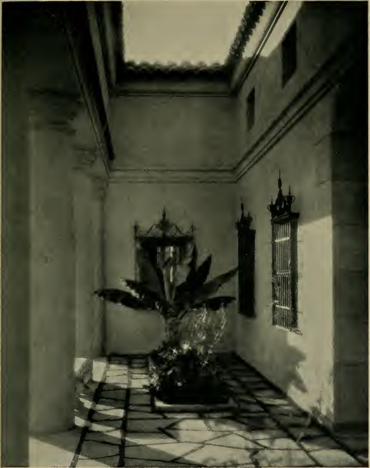
ENTRANCE LOGGIA, AUTO SALES BUILDING FOR STANLEY W. SMITH, INC., HOLLYWOOD, CALIFORNIA MCNEAL SWASEY, ARCHITECT
