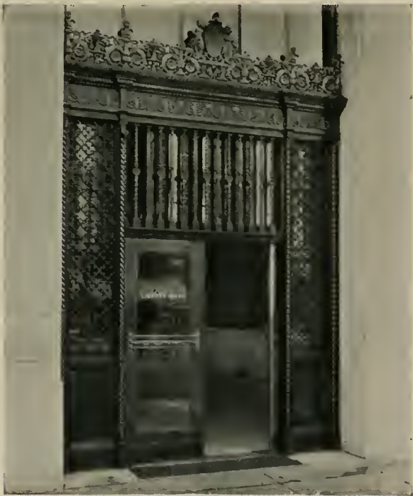
Liberty Bank Building, San Francisco. H. A. Minton, Architect Ornamental Iron Entrance and Bronze Teller Cages Show True Craftsmanship.
