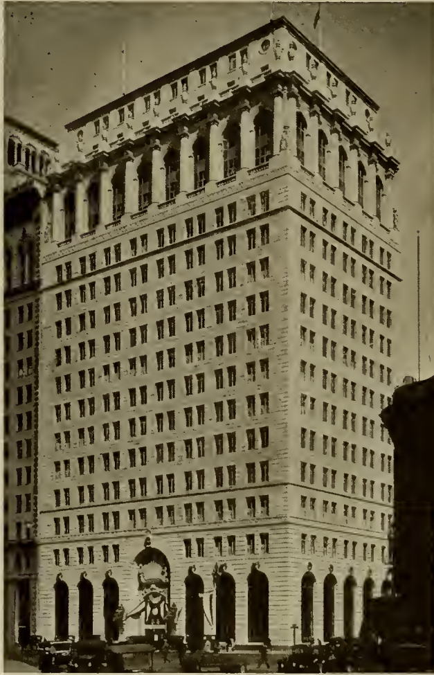
PACIFIC GAS AND ELECTRIC BUILDING, SAN FRANCISCO BAKEWELL & BROWN, ARCHITECTS
