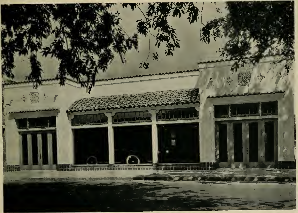
ABOVE—ORMSBY CHEVROLET COMPANY, SAN ANTONIO, TEXAS; BELOW—AUTOMOBILE SHOWROOM OF JACK W. NEAL SAN ANTONIO, TEXAS. ATLEE B. AND ROBERT M. AYRES, ARCHITECTS
