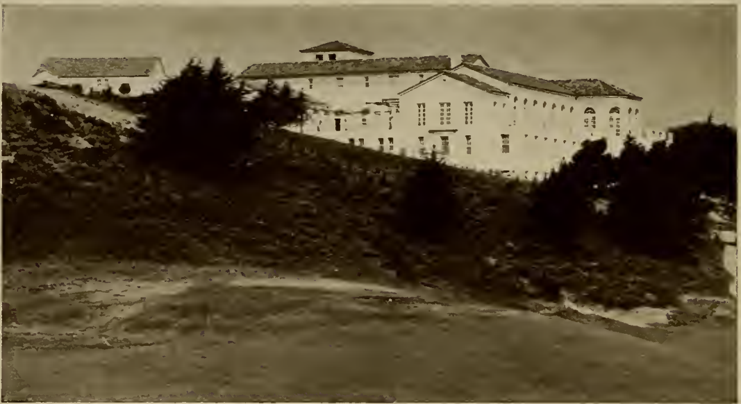
New Club House, Olympic Golf and Country Club, Lakeside Associate Architects, Bakewell & Brown, and John A. Bauer, San Francisco General Contractors, K. E. Parker Co., San Francisco Painting and Decorating, William Nielson, San Francisco
