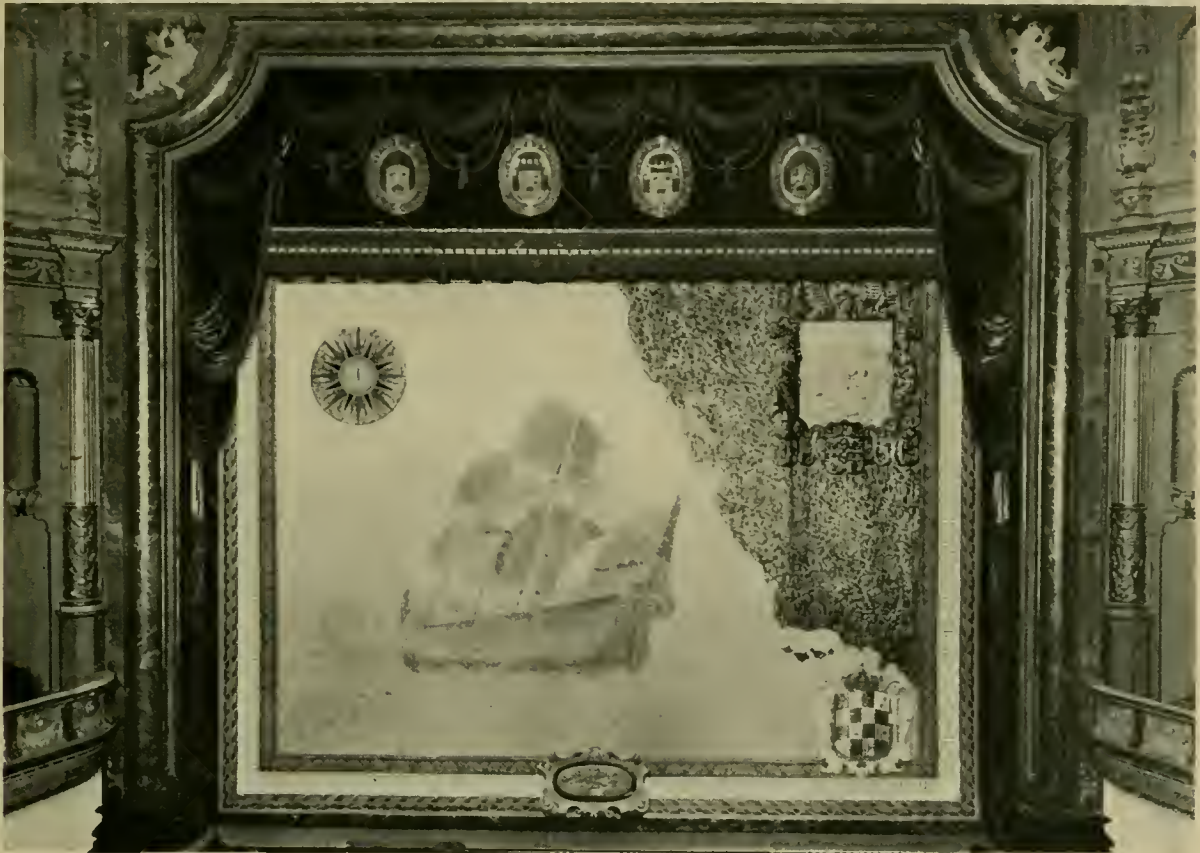
PROSCENIUM ARCH, BILTMORE THEATRE. SCHULTZE & WEAVER, ARCHITECTS
