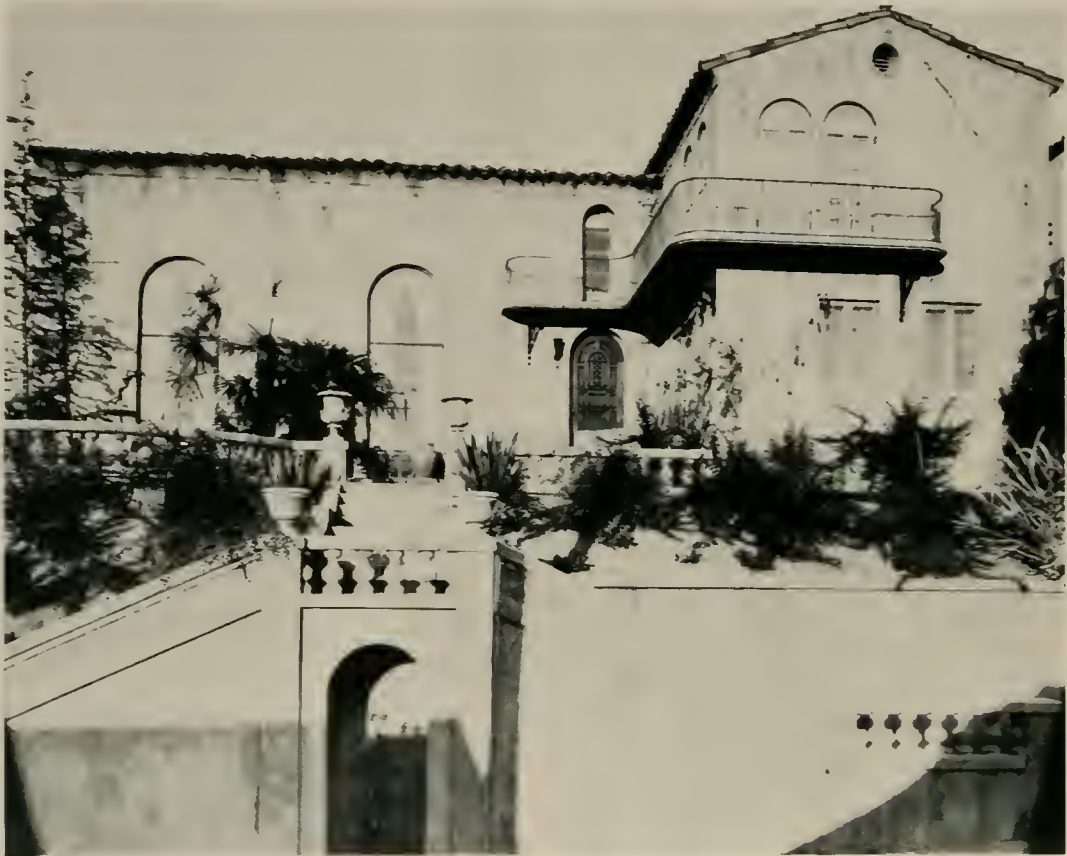
ITALIAN HILLSIDE HOME, PATTERNED AFTER A RARE OLD RESIDENCE IN SOUTHERN ITALY. BUILT IN HOLLYWOOD AND FINISHED WITH CALIFORNIA STUCCO TO SIMULATE THE ORIGINAL
