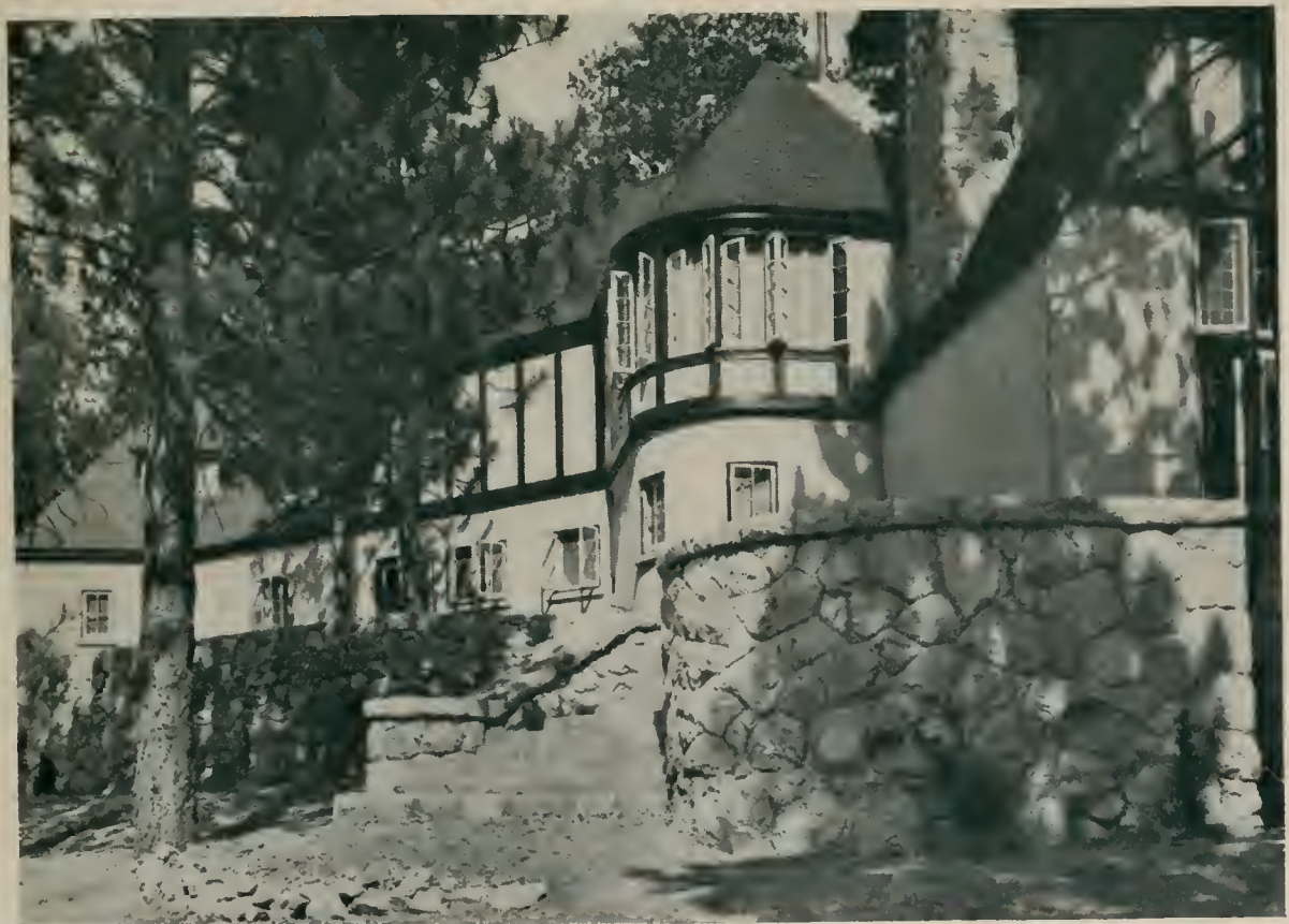
ABOVE—VAN NUYS RESIDENCE; BELOW—MODINI-WOODS RESIDENCE, LAKE ARROWHEAD, CALIFORNIA MCNEAL SWASEY, ARCHITECT, H. C. MCAFEE, ASSOCIATE
