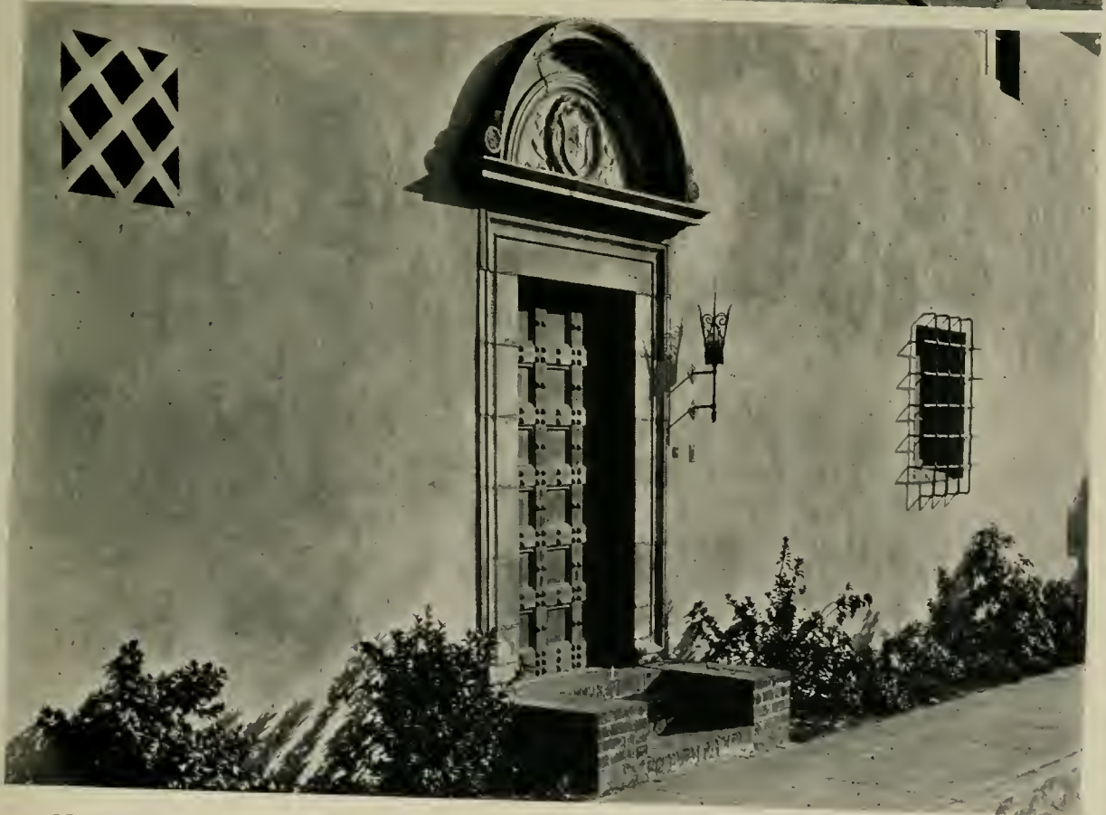
RESIDENCE OF MR. F.W. CONANT, HOLLYWOOD, CALIFORNIA. PIERPONT AND WALTER S. DAVIS, ARCHITECTS
