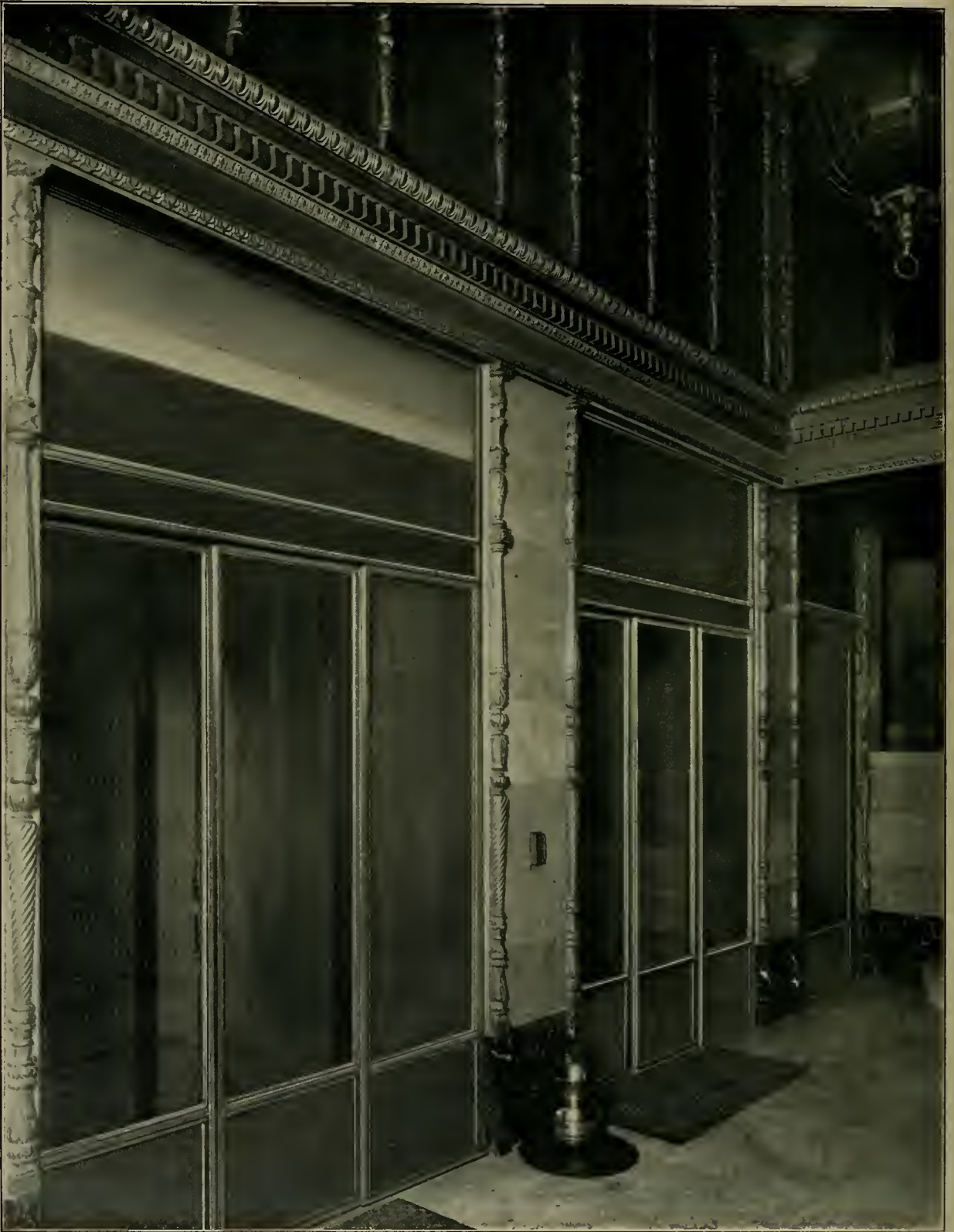
ELEVATOR FRONTS IN LOBBY
