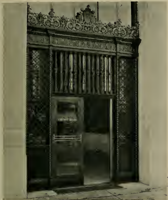
Liberty Bank Building, San Francisco. H. A. Minton, Architect Ornamental Iron Entrance and Bronze Teller Cages Show True Craftsmanship.
