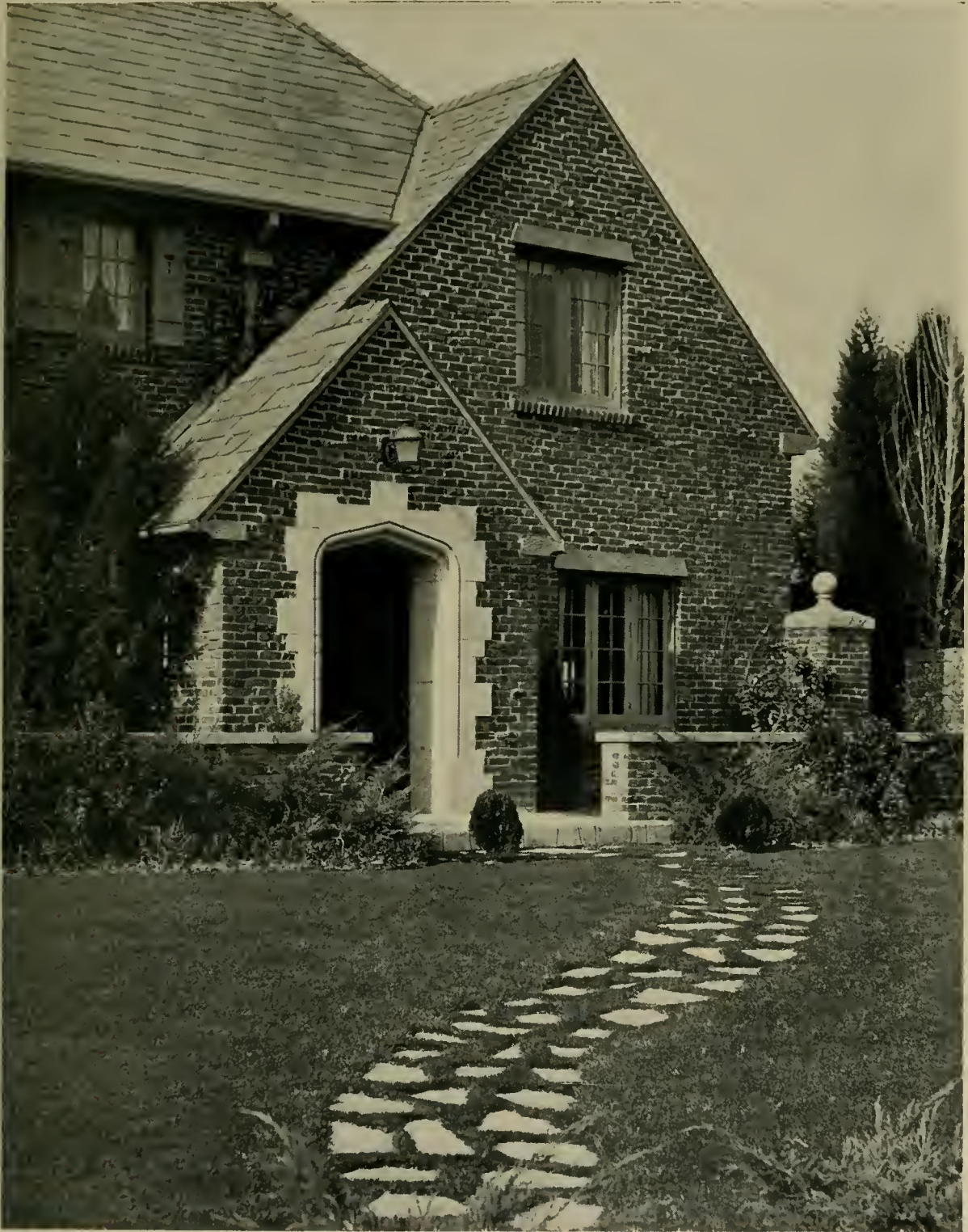
ENTRANCE, RESIDENCE OF MR. C. H. STONE, LOS ANGELES, CALIFORNIA. STILES O. CLEMENTS, ARCHITECT
