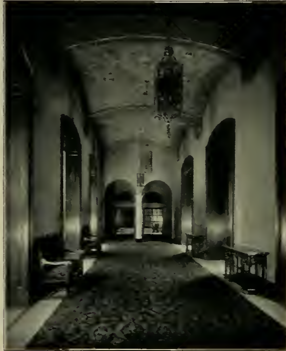
Interior View, Elks Club, San Francisco Architects, Meyer & Johnson, San Francisco General Contractors, R. McLeran & Co., San Francisco Painters, Heinsbergen Decorating Co., San Francisco and Los Angeles
