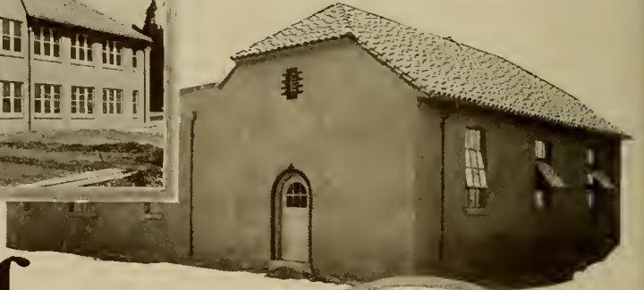
STATE HOSPITAL NORWALK, CAL. ROOFED WITH SIMONS SPANISH TILE
