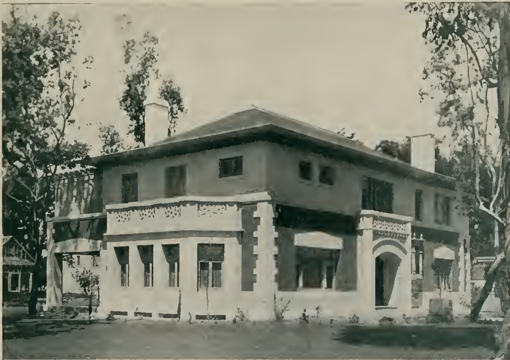
EXTERIORS THE DOHRMAN HOME, STOCKTON, CALIFORNIA, GLENN ALLEN, STOCKTON, ARCHITECT
