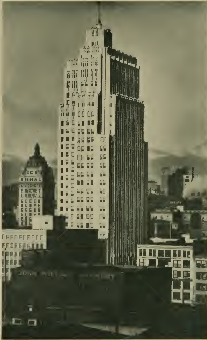
PACIFIC TELEPHONE AND TELEGRAPH CO. BUILDING · SAN FRANCISCO Miller & Pflueger and A. A. Cantin, Assoc. Architects · A. Quandt & Sons, Painters
