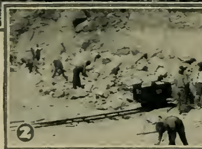
2. Result of first big shot of dynamite at quarry.
