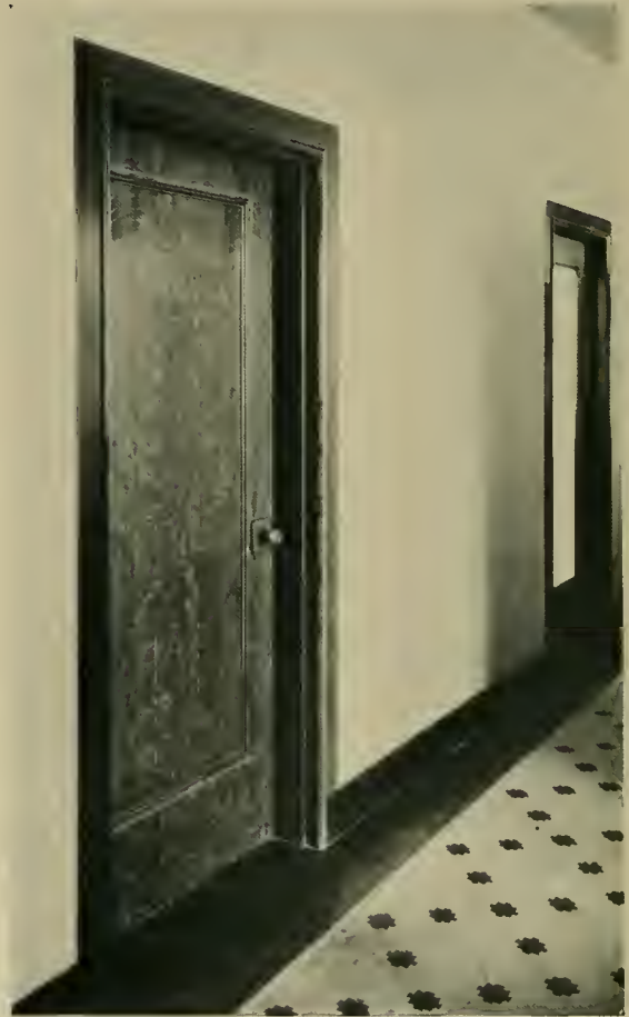
HOLLOW METAL DOOR AND TRIM COAST DIVISION BUILDING
