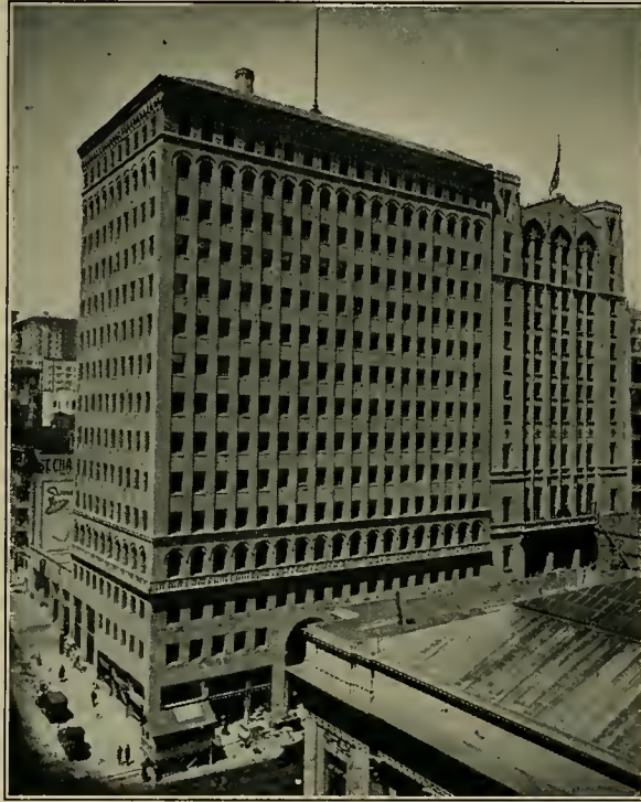
Medico Dental Building and adjacent Elks Club Building, San Francisco
