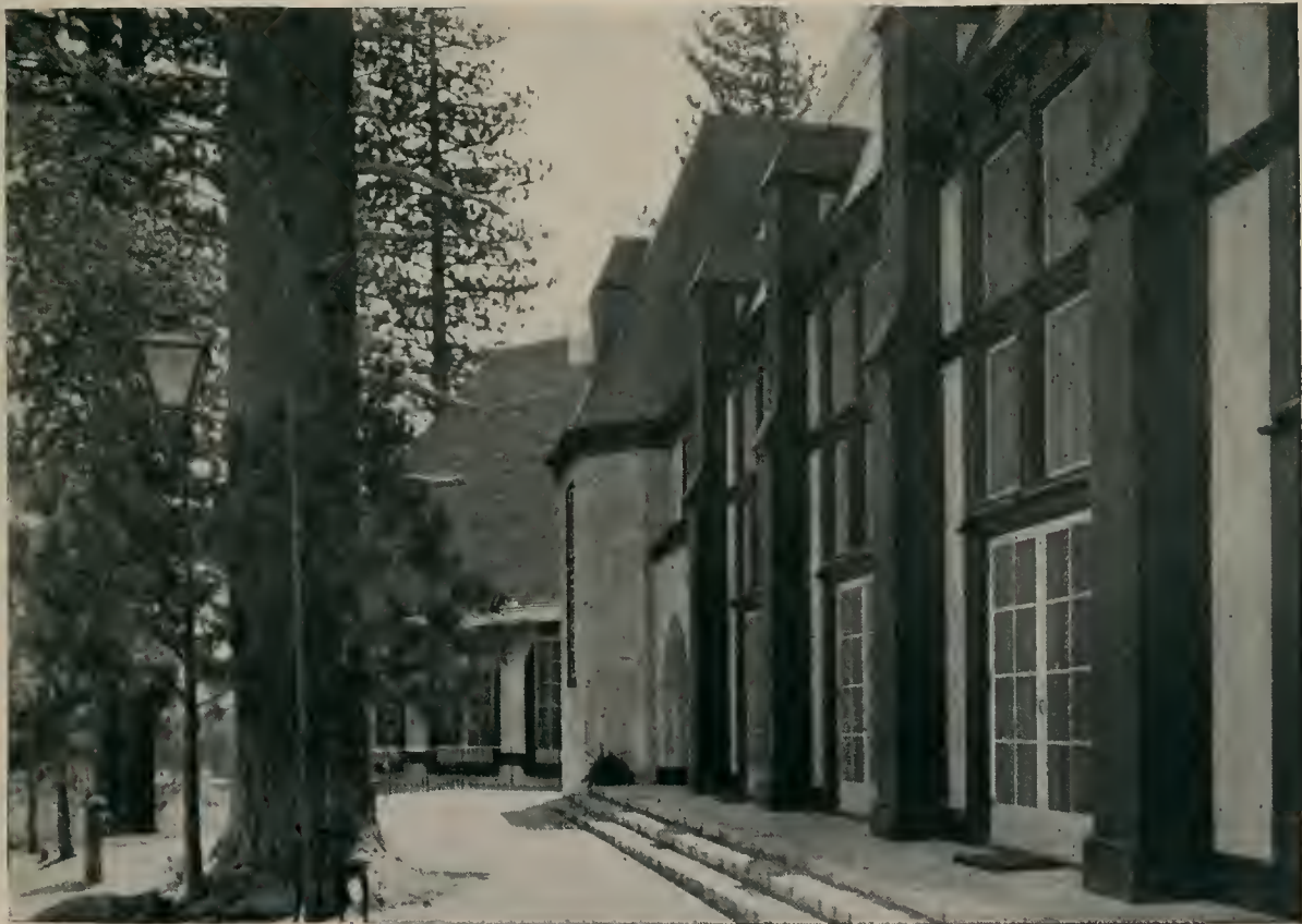
THE GREAT HALL, ARLINGTON LODGE, LAKE ARROWHEAD, CALIFORNIA MCNEAL SWASEY, ARCHITECT, H. C. MCAFEE, ASSOCIATE
