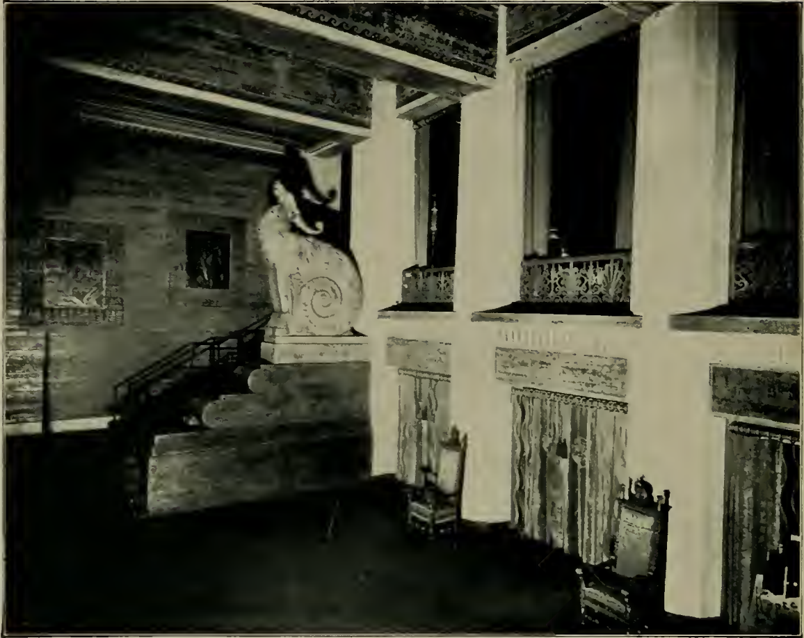
Interior of Grauman Metropolitan Theatre, Los Angeles. Done entirely in concrete. William Lee Woollett, Architect.
