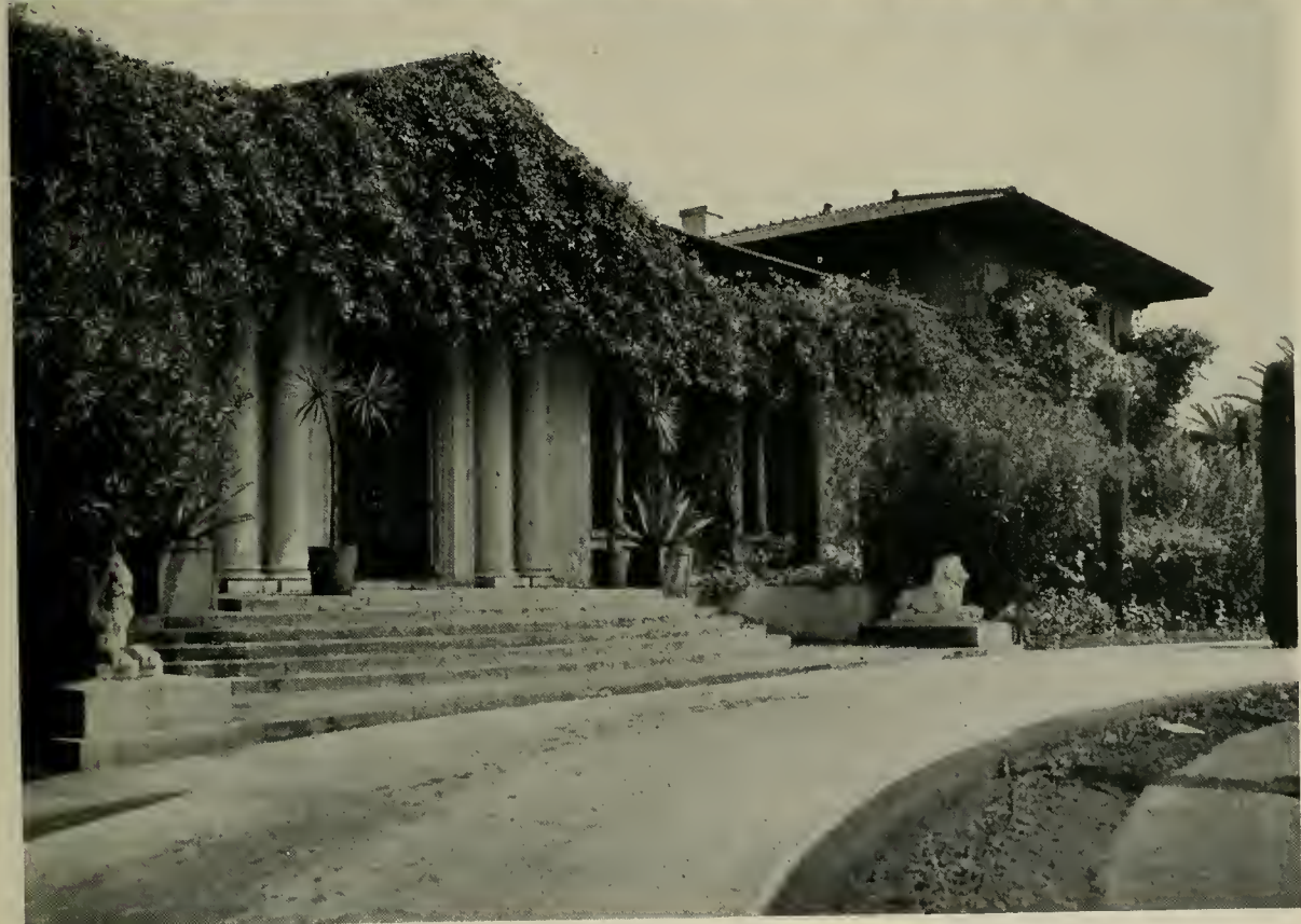
EL MIRASOL, SANTA BARBARA, CALIFORNIA. DELANO AND ALDRICH, ARCHITECT PHOTOGRAPH BY J. WALTER COLLINGE
