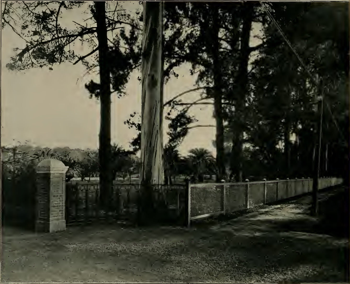
ESTATE OF MR. GEO. L. PAYNE, ATHERTON, CALIFORNIA Page Protection Fence on Redwood Posts
