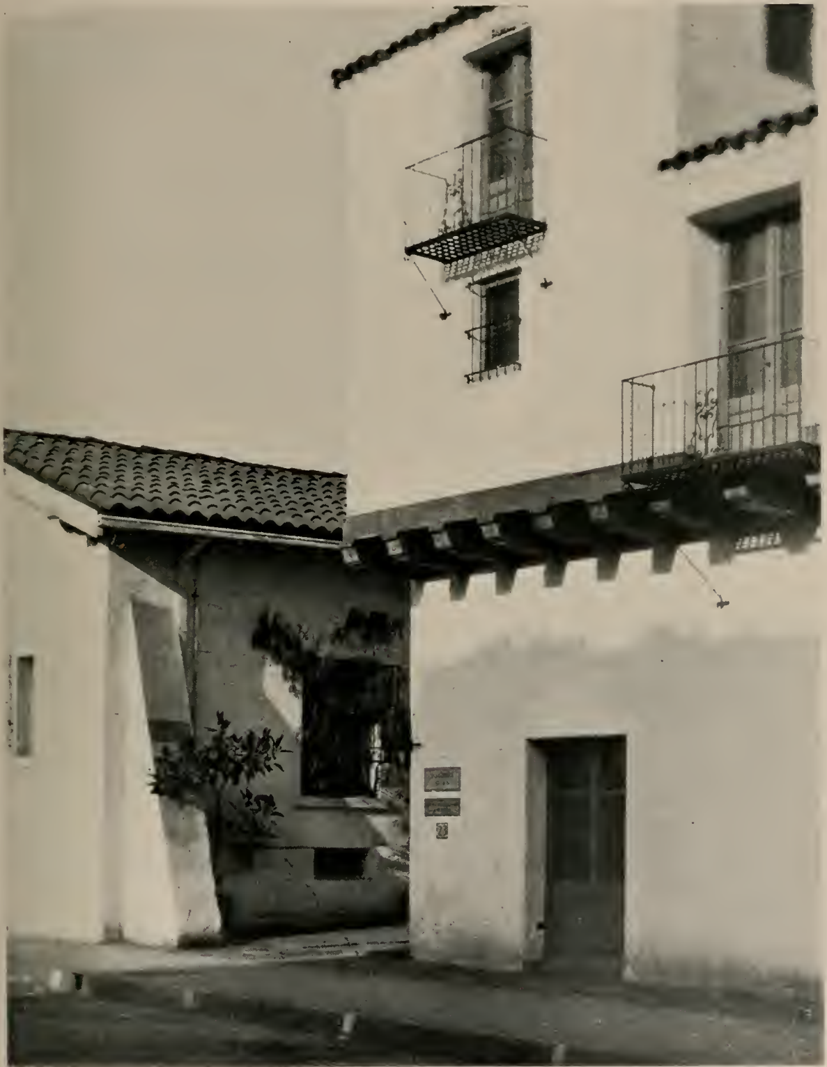
PASSAGE FROM DE LA GUERRA STREET TO COURT "STREET IN SPAIN" SANTA BARBARA, CALIFORNIA JAMES OSBORN CRAIG, ARCHITECT, PHOTOGRAPH BY J. WALTER COLLINGE
