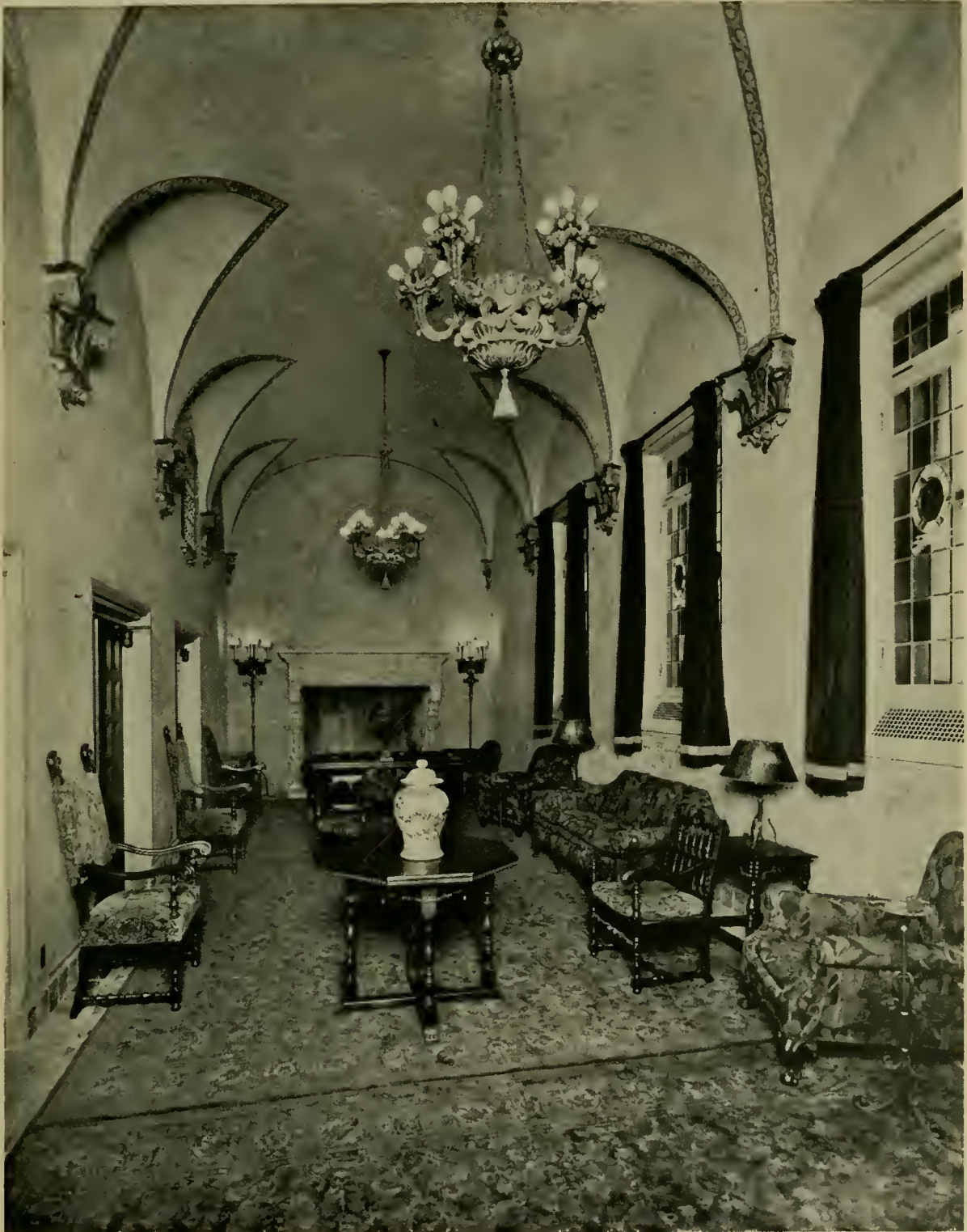
SMOKING ROOM, BILTMORE THEATRE, LOS ANGELES, CALIFORNIA. SCHULTZE & WEAVER, ARCHITECTS
