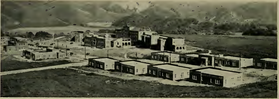
SOME OF THE 24 BUILDINGS OF THE U. S. VETERANS' HOSPITAL AT LIVERMORE
