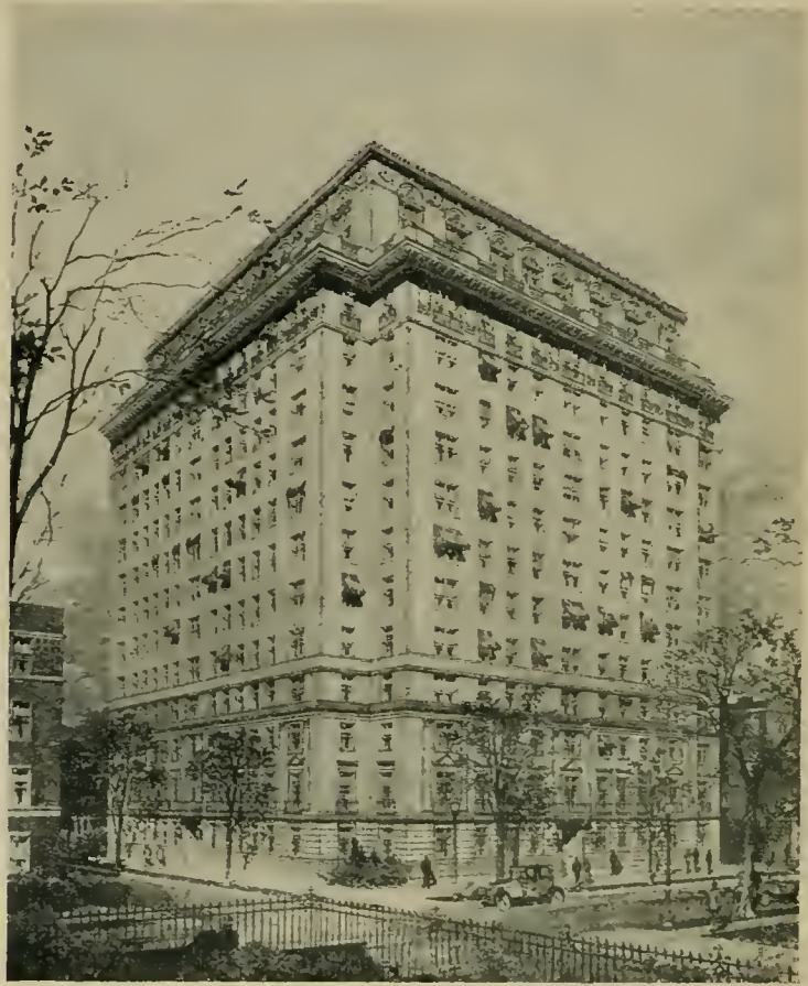
BARRY APARTMENTS, 3100 Sheridan Road, Chicago, Ill. Robert S. De Golyer, Architect; Weil-McLain Co., Jobbers; Carl John Stein Co., Plumbers. 337 Kohler fixtures are installed in this building, among them 133 "Viceroy" built-in baths.
