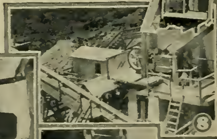
3. Crushed gypsum flowing into automatic hopper of tramway.
