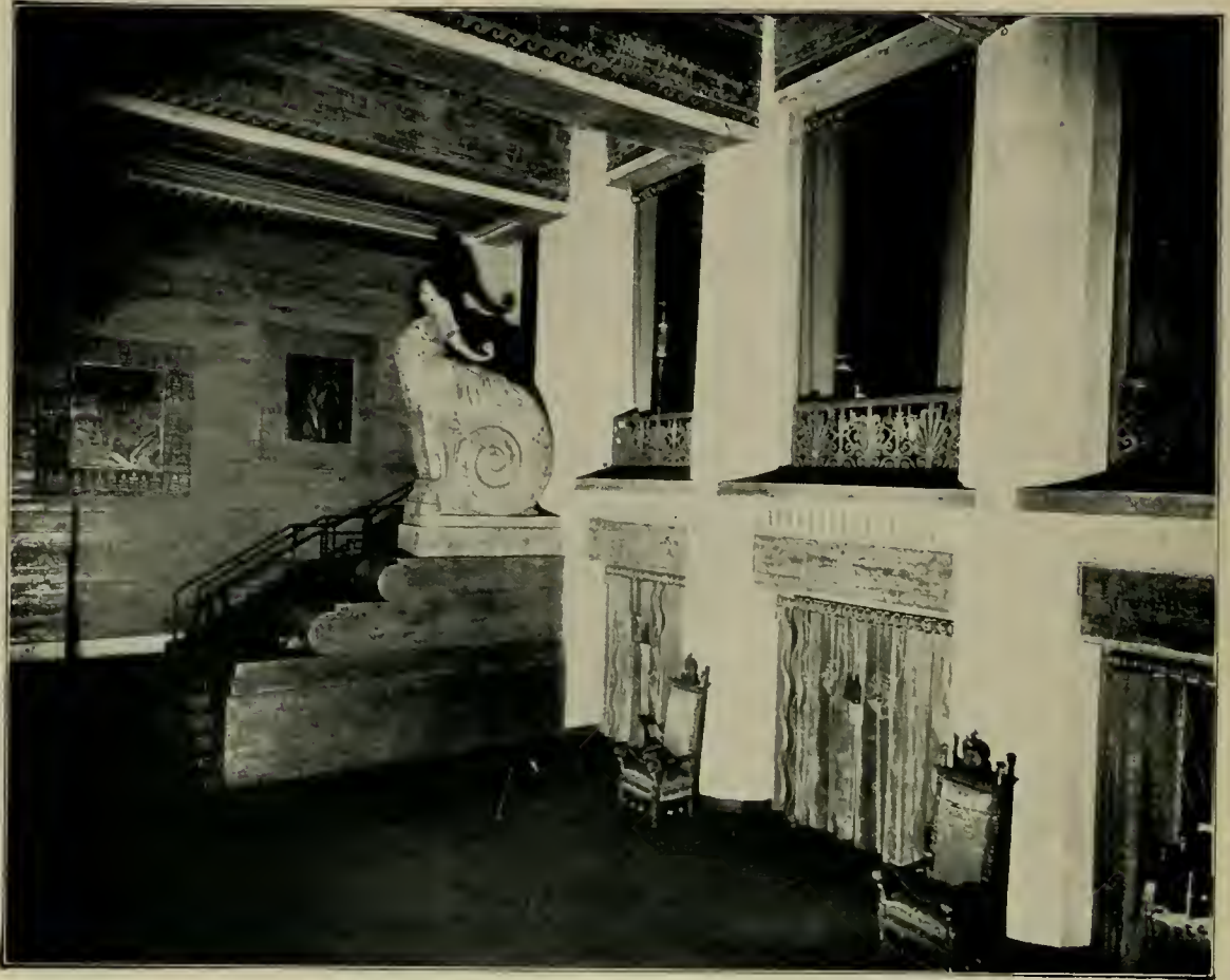
Interior of Grauman Metropolitan Theatre, Los Angeles. Done entirely in Concrete. William Lee Woollett, Architect.
