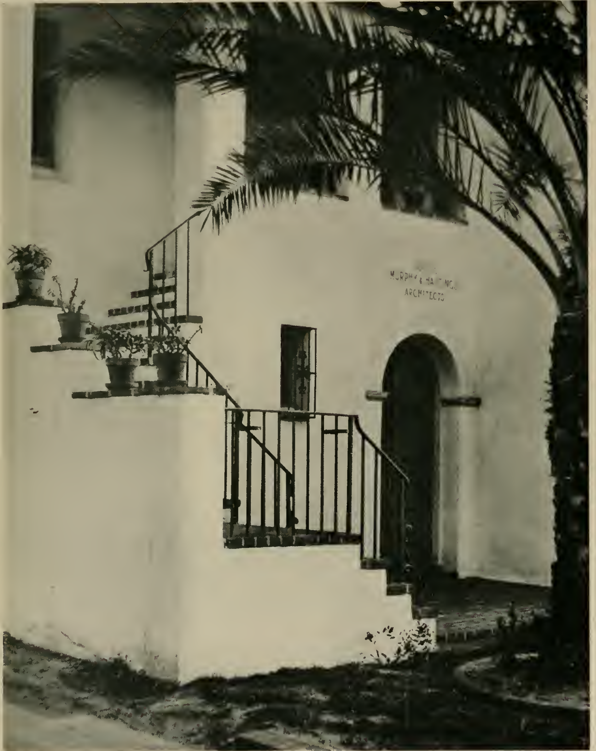
OFFICES OF SOULE, MURPHY AND HASTINGS, ARCHITECTS, SANTA BARBARA, CALIFORNIA
