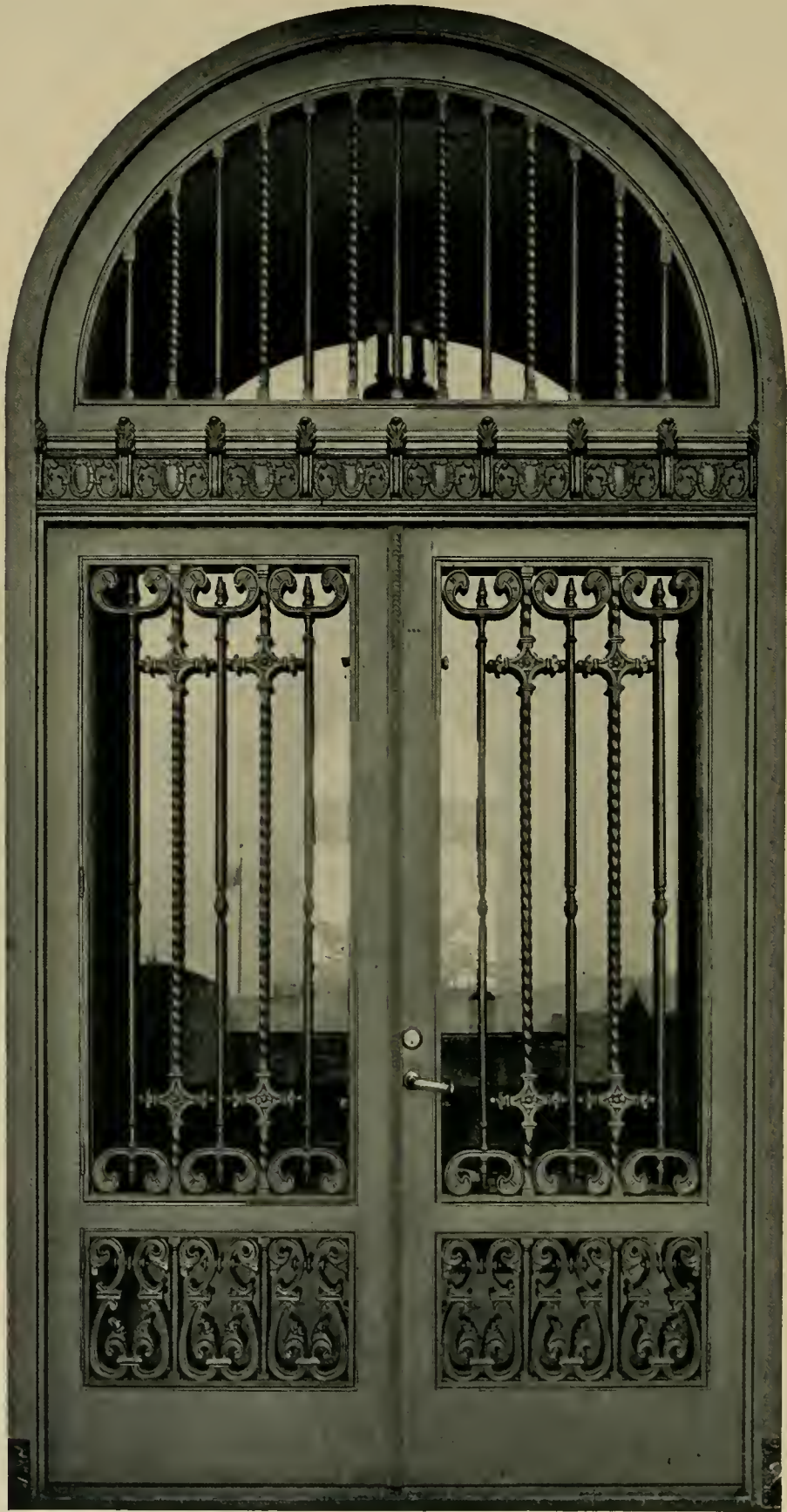
Main Entrance, Crest View Apartments JOSEPH L. STEWART, Architect
