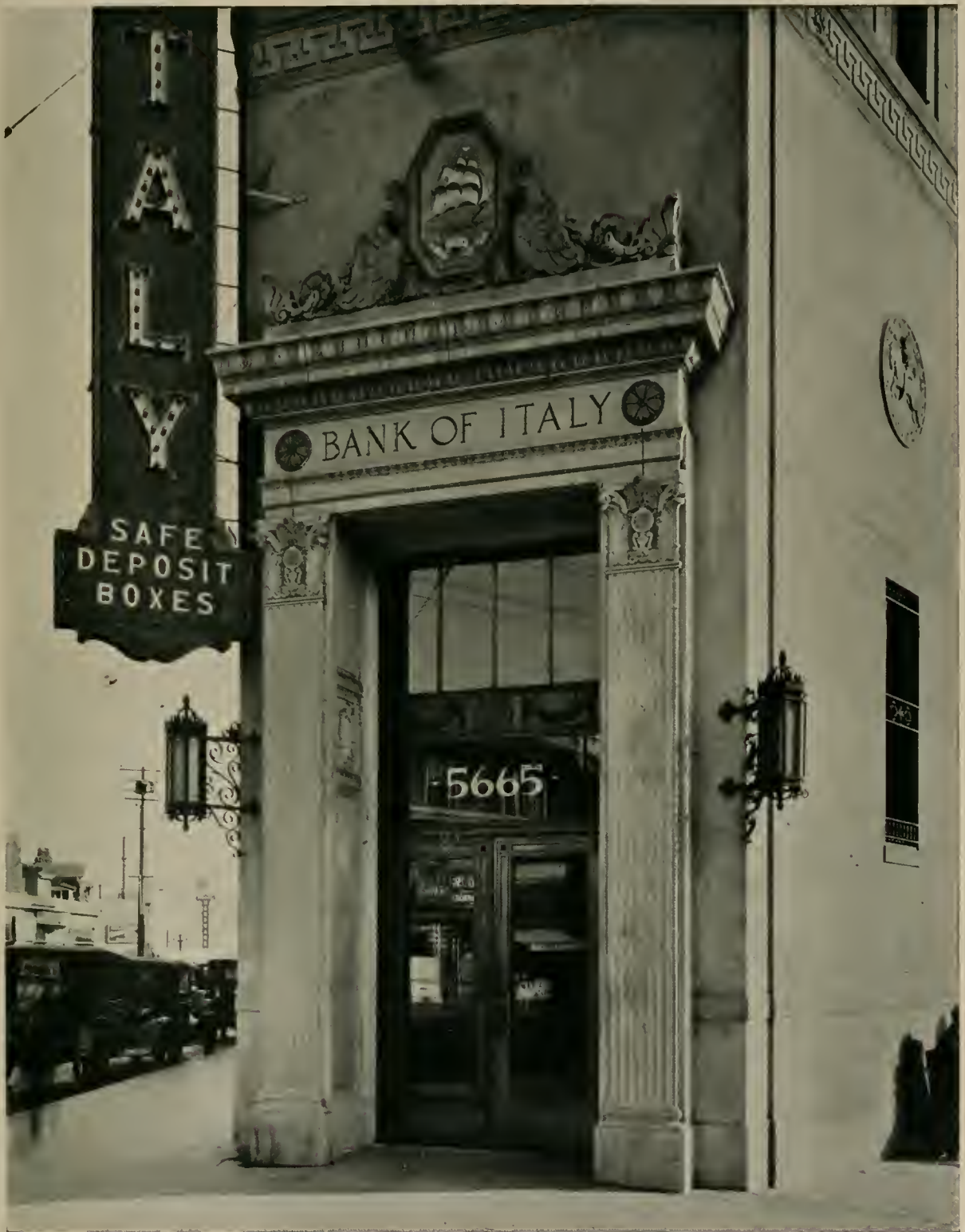
ENTRANCE DETAIL, COLLEGE AVENUE BRANCH, BANK OF ITALY, BERKELEY, CALIFORNIA. H. A. MINTON, ARCHITECT
