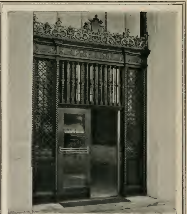
Liberty Bank Building, San Francisco. H. A. Minton, Architect Ornamental Iron Entrance and Bronze Teller Cages Show True Craftsmanship.
