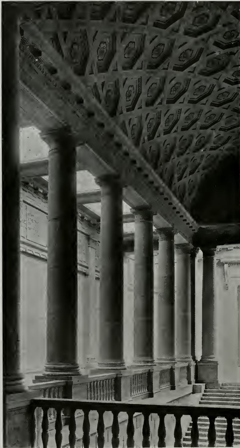
Stair Hall, Looking Toward Delivery Room
