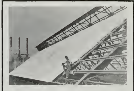
ASBESTOS CORRUGATED ROOFING BEING APPLIED
