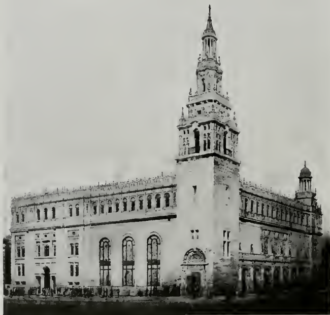
FIRST METHODIST EPISCOPAL CHURCH LOS ANGELES JOHN C. AUSTIN, Architect
