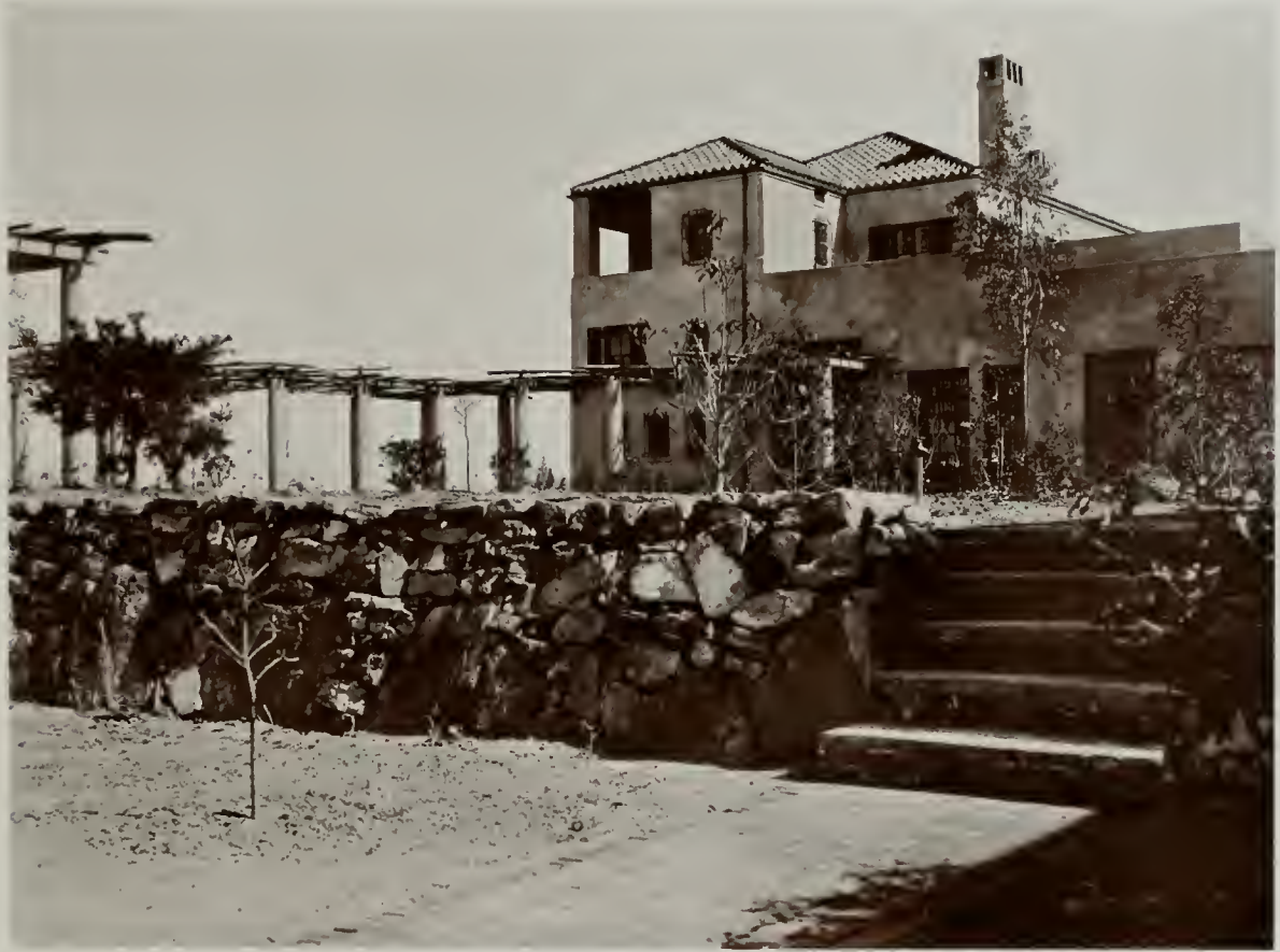
RESIDENCE OF E. M. FOWLER, CHINO, CAL. MYRON HUNT, ARCHITECT
