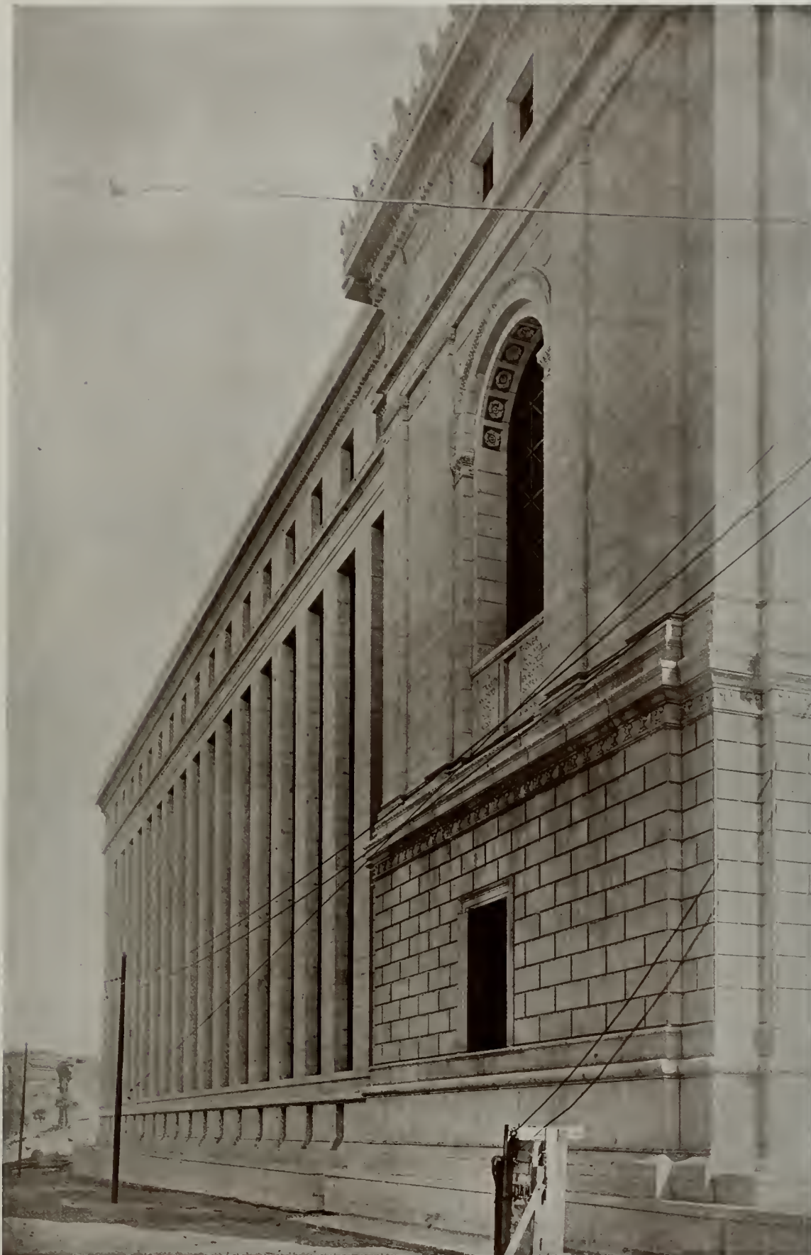
McALLISTER STREET FACADE
