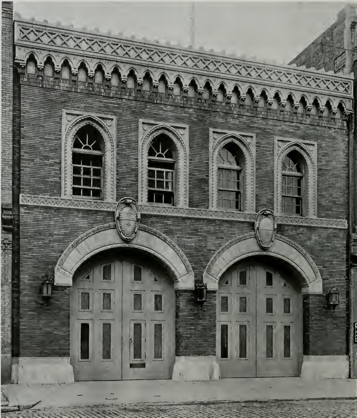
SAN FRANCISCO FIRE DEPARTMENT - ENGINE No. 4
