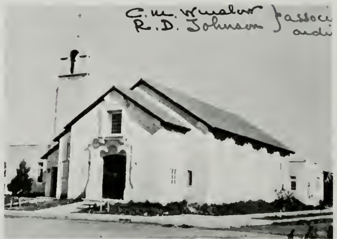
LA JOLLA CONGREGATIONAL CHURCH C. M. WINSLOW AND R. D. JOHNSON Associate Architects
