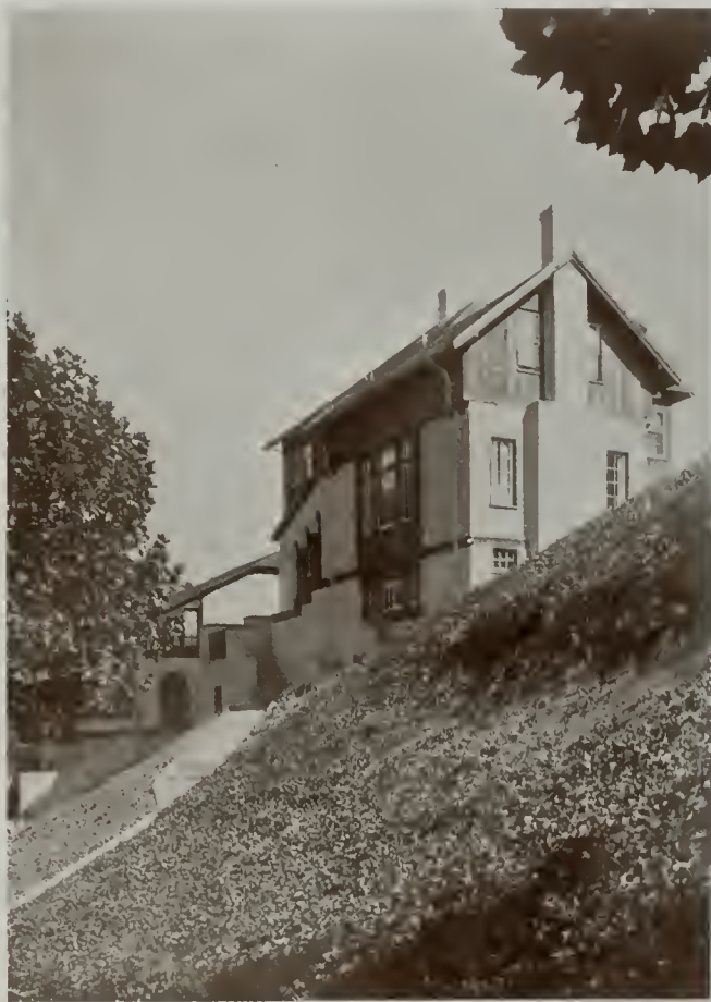
RESIDENCE OF W. E. SHOCKLEY, CLAREMONT, BERKELEY, CALIFORNIA HENRY H. GUTTERSON, ARCHITECT
