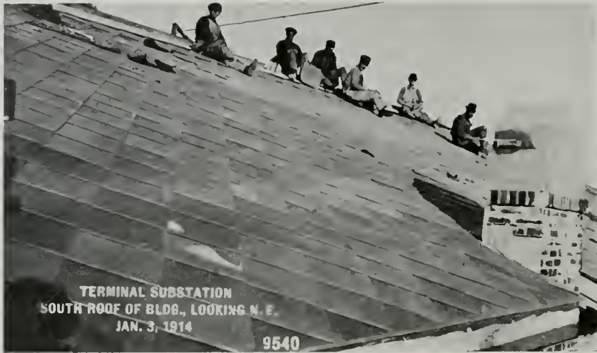
APPLYING "AMBLER ASBESTOS SHINGLES" TO ROOF
