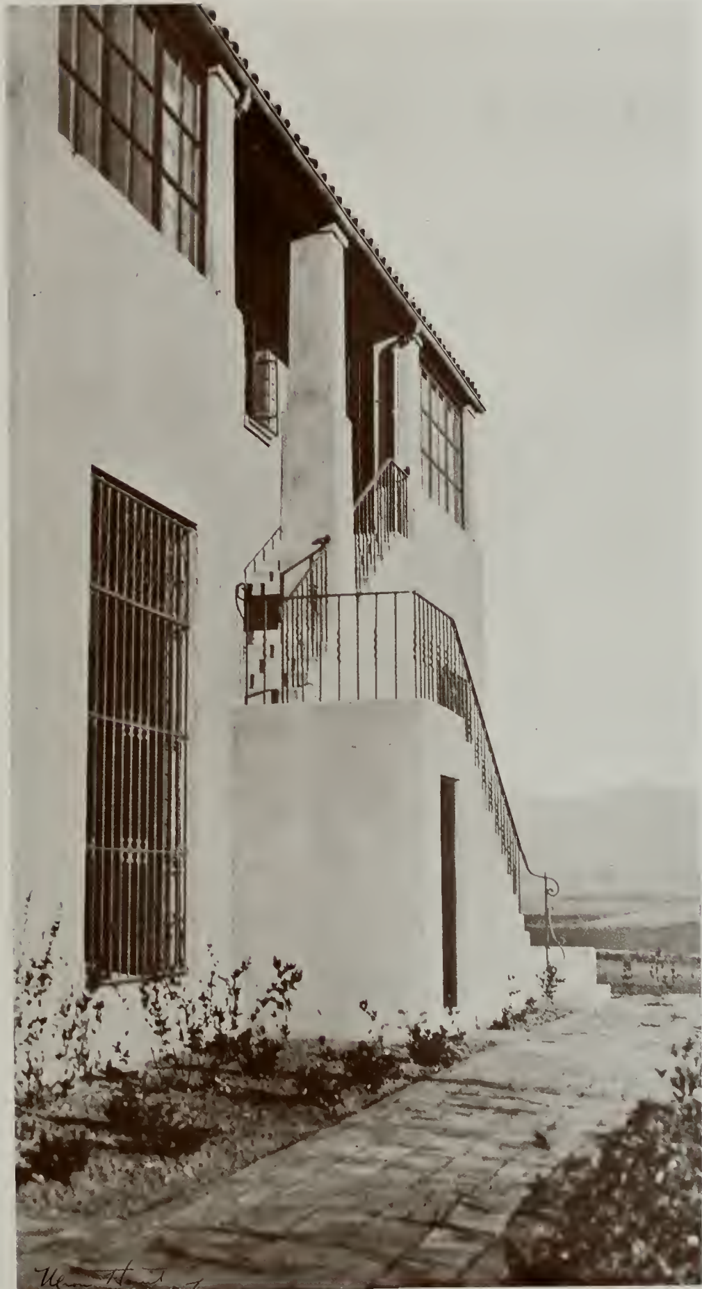
DETAIL OF E. M. FOWLER RESIDENCE, CHINO, CAL. MYRON HUNT, ARCHITECT.
