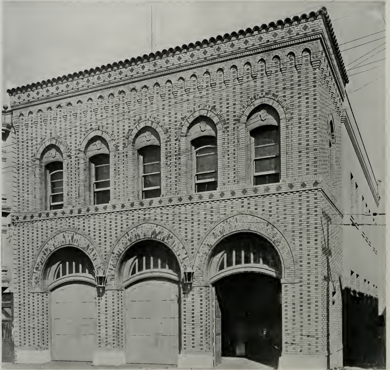
SAN FRANCISCO FIRE DEPARTMENT, ENGINE NO. 5
