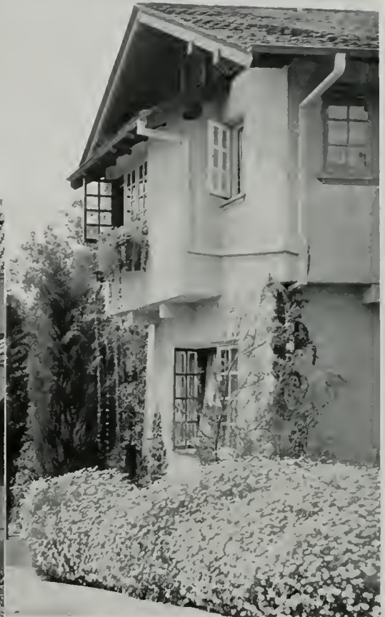
Detail, residence of Architect Elmer Grey, Pasadena, Cal. "Bay State Coating" applied.
