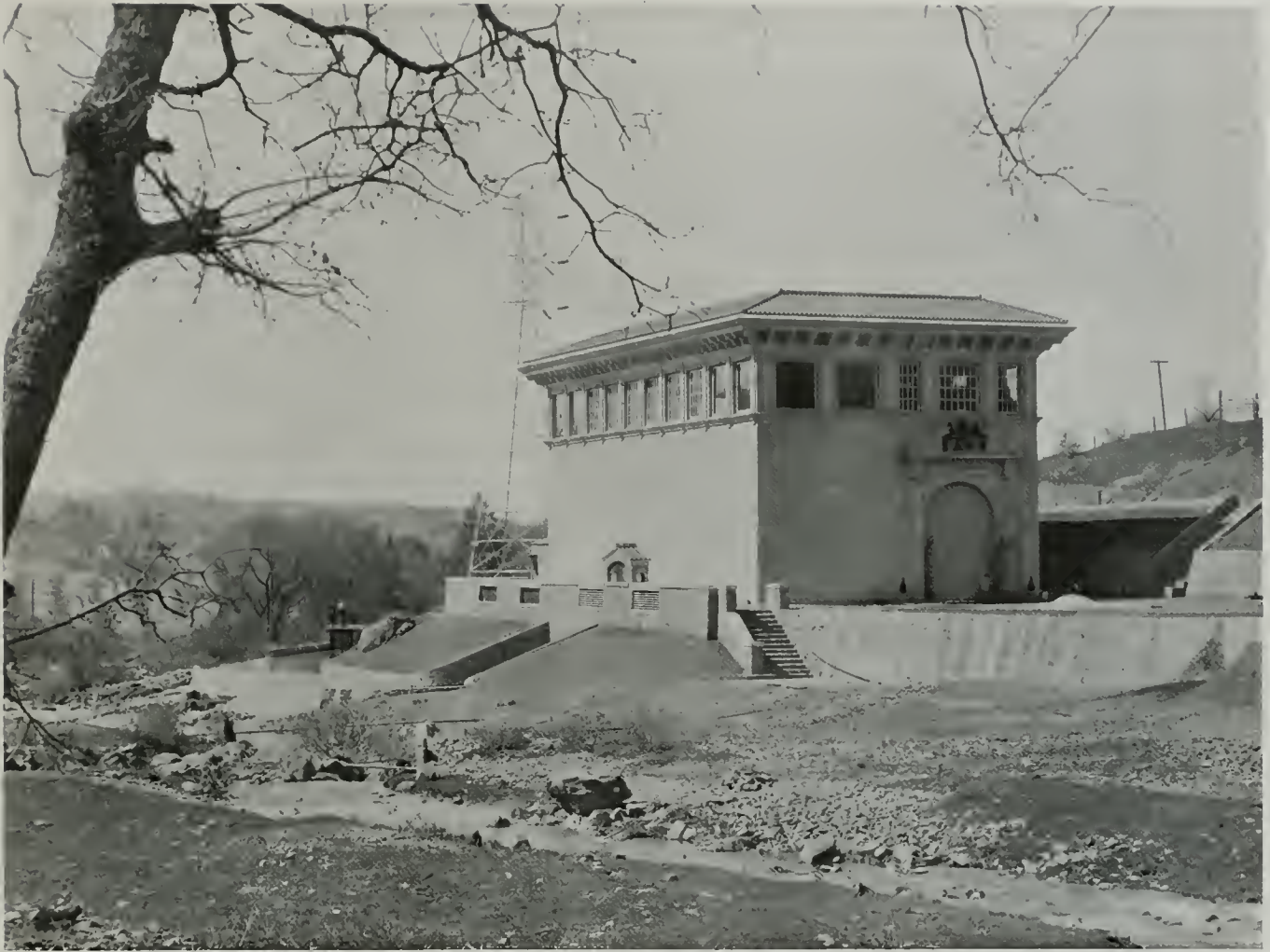
WISE POWER HOUSE OF PACIFIC GAS & ELECTRIC CO. AUBURN RAVINE, PLACER COUNTY, CAL.
