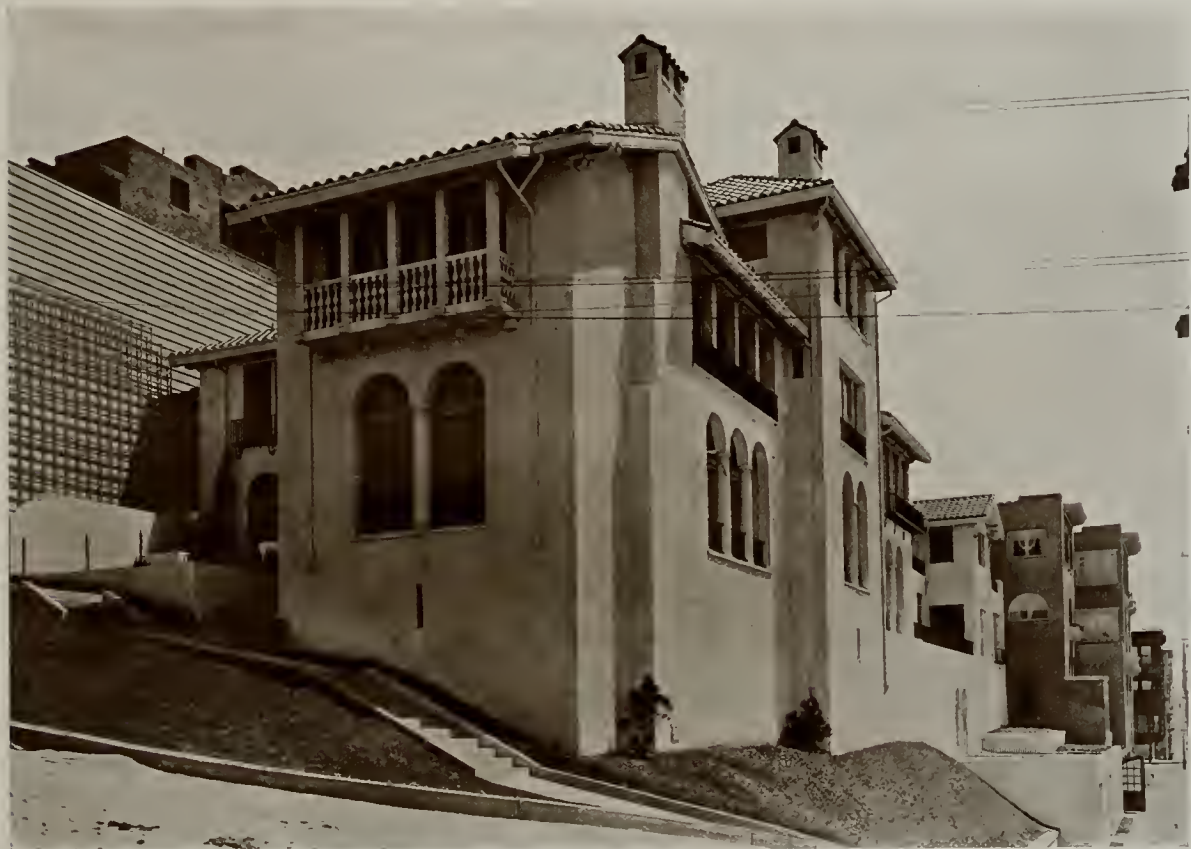
COMMUNITY APARTMENTS FOR HORATIO P. LIVERMORE, SAN FRANCISCO C. W. McCALL, ARCHITECT
