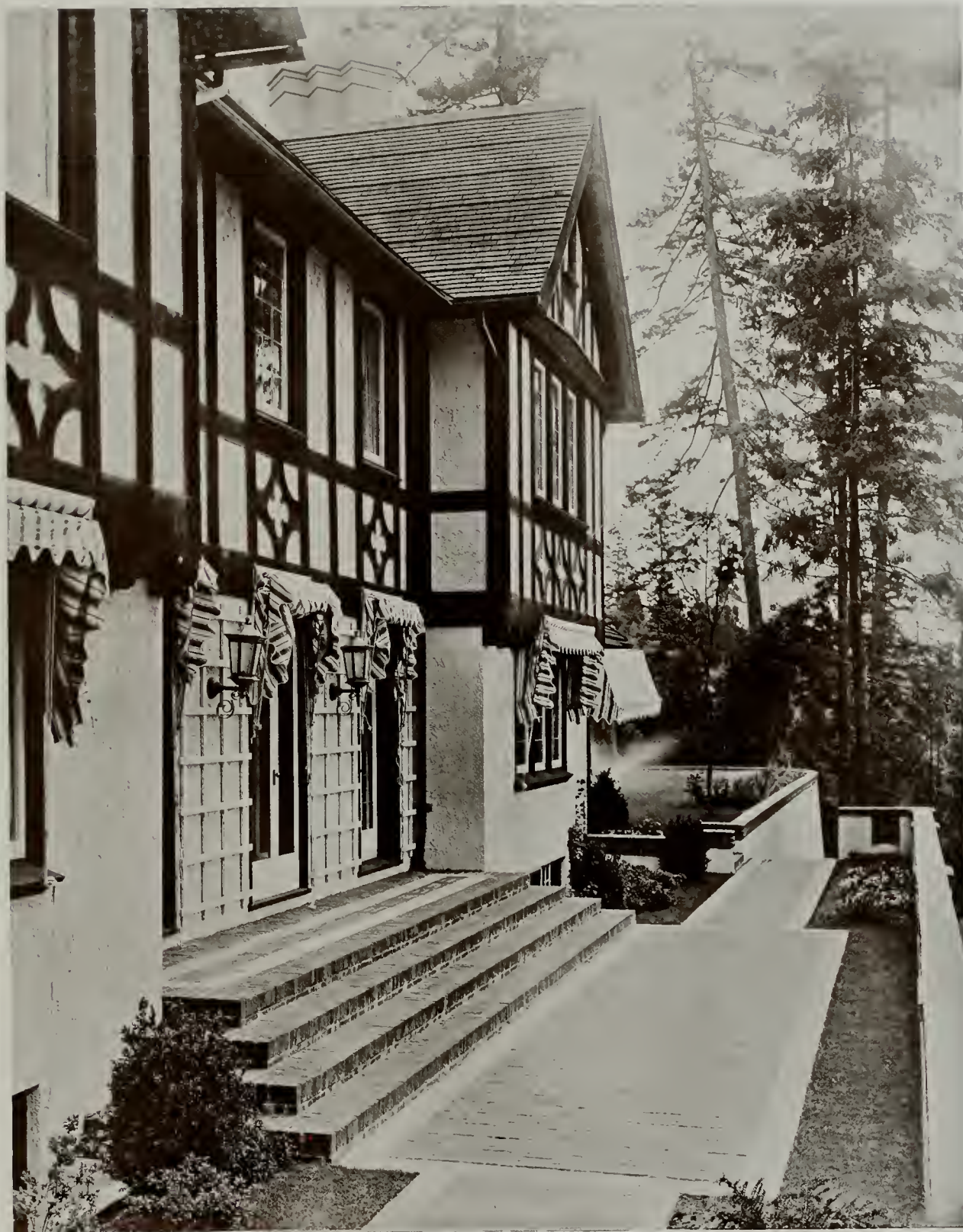
DETAIL M. A. ARNOLD RESIDENCE AT "THE HIGHLANDS," NEAR SEATTLE DAVID J. MYERS, ARCHITECT
