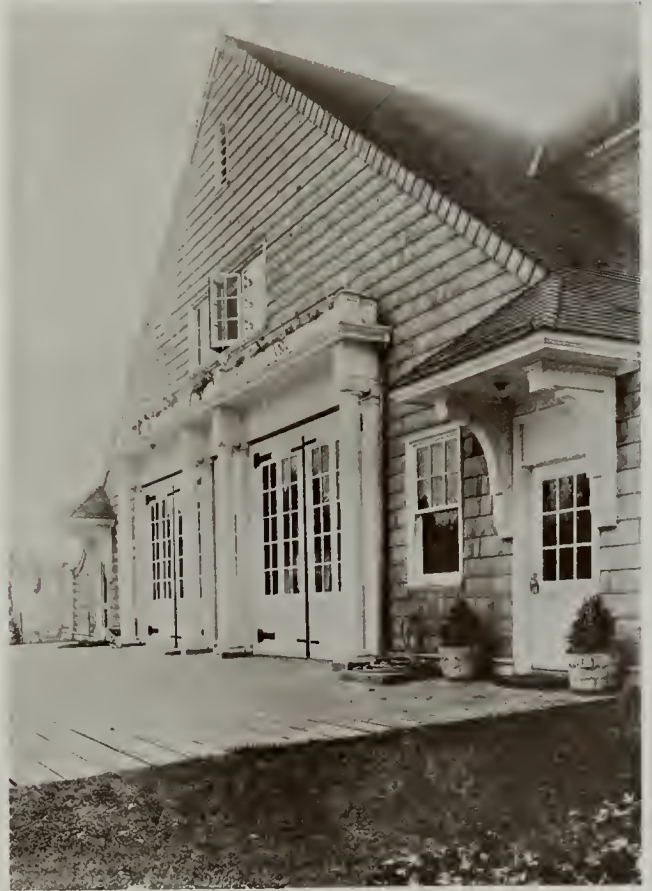
DETAIL OF FIRE STATION, WEST SEATTLE
