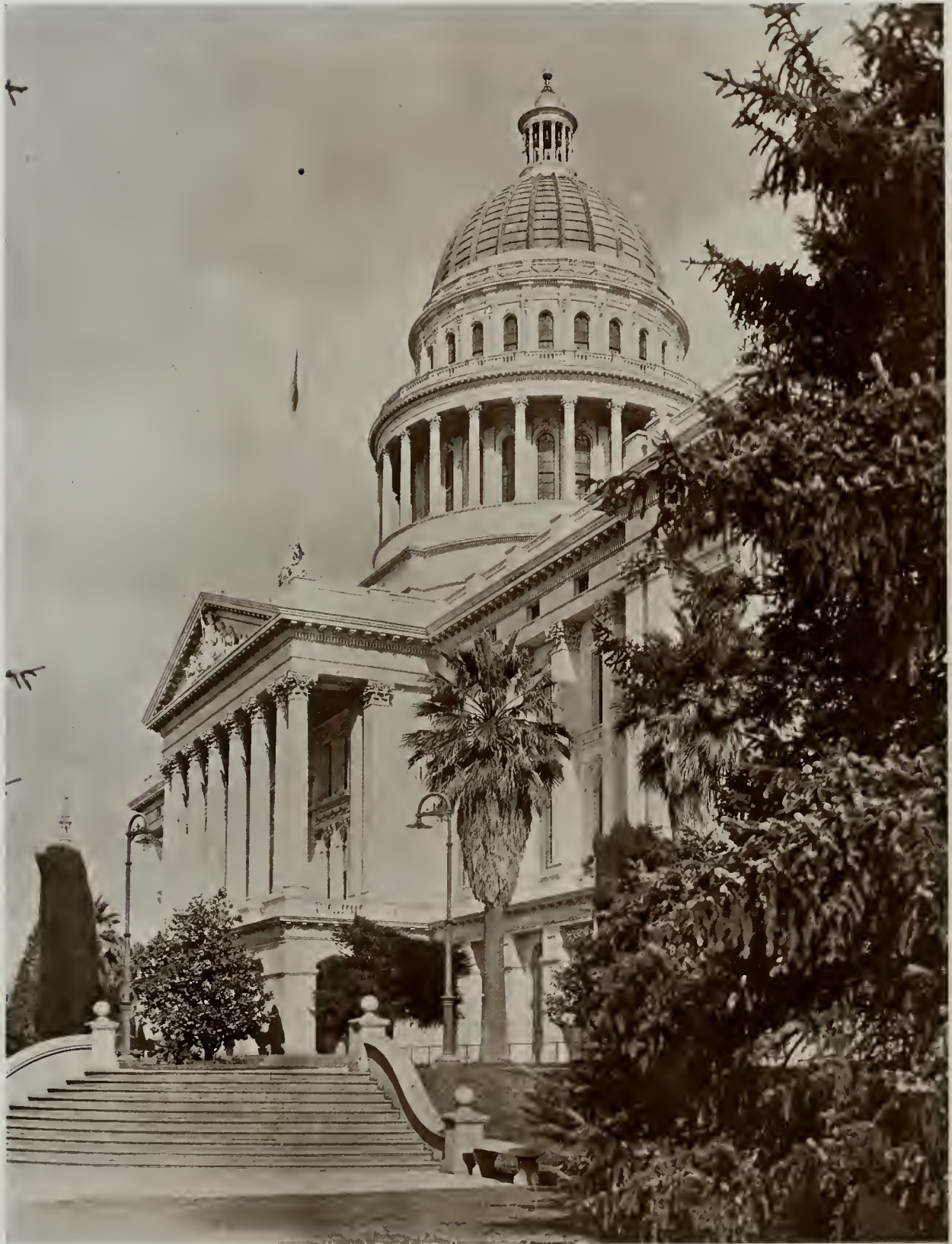
DETAIL MAIN ENTRANCE CALIFORNIA STATE CAPITOL BUILDING
