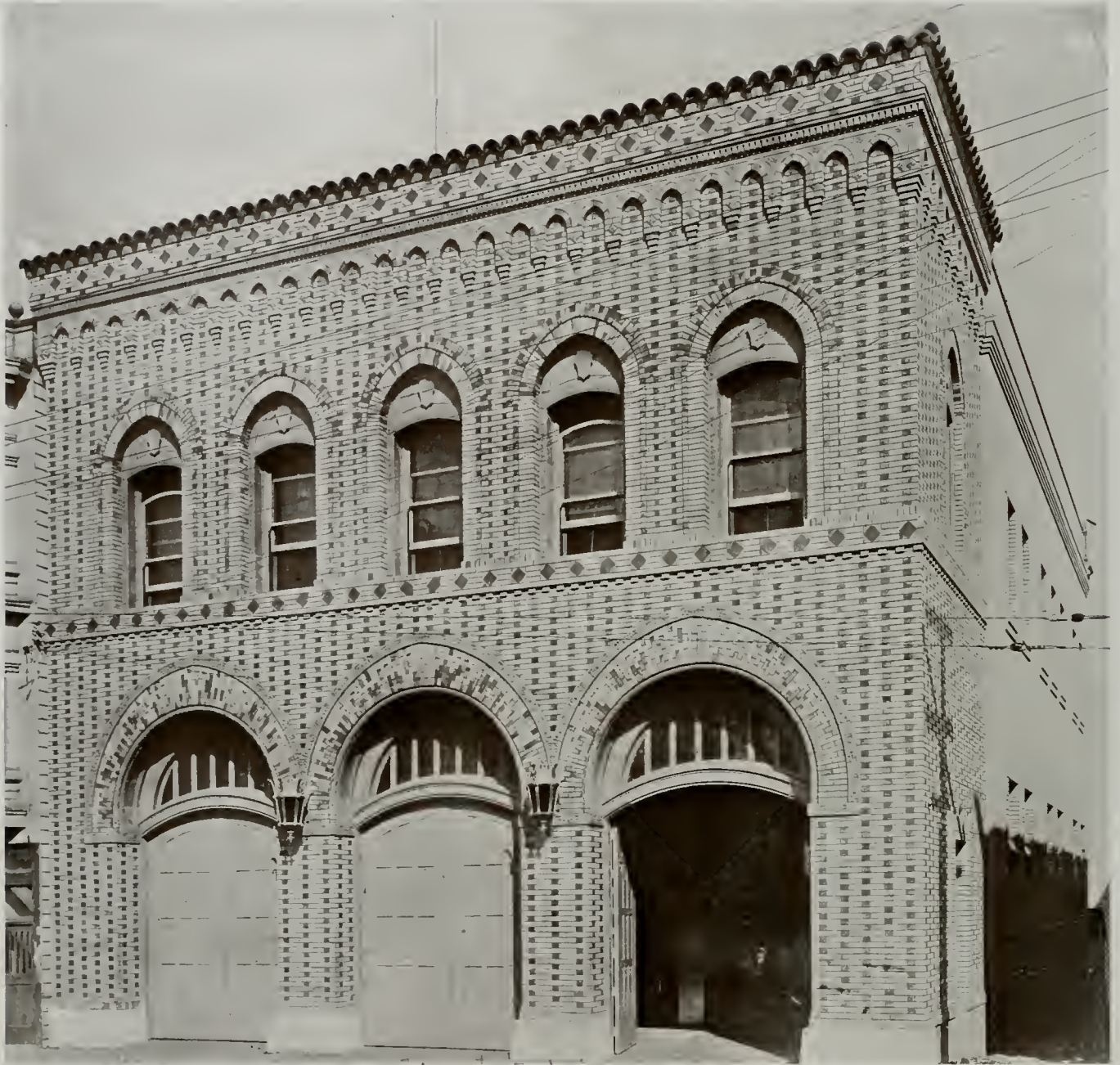
SAN FRANCISCO FIRE DEPARTMENT, ENGINE NO. 5
