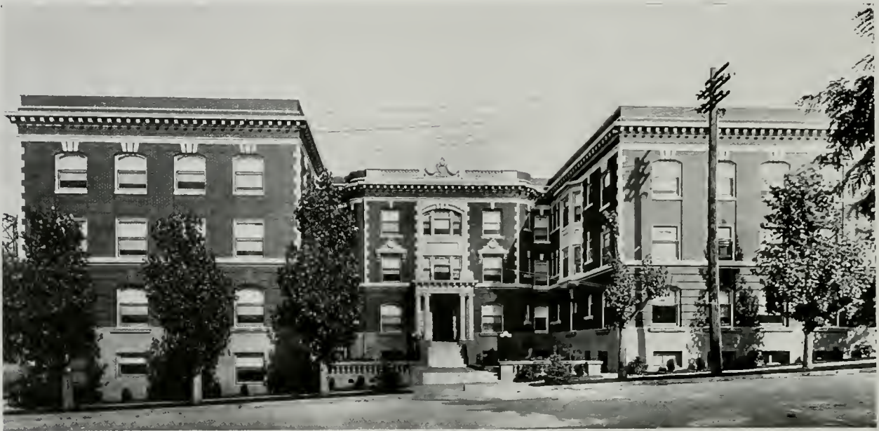
KNICKERBOCKER APARTMENTS, SPOKANE, WASH. ALBERT HELD, ARCHITECT
