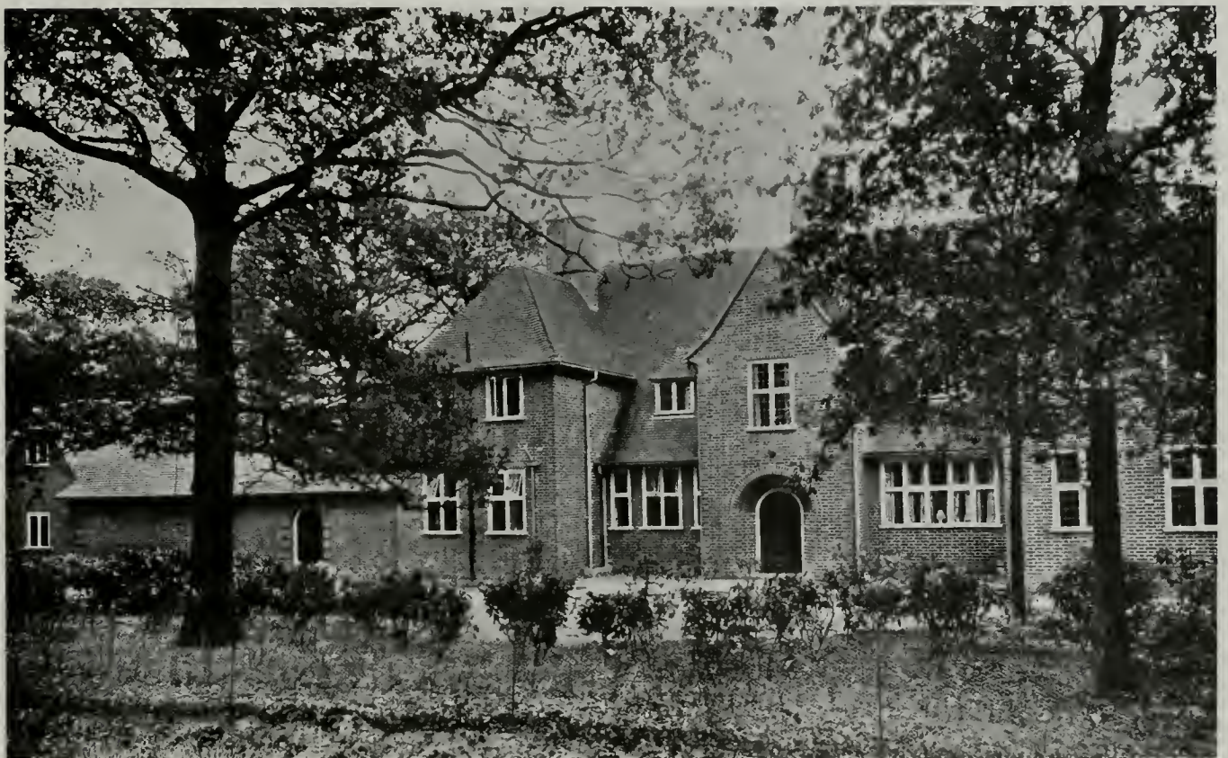
ENTRANCE FRONT. HOMEWOOD HOUSE, CUFFLEY, HERTS ALLEN & THOMPSON, ARCHITECTS
