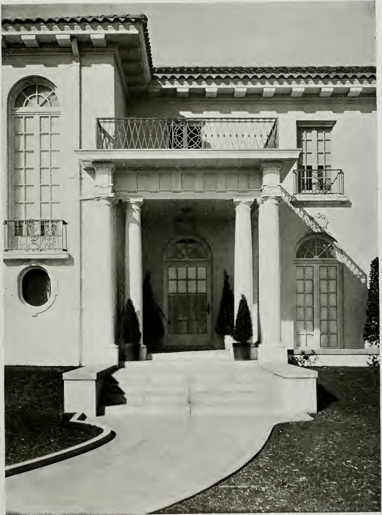
DETAIL OF ENTRANCE HOUSE OF C. F. PERRY, HOLLYWOOD, CAL. B. COOPER, CORBETT, ARCHITECT
