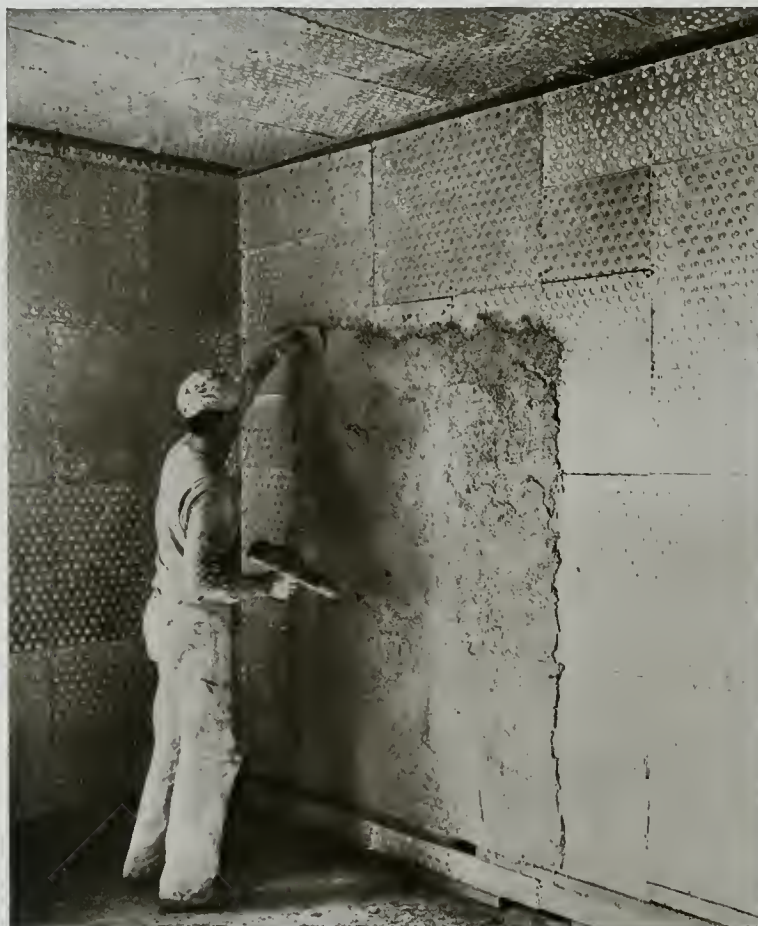
A BUTTONLATHED ROOM IN THE MAKING
