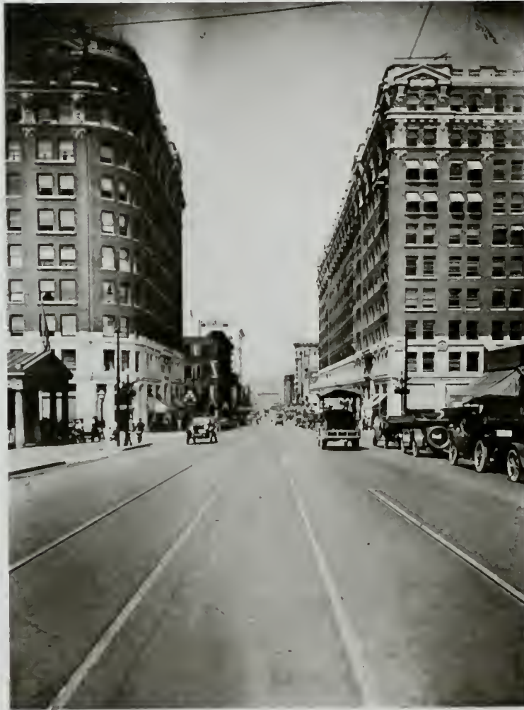
Creosoted Wood Block Pavement on Fourth Avenue, Seattle, after almost 7 years of service. This is the highest developed office district in Seattle and this quiet pavement is much appreciated.
