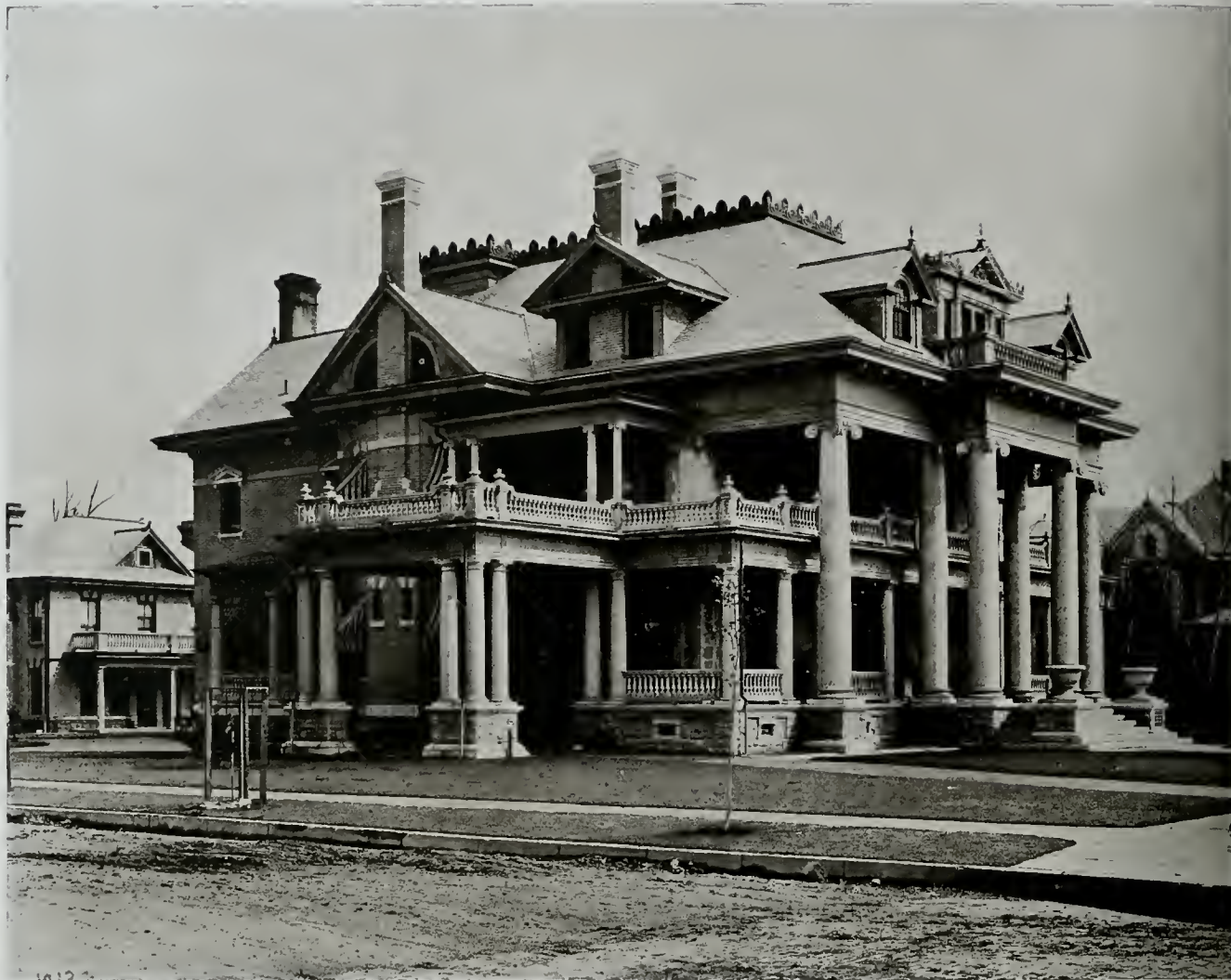
RESIDENCE OF E. W. TWADDELL
