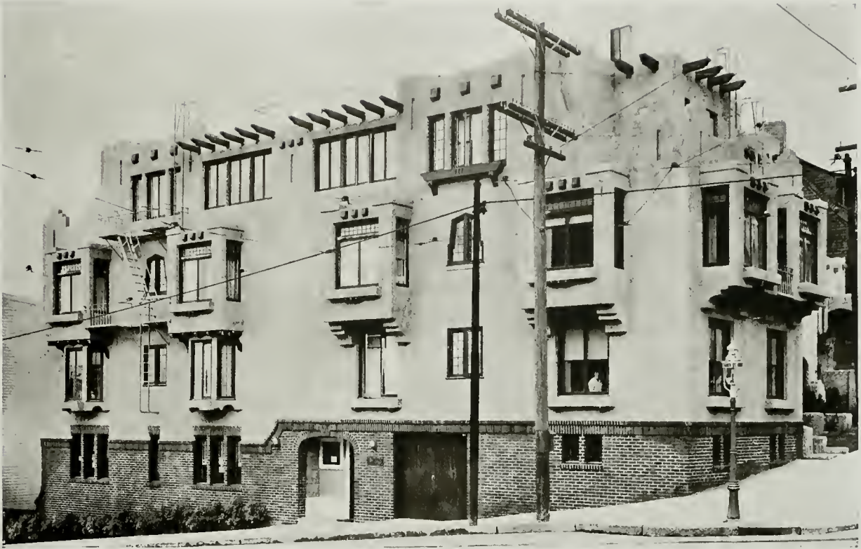
MAC ROTH APARTMENTS, SAN FRANCISCO ROUSSEAU & ROUSSEAU, ARCHITECTS
