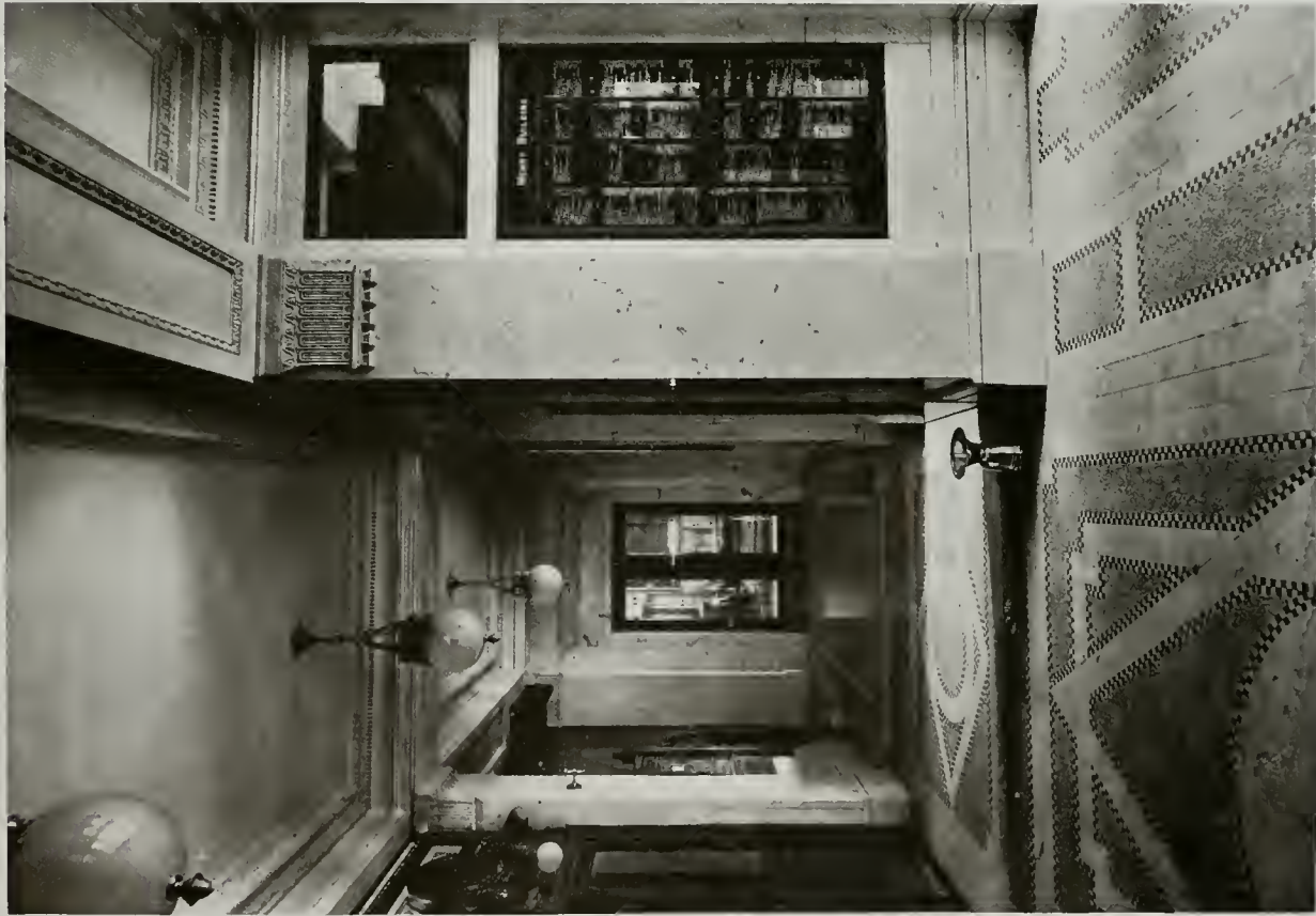
ELEVATOR HALL OF HENRY BUILDING, SEATTLE Howells and Stokes, Architects, A. H. Albertson, Associate The main entrance is directly across the hall from the elevators. Stairs start at the right at each end of the hall. The floors are in marble and mosaic border with terrazzo panels. The side walls are Italian marble.
