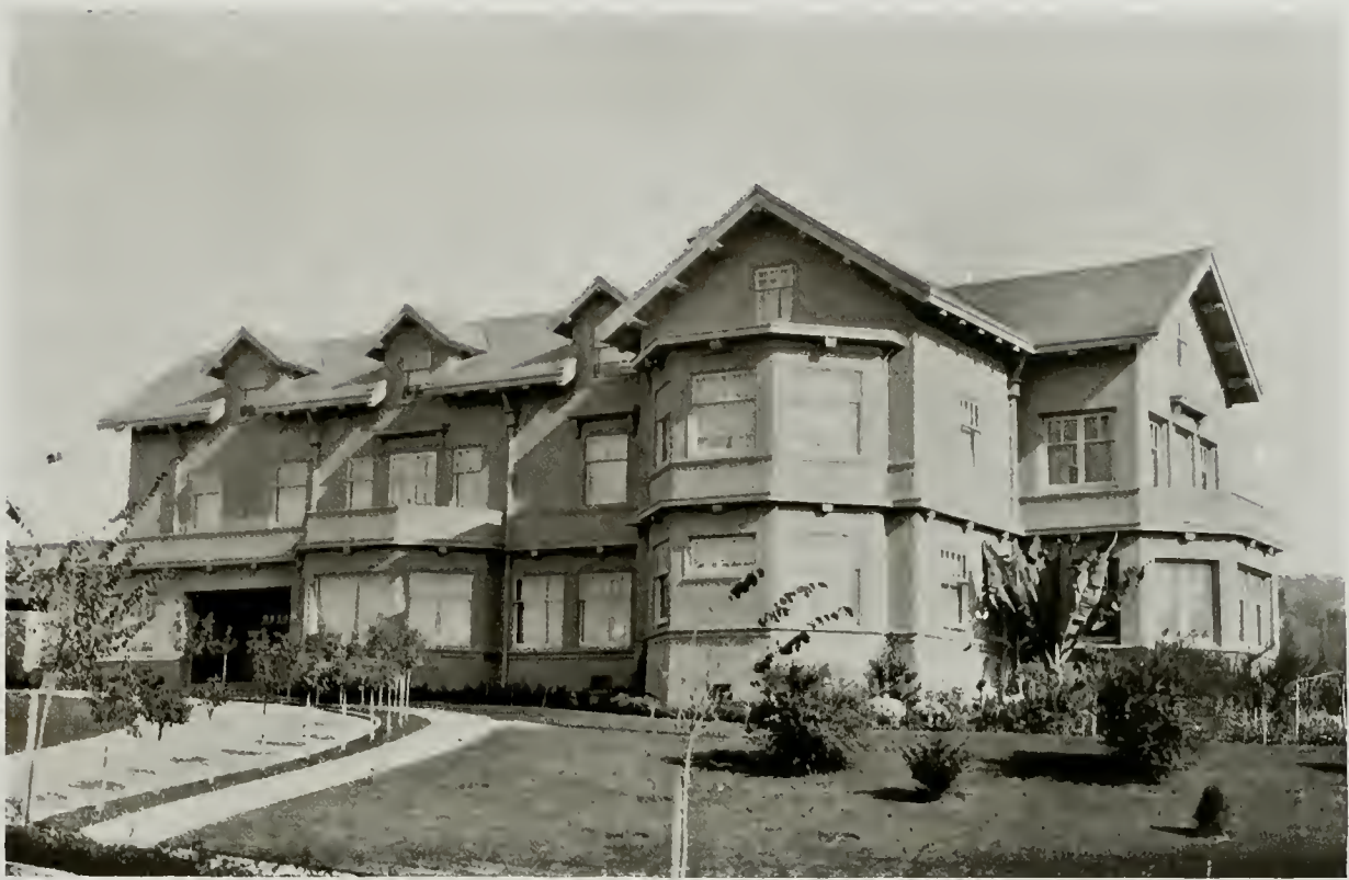
HOME OF MRS. S. T. ALEXANDER, PIEDMONT, CAL. C. W. DICKEY, ARCHITECT
