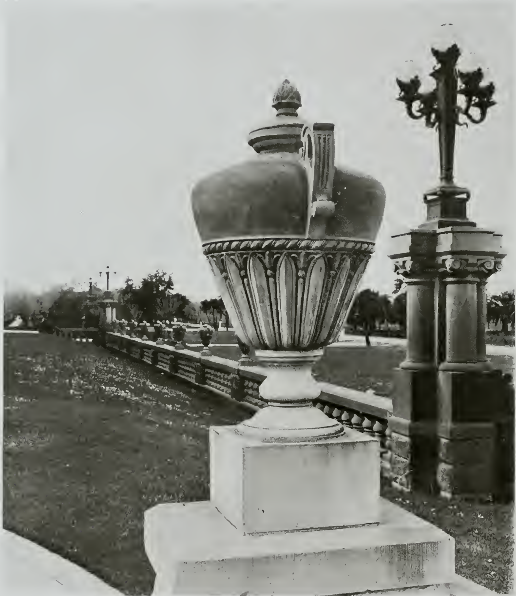
One of the many Terra Cotta Urns surmounting and perfectly matching the buff sandstone of buildings in quadrangle of Stanford University
