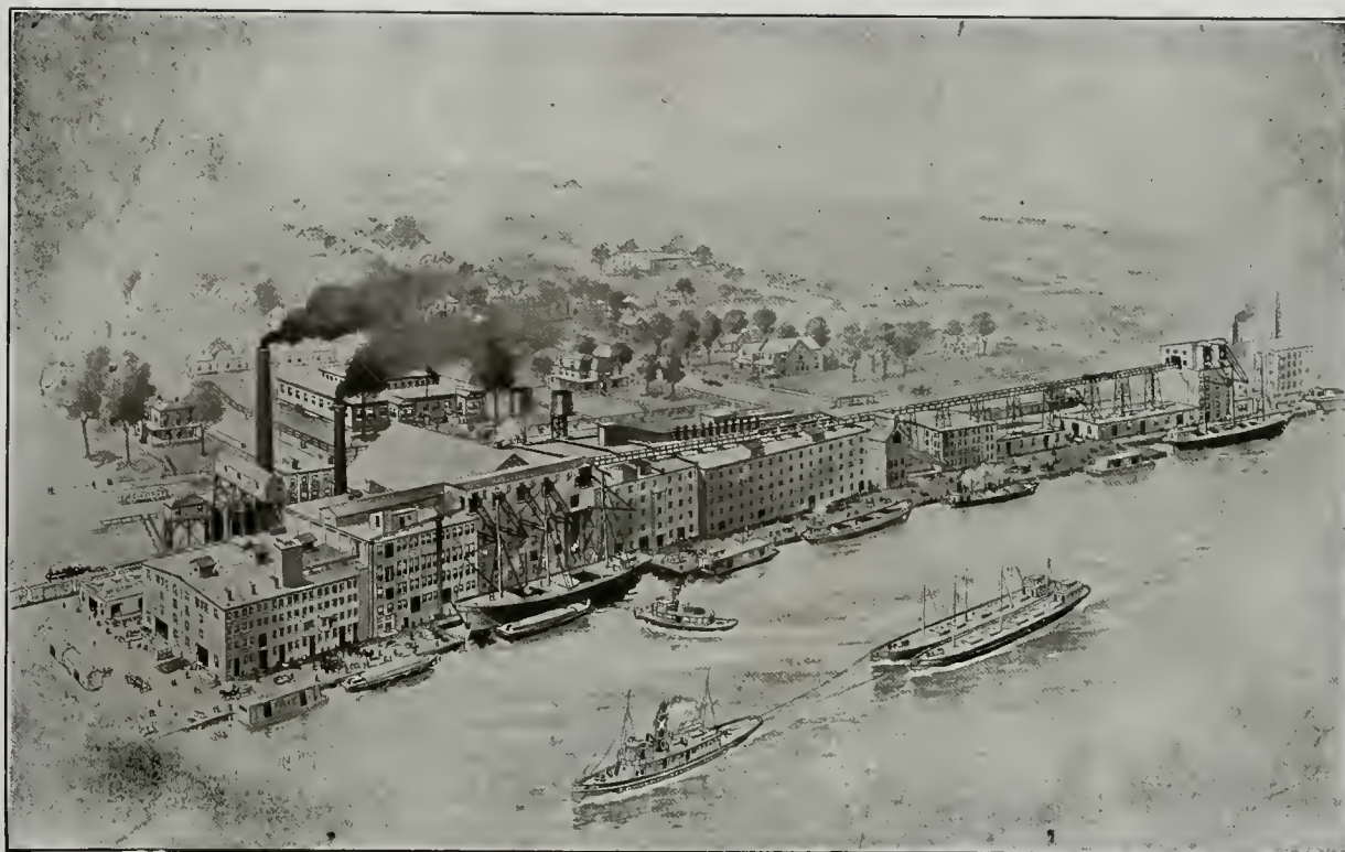
Main Office and Works, the Muralo Company, New Brighton, N. Y.
