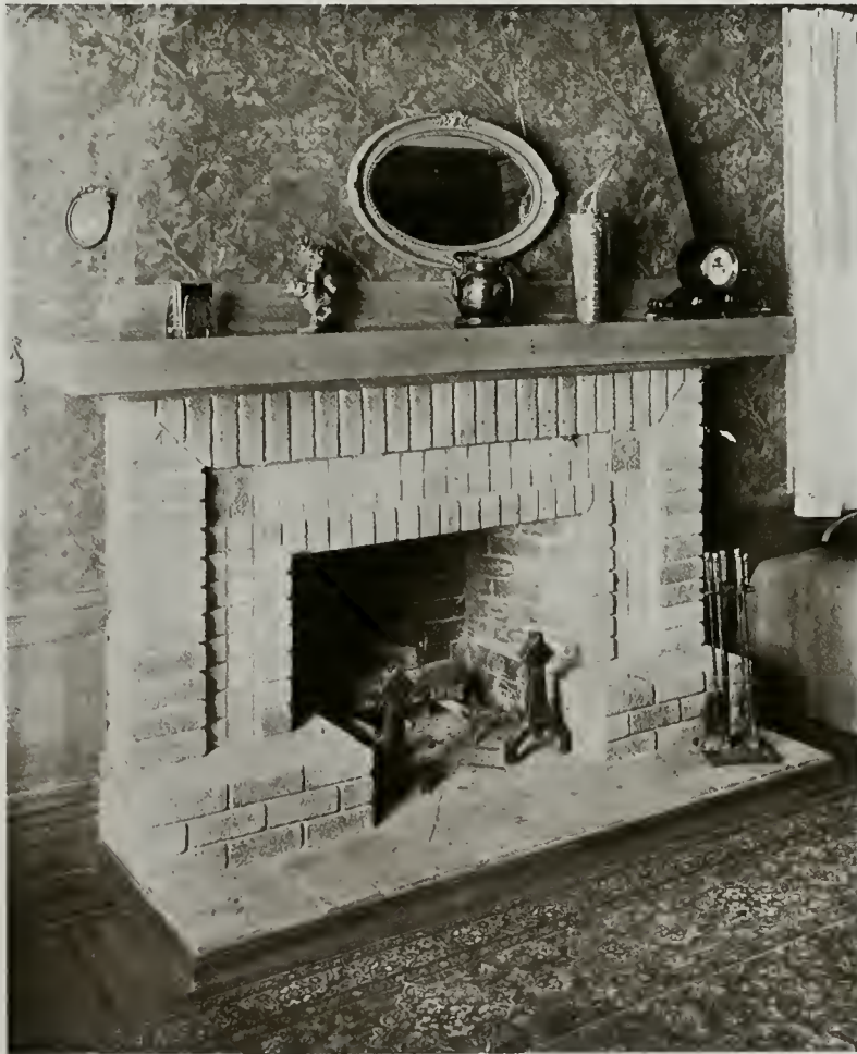
Living Room Fireplace, by Enri H. Richardson. Colors, mulberry brown and dull blue. Hearth in brown quarry tile. Butchelder tile insert.
