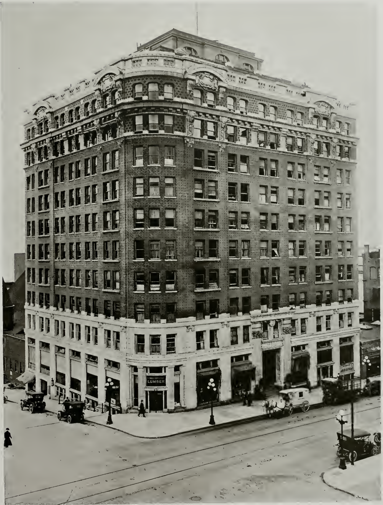
COBB BUILDING, SEATTLE
