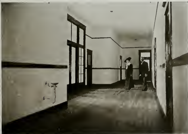
WELL LIGHTED CORRIDOR
