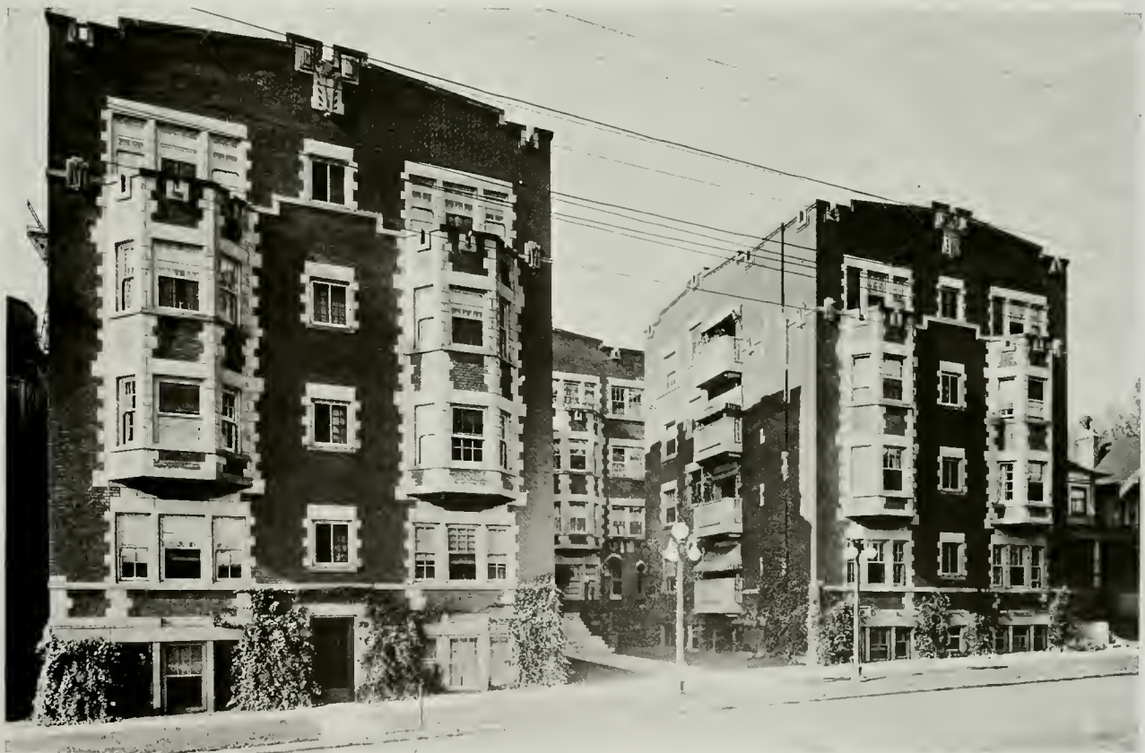
TRINITY PLACE APARTMENTS, PORTLAND ROOT & KERR, ARCHITECTS
