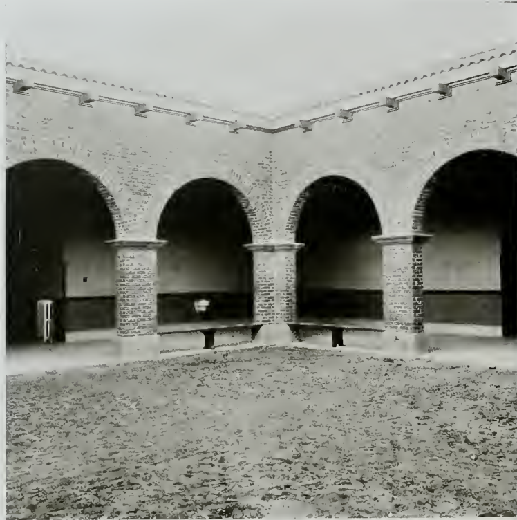
PATIO, DOUGLAS GRADE SCHOOL, DOUGLAS, ARIZONA
