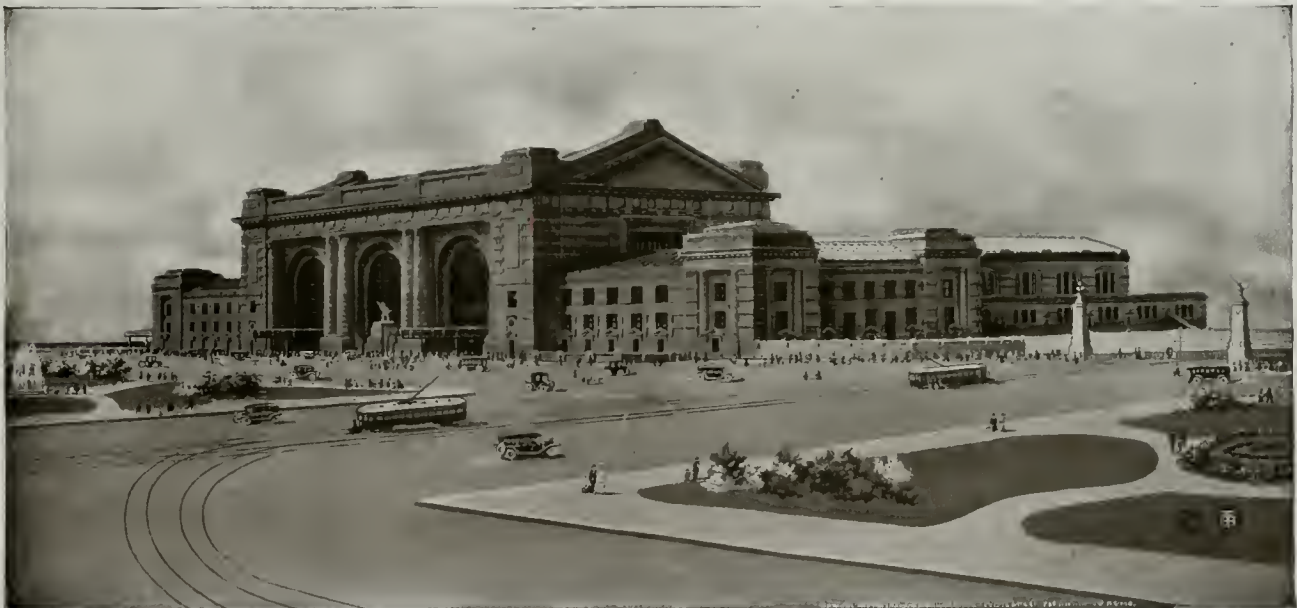
Creosoted Wood Block Pavement Laid Around Kansas City's New Union Station.
