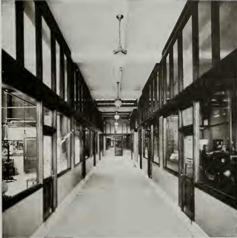
ARCADE IN WHITE BUILDING, SEATTLE Howells and Stokes, Architects, A. H. Albertson, Associate Shows one stretch of the arcade and public corridor in the ground floor running from one street front to the other through the space at the rear of the elevators for the purpose of enhancing the value of the space.
