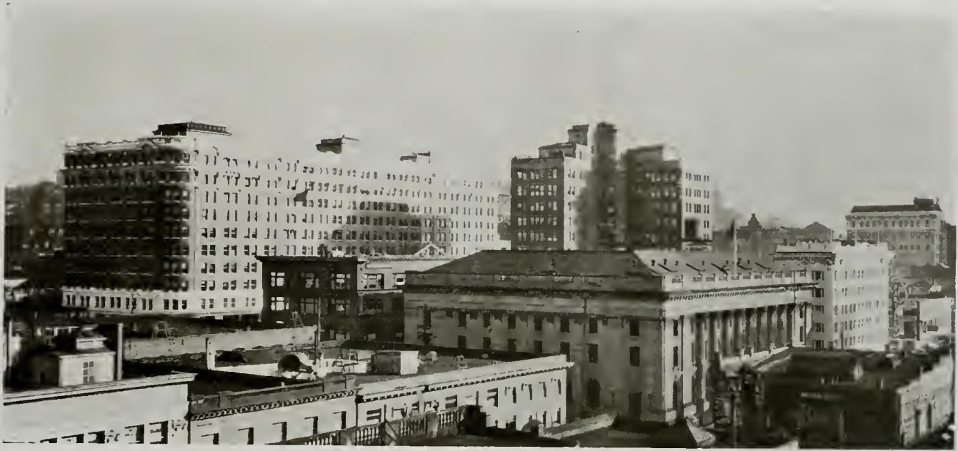
GENERAL VIEW OF THE WHITE-HENRY-STUART BUILDING AND THE COBB BUILDING, SEATTLE Howells and Stokes, Architects, A. H. Albertson, Associate
