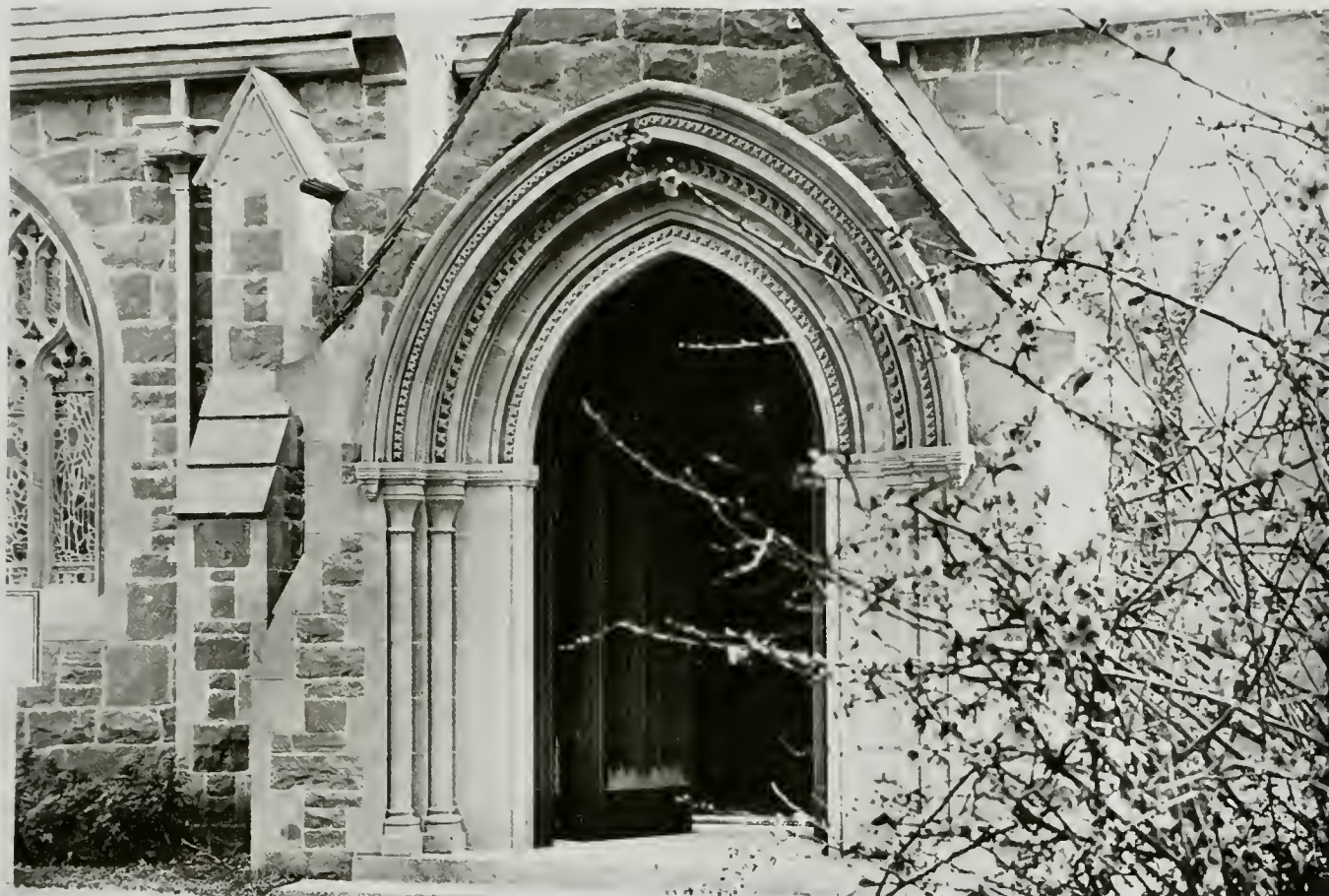
DETAIL OF ENTRANCE
