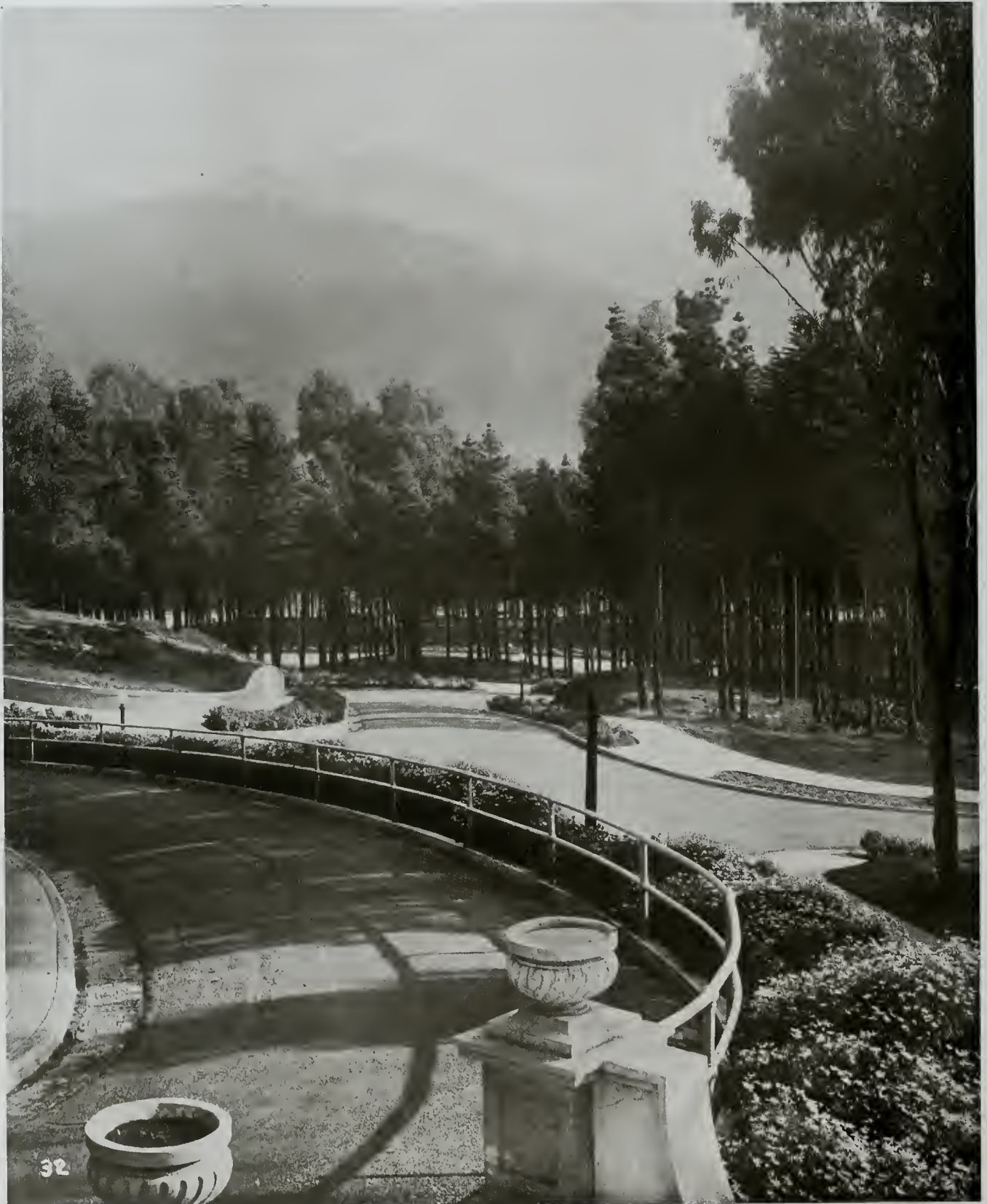
AN EFFECTIVE PIECE OF ENGINEERING IN DESIGN OF STREETS, FOREST HILL SAN FRANCISCO MARK DANIELS, ENGINEER
