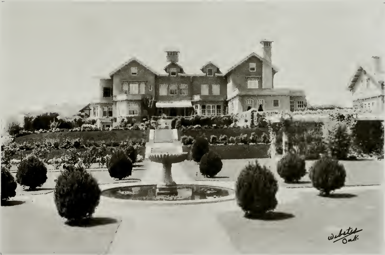
HOME OF MRS. S. T. ALEXANDER, PIEDMONT, CAL. C. W. DICKEY, ARCHITECT
