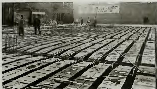
STEELFORMS READY FOR CONCRETE
