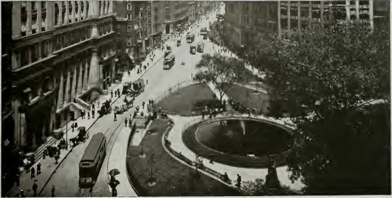
Broadway, New York, Paved with Creosoted Wood Block. This quiet form of pavement has increased office values on America's Best Known Street.
