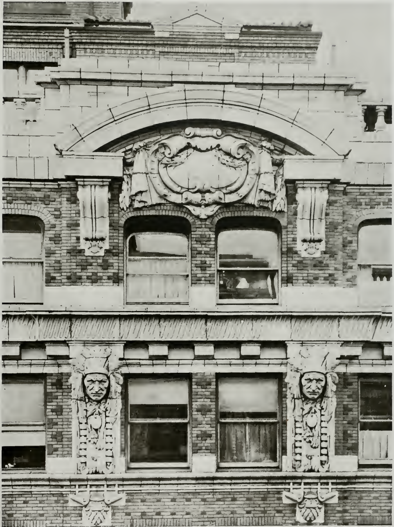
DETAIL OF UPPER STORIES OF COBB BUILDING, SEATTLE Howells and Stokes, Architects, A. H. Albertson, Associate
