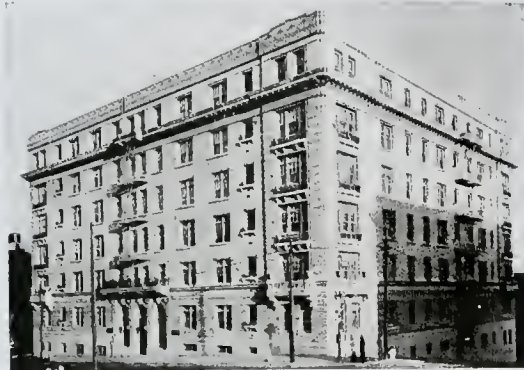
WARRINGTON APARTMENTS — FREDERICK H. MEYER S. E. Cor. Post and Leavenworth Sts., S. F. Architect
