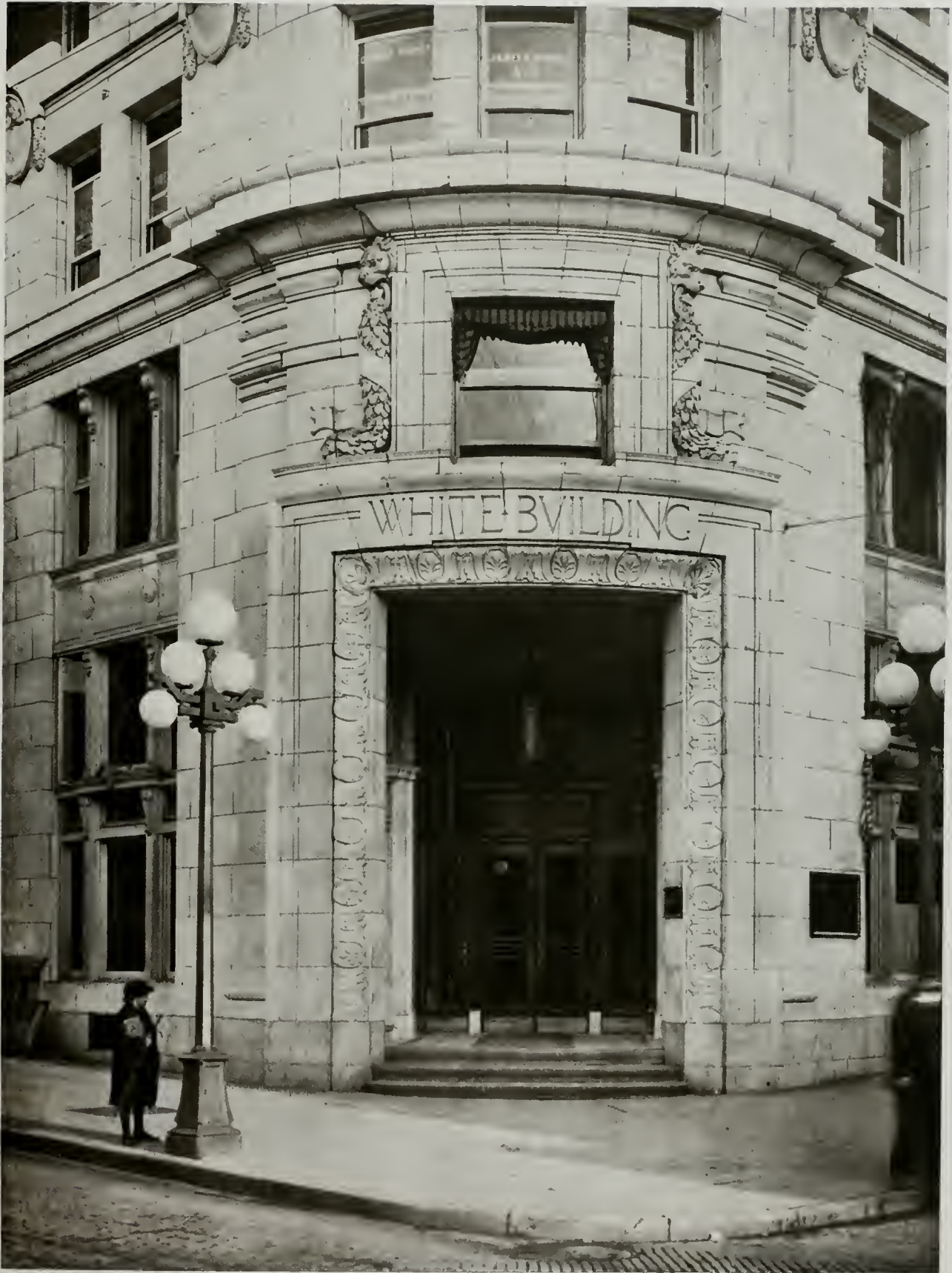
ENTRANCE DETAIL OF WHITE BUILDING, SEATTLE Howells and Stokes, Architects, A. H. Albertson, Associate
