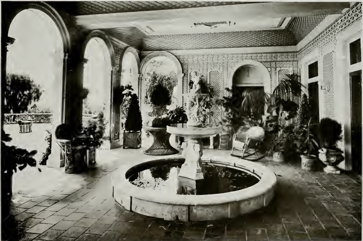
COURT AND FOUNTAIN HOUSE OF DAN MURPHY, LOS ANGELES HUDSON & MUNSSELL, ARCHITECTS
