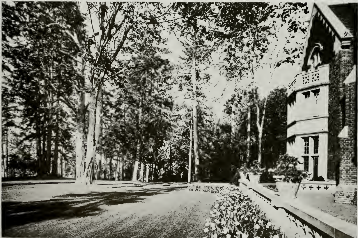
WOODED PARK AND LAWN THORNEWOOD, COUNTRY HOME OF CHESTER THORNE, TACOMA CUTTER & MALMGREN, ARCHITECTS, SPOKANE
