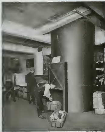
Inlet to closed type conveyor at one of the stock floors.
