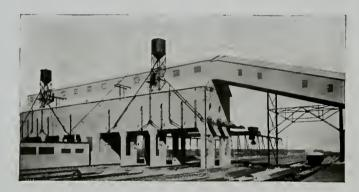
Ambler Corrugated Asbestos Roofing and Siding as Applied to Coal Pockets of the Central Rallroad of N. J., at Communipaw
