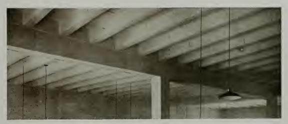
Open Ceiling Construction Resulting from use of Meyer System Metal Forms.
