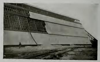
Corrugated Asbestos Roofing and Siding Being Applied to Phosphate Rock Storags Bin of the American Agricultural Chemical Co.,
