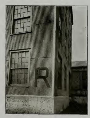
Ambler Corrugated Asbestos Used as Siding with Ambler Flat Asbestos Bulding Lumber for Framing, and Asbestos Ridgs Roll on Corners. Neighboring Building Covered with Century Asbestos Shingles
