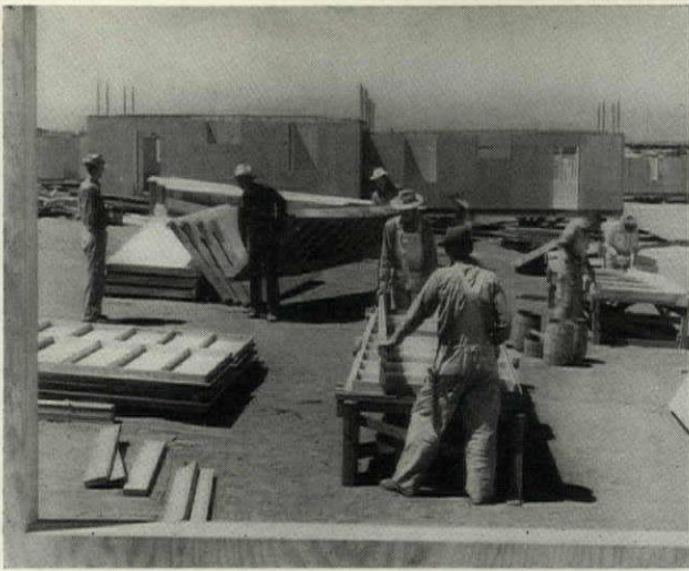
Prefabricated house construction—whose value many question—is about the most we have found practicable in plywood, but—
