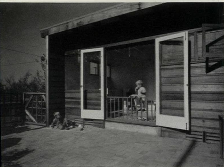
Mrs. McCormack laid the brick paving and built the barricade to the children's room herself.
