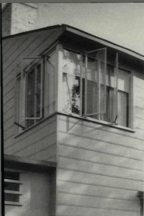
Steel sash open up a corner
