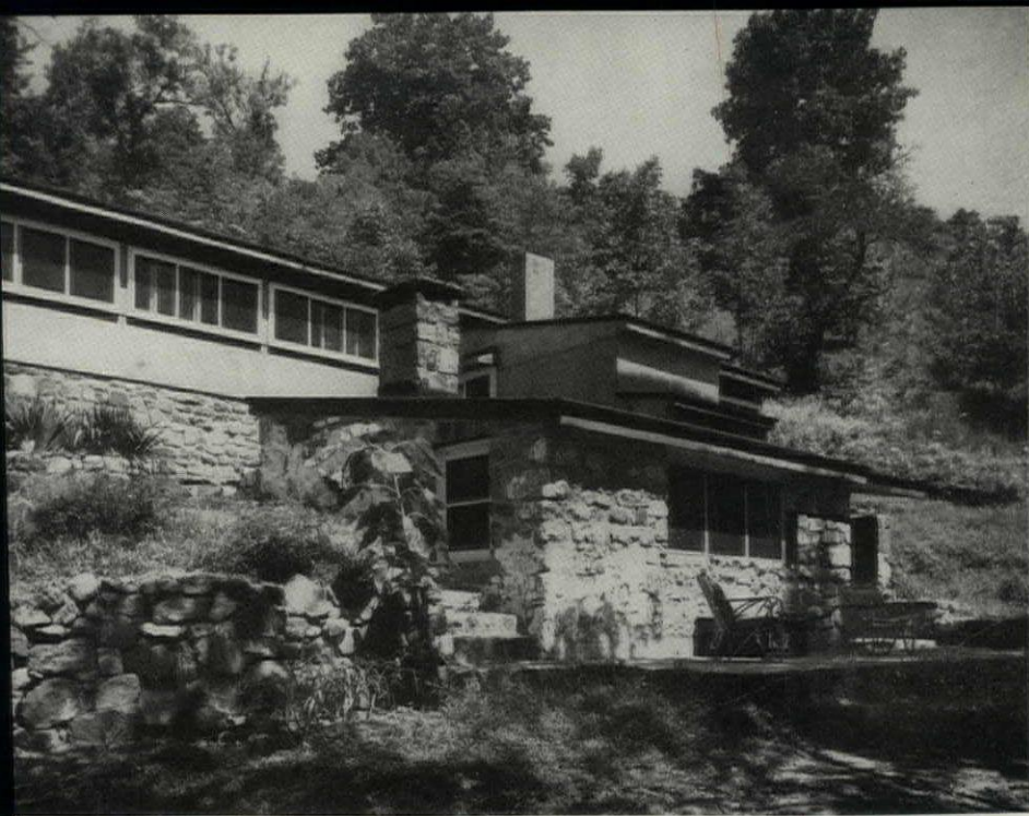
Masonry from an old house built the walls of the first level.
