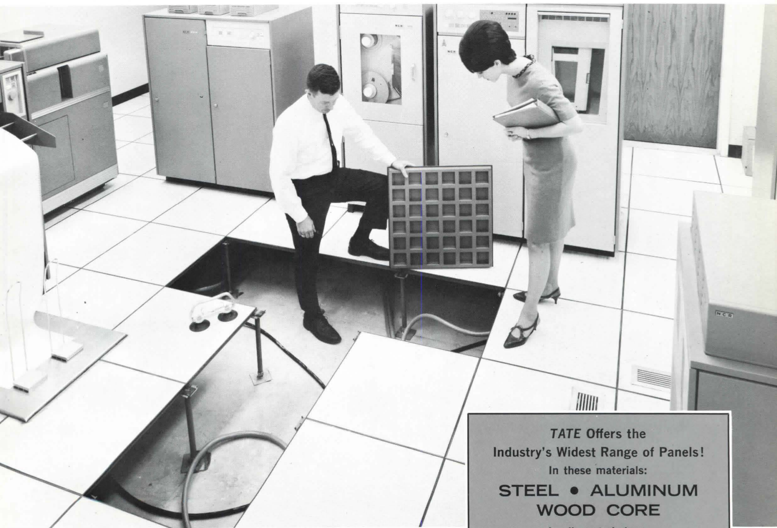
The Computer Center, Koppers Company, Inc., Baltimore, Md.
