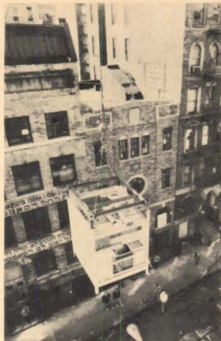
Preassembled kitchen-bathroom core unit being lifted to roof of building.
