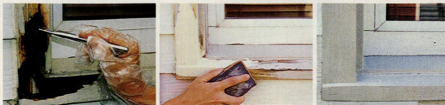
Restoration of rotted window is easy and cost-effective.
