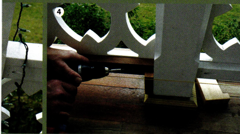
Next, he used pocket screws to securely fasten the railing section to the posts at the top (3) and bottom (4). The finished sections, complete but for some paint and the installation of the ¾" top rail, are ready to weather another 100 years.
