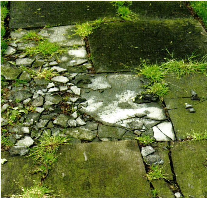
Parts of the walkway were falling to pieces—especially in areas where thin slate flagstones had been used for repairs through the years. Grass poking through joints and cracks was also a problem.
