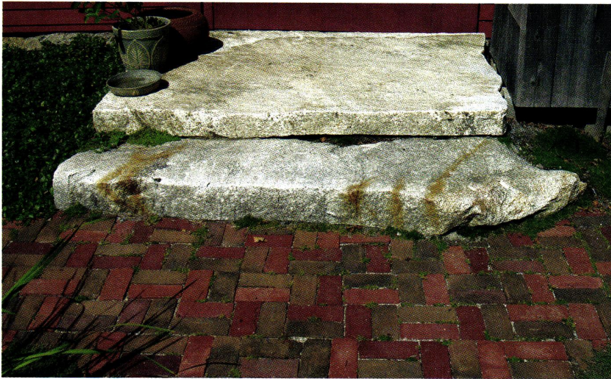
Hefty fieldstones provide a sturdy new stoop, replacing the rickety wooden one.
