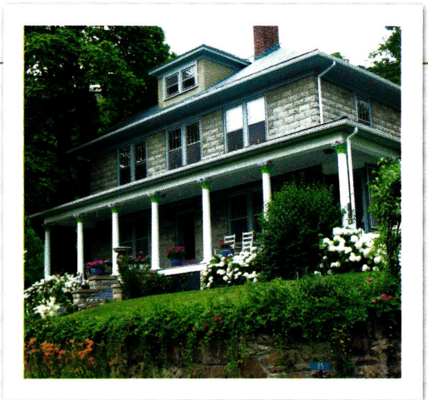
The blocks comprising this Foursquare house are made of concrete fabricated to resemble stone—an early 20th-century fad.
