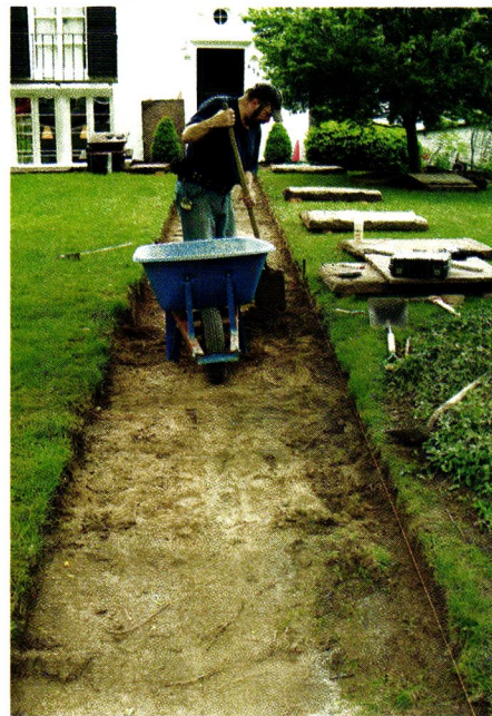
CLOCKWISE FROM TOP: Marty (at left) and Lou carefully removed the heavy original stones. Next, they used shovels to dig out the base, and spread a 5" to 6" layer of crushed dolomite limestone, which was compacted with a plate tamper (in foreground).
