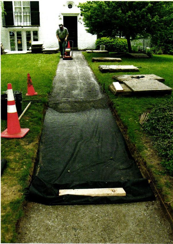
CLOCKWISE FROM ABOVE: To keep vegetation from penetrating the walk, the men laid a length of landscape fabric, which was covered by a layer of stone dust (also compacted). Next, they carefully re-positioned the stones, using a level to ensure their work was square. Finally, Marty used a dry saw to trim rough edges off of replacement stones for a perfect fit.
