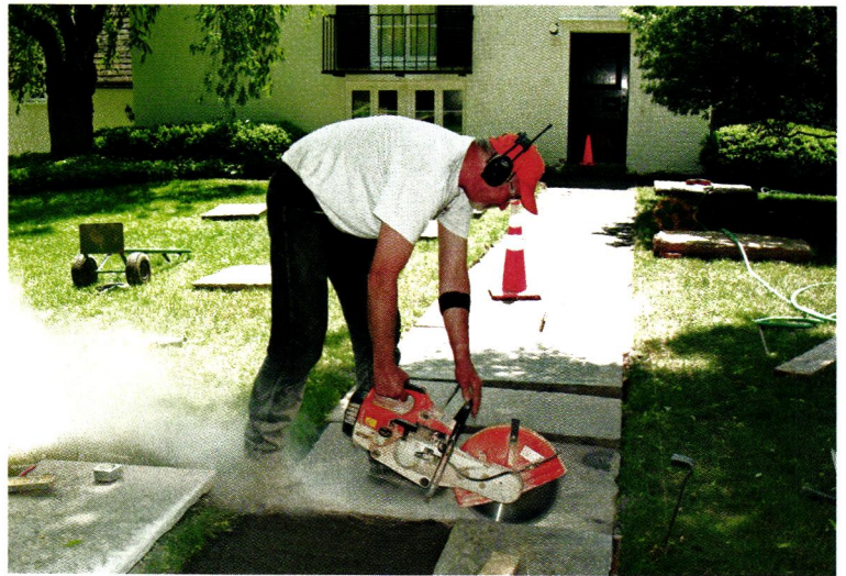
CLOCKWISE FROM ABOVE: To keep vegetation from penetrating the walk, the men laid a length of landscape fabric, which was covered by a layer of stone dust (also compacted). Next, they carefully re-positioned the stones, using a level to ensure their work was square. Finally, Marty used a dry saw to trim rough edges off of replacement stones for a perfect fit.
