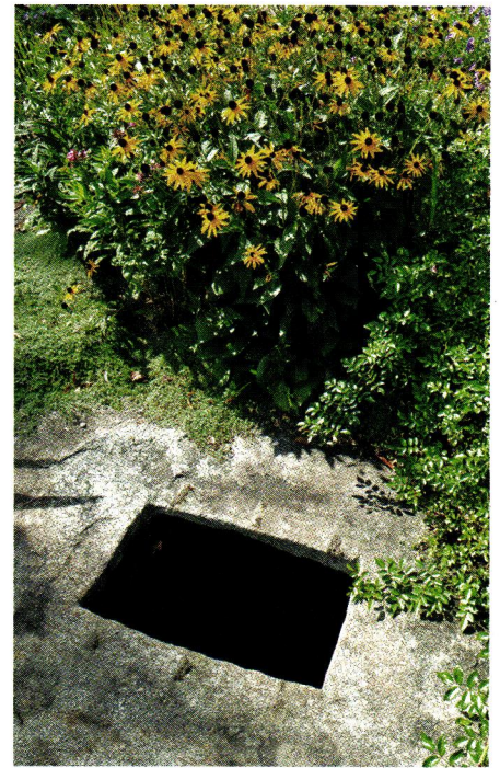
Antique granite surrounds a stone-lined well, which is usually topped with a wooden cover.
