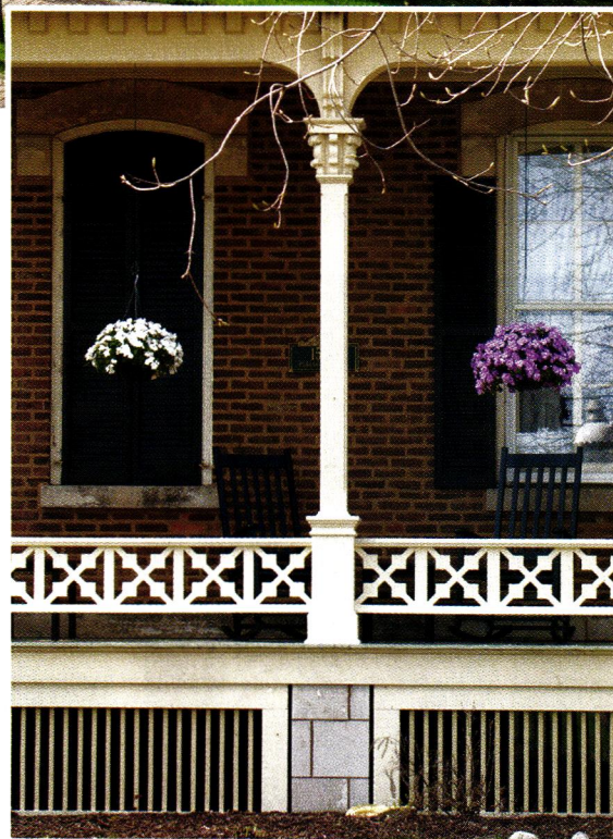
TOP: The new addition (at left) is understated. ABOVE: The porch was completely restored; its snowflake railing was modeled after one found on a similar house. OPPOSITE: The back entrance’s screened porch serves as a passageway for the homeowners’ son, Sam.
