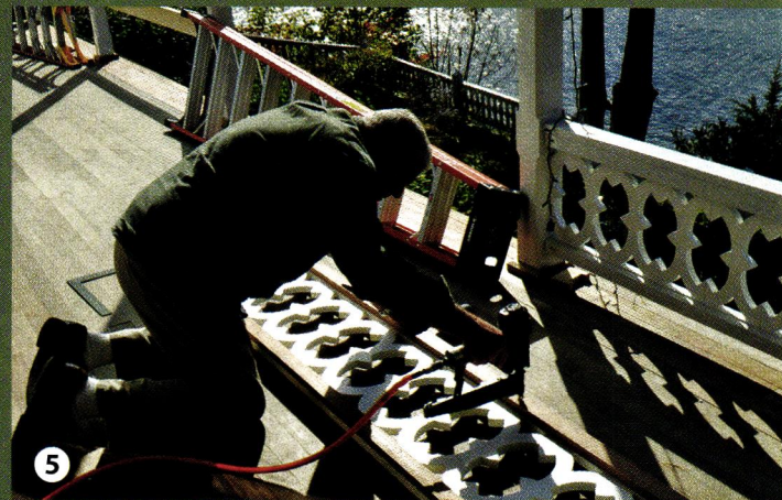
After checking to ensure that everything was squared up (4), Jim began securing individual elements. He drove 2½" galvanized trim nails into the four corners using a pneumatic nail gun, then placed four nails into each baluster piece (5).
