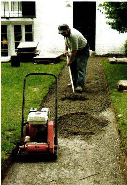
CLOCKWISE FROM TOP: Marty (at left) and Lou carefully removed the heavy original stones. Next, they used shovels to dig out the base, and spread a 5" to 6" layer of crushed dolomite limestone, which was compacted with a plate tamper (in foreground).
