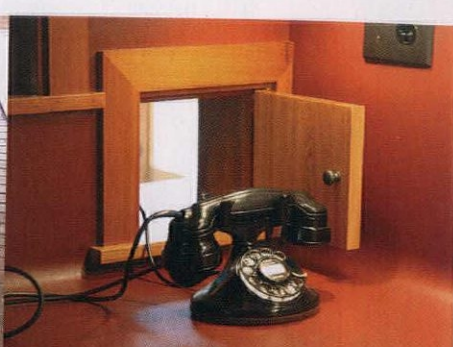
The finished countertop's coved back seamlessly curves up the wall and jogs around a built-in telephone nook.
