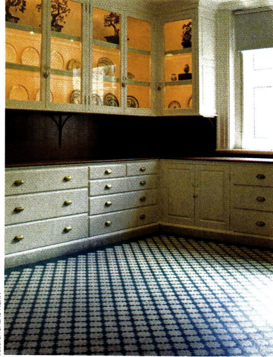
An original rubber kitchen floor in Washington, D.C.'s Anderson House, built in 1905, shows how early tiles fit together like pieces of a puzzle.
