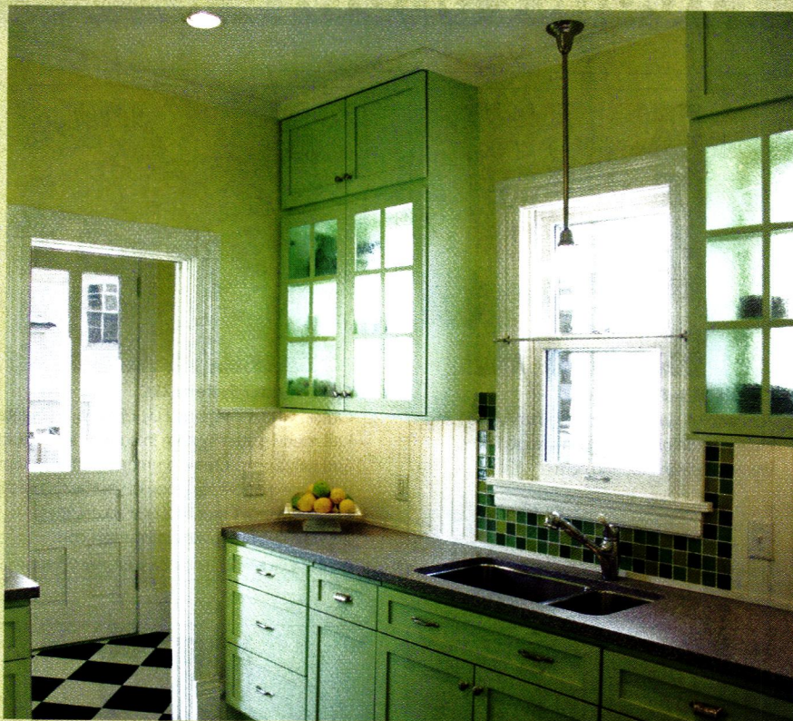
To bring light into the dark kitchen, U+B installed windows—chosen to match the originals as closely as possible from the outside-the-house view—behind the kitchen cabinets.
