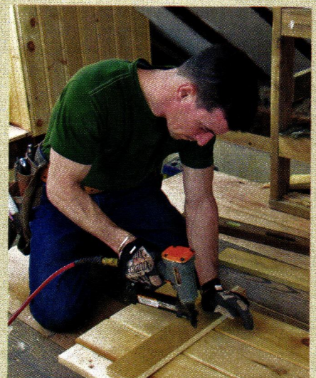
Fasten the rail onto the first board using 1/4" narrow crown staples, then weave subsequent boards in, fastening as you go.
