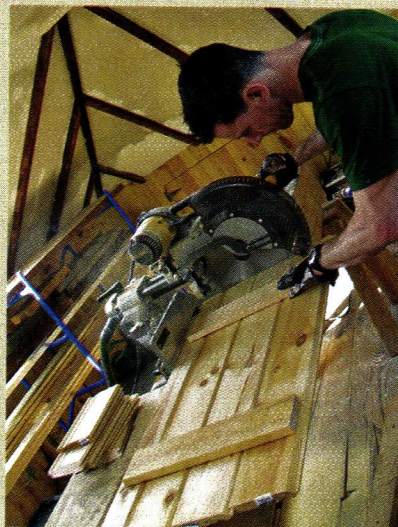
Take the blank to the slide compound miter saw and square cut one end. Then measure for finished height and cut the other end.
