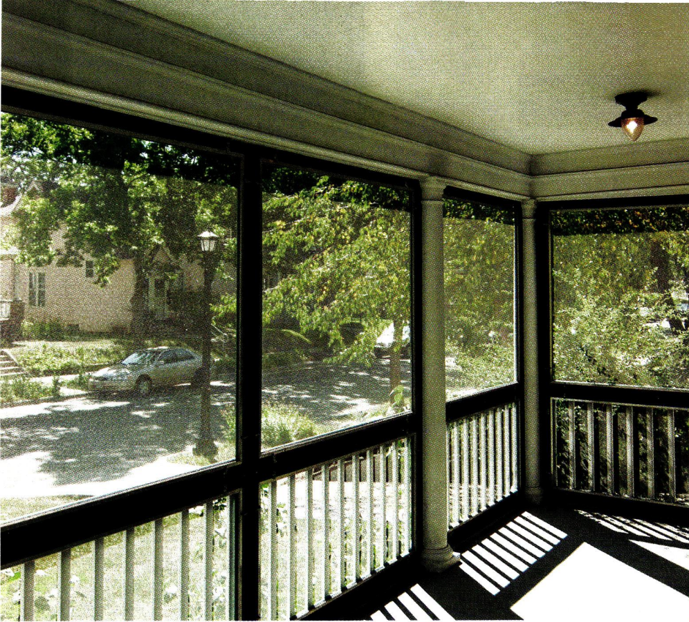
The U+B team designed a screening system that fits inside the original porch rails, creating a space where the couple can eat outside, "without being attacked by Minnesota mosquitoes," jokes Marlee.
