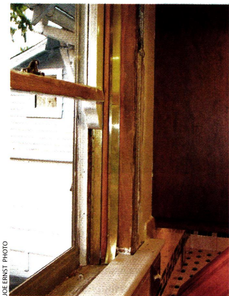
LEFT: Weatherstripping helps keep winter weather at bay on even the coldest days. ABOVE: The brass flange installed here is one of many ways to tighten up drafty areas around windows.
