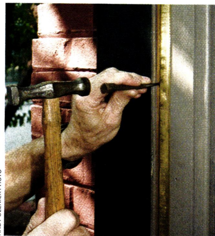
Brass channel strips are easily nailed into place—be sure to use brass- or copper-plated brads to prevent galvanic corrosion.
