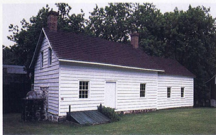
Flared eaves on the plain gable roof of the Kruser-Finley house, 1790, now at Richmondtown Restoration, Staten Island, N.Y.
