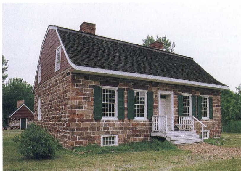
A brownstone Dutch Colonial with gambrel, flared eaves, and clapboards in the gable, built in New Milford, N.J., ca. 1774.
