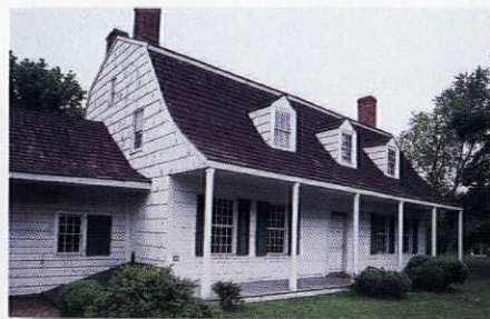
Flared eaves project outward to form a porch on this 1740 New Dorp, N.Y. house, now at Richmondtown Restorations.
