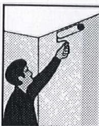
2. Apply saturant to area to be covered.
