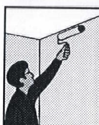
7. Apply second coat of saturant to wet mat.
