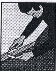
5. Trim mat at baseboard and window.
