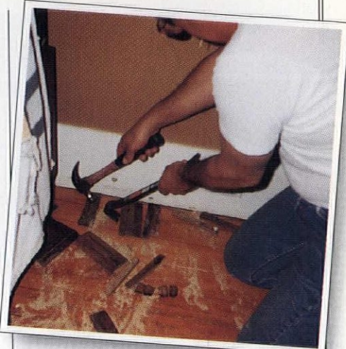
The last of the parquet put us past the point of no return, with plenty of glue to go.
