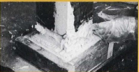
...were completely sawed off and replaced with...
