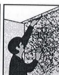
4. Trim excess mat where wall meets ceiling.
