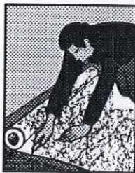
1. Cut fiberglass mat 2" longer than height.
