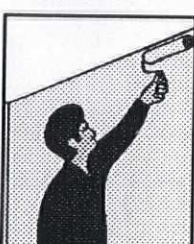
12. Apply 2nd coat of saturant (include seam)
