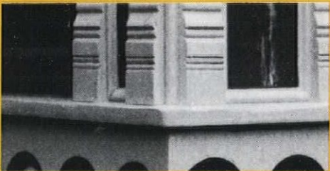
...sanded, nailed, stained or painted.
