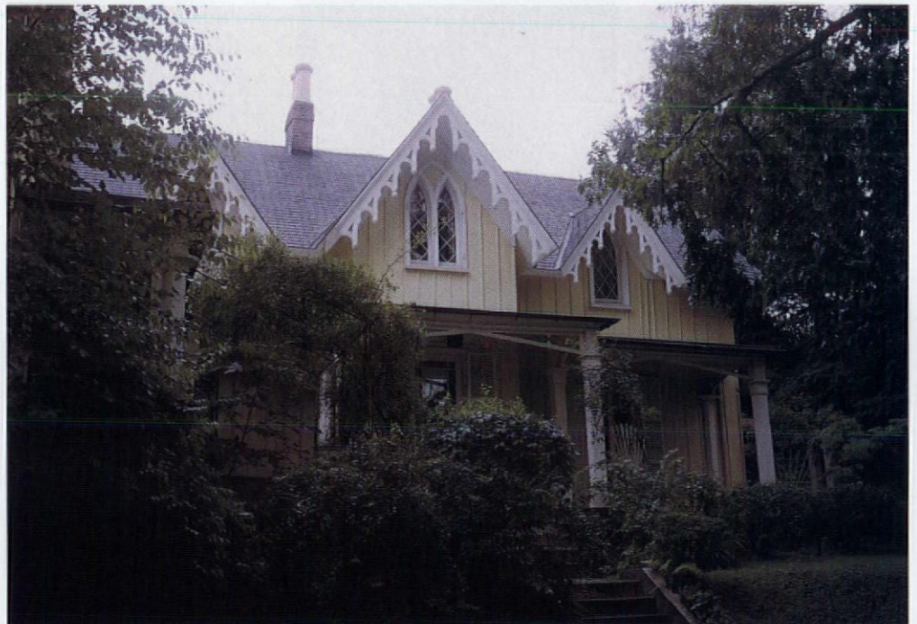
Vergeboard (or bargeboard) decorates Gothic gables. This example, from A. J. Downing's Cottage Residences has a kingpost with pendant and finial.
