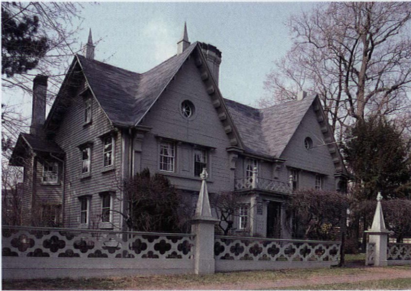
ABOVE: The extraordinary fence, with its quatrefoils and crocketed finials, was added to the Salem, Massachusetts, Pickering House when it was Gothicized in 1841, almost 200 years after construction. RIGHT: New York's Jasper Cropsey House and Studio (c. 1840) has an "organic" rural setting, popular for the style.
