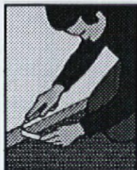
5. Trim mat at baseboard and window.
