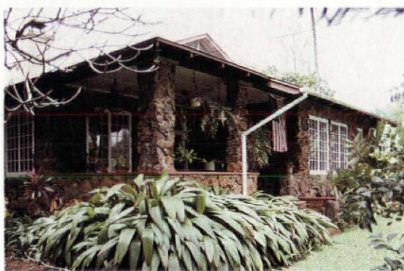
The lava rock walls of the 1930 Head Bookkeeper's house were a product of Kauai's volcanic environment.
