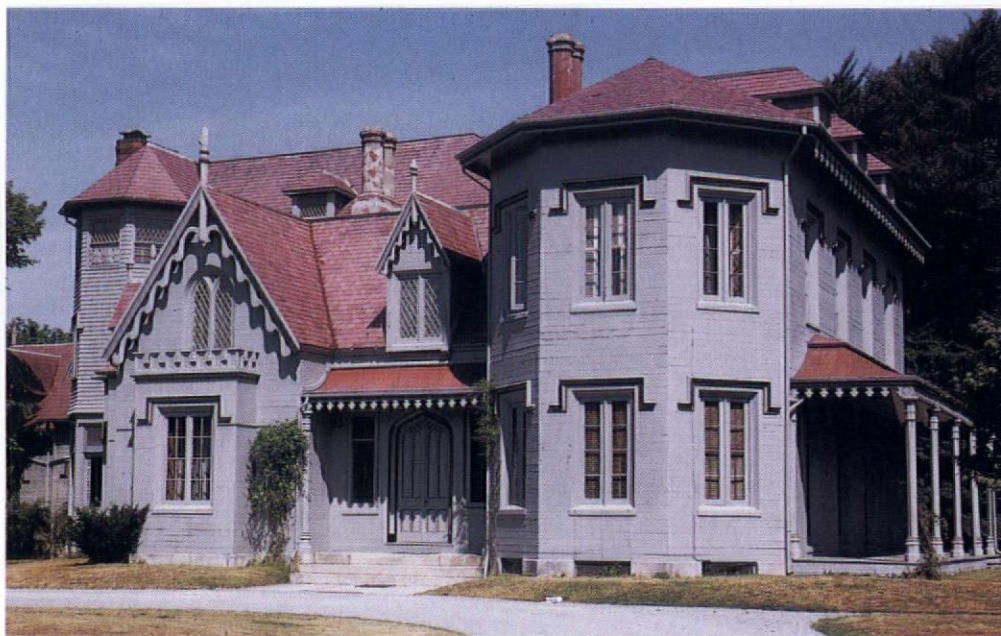
LEFT: Rich with Gothic ornament, this Rhode Island mansion has dripping pendants, diamond-paned casement windows, lancet arches, hood molds, clustered columns, and a crenellated parapet around the bay window. CENTER: A tiny house with four arched openings and a miniscule balcony is on the other end of the revival's spectrum — small, rural cottages.
