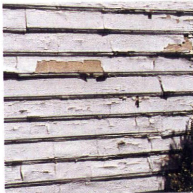
Peeling down to bare wood
