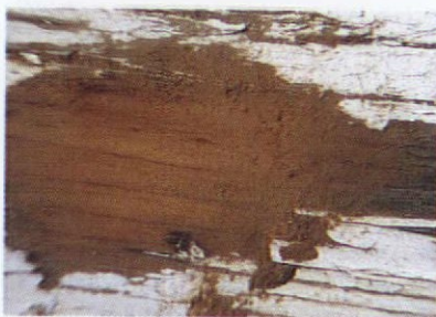
Sand weathered areas until “bright” wood shows.
