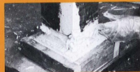
...were completely sawed off and replaced with...
