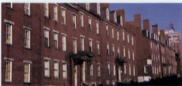
Manchester, N.H., c. 1890: Despite differences in size and elaboration, row houses varied remarkably little as they were built over the centuries, for different social classes, and in far-flung cities. This row was built as mill-worker housing.
