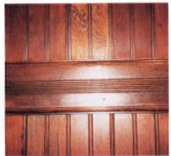
Heavily beaded and uniformly milled wall panelling in an 1890 railroad station.
