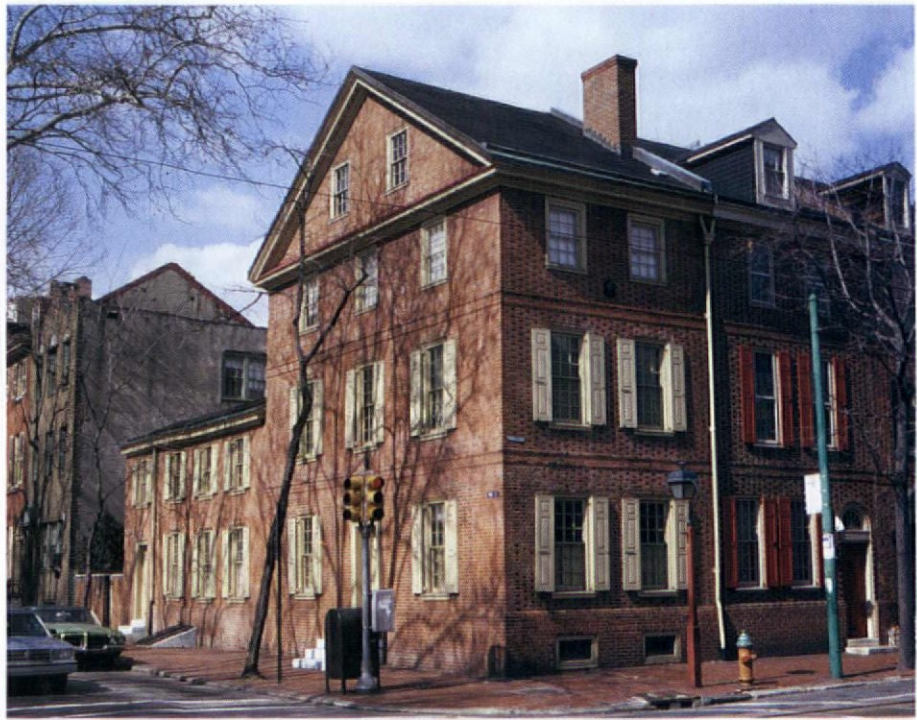
Philadelphia, 18th century: Corner houses offered options in floorplan, with more light and air. The entry could be moved to the long side, too, providing a gracious center hall. A cornice return creates a neat pediment.
