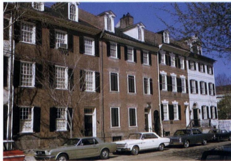
Alexandria, Virginia, late 18th century: brick houses in the Federal or Adam style, each three storeys tall and three bays wide. Note the projection of the firewell well above the roofline.
