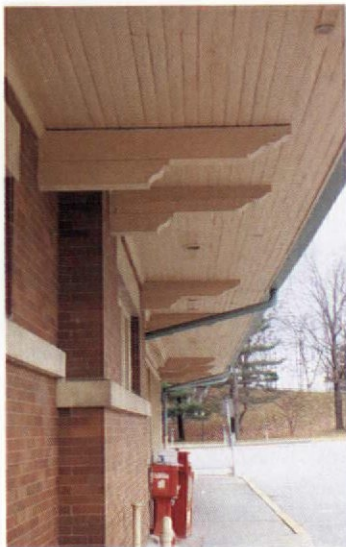
Simple edge-matched beaded boards were a common soffit finish, indoors and out, by the turn of the century.
