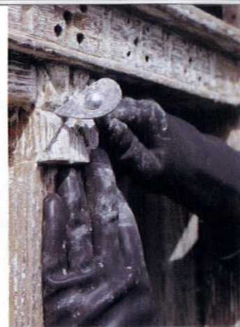
Shaped scrapers pick away softened paint without damaging the wood carvings.
