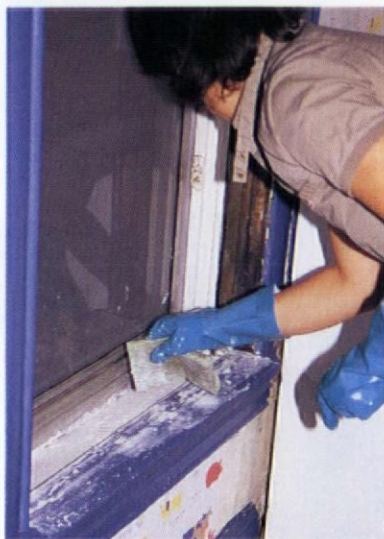
Patching compound, used to cover chipped paint, can be smoothed with a sponge to avoid dry-sanding.
