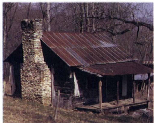
(left) Spanish-style metal tile. (right) Corrugated metal roofing on a North Carolina homestead.
