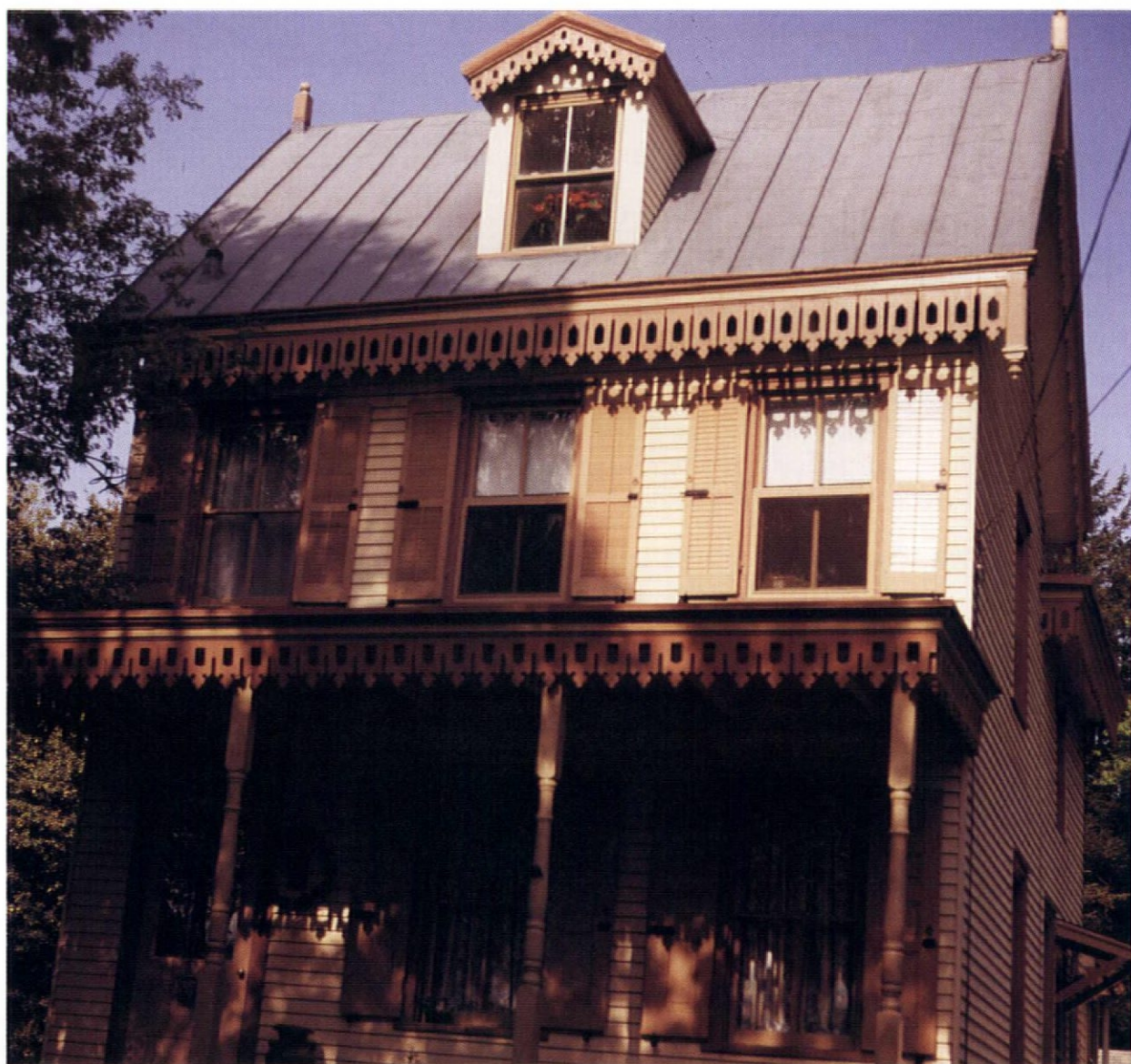
The ubiquitous standing-seam roof (above), here in Haddonfield, N.J. Two styles of decorative metal shingles (left): Gothic and hexagonal.
