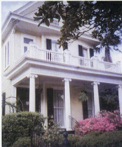
Candidate for lead abatement? In New Orleans, 60 to 70 percent of the housing contains lead paint — a hazard even in affluent areas, as it is in deteriorated housing.
