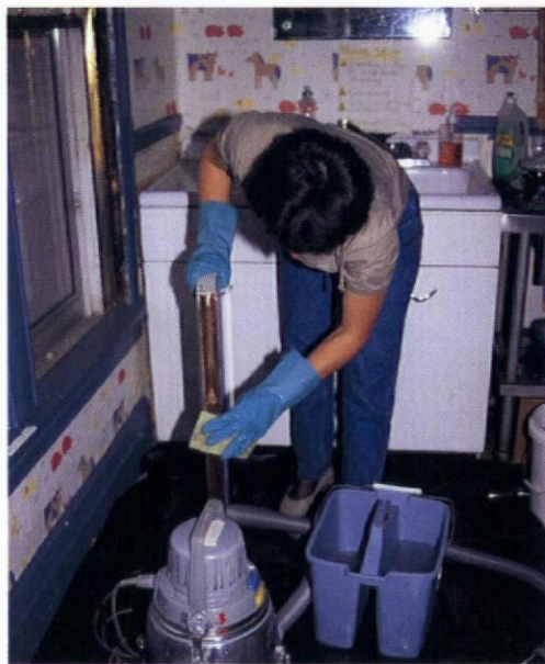
Low-tech but effective: Alternate washing and vacuuming until most of the loose paint chips and dust are gone.
