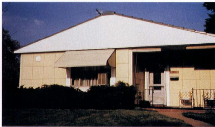
In Brookfield, Illinois, the roof, walls (interior and exterior), and ceilings of this prefabricated Lustron house are made of porcelain enamel-finished steel panels.
