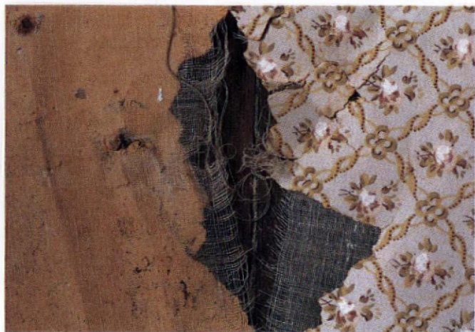
If the old wallpaper pulls off relatively easy, it's likely you'll find netting such as this adhered to the back.
