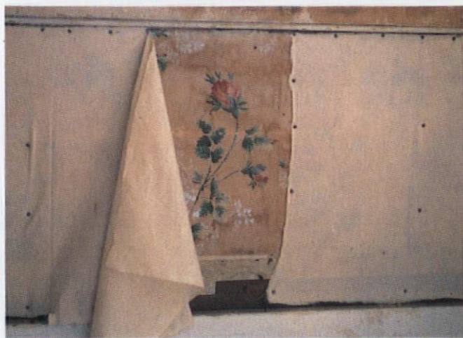
If you want to provide a record for curious historians and restorers of a future time, you can place new netting over smooth, secure remnants of old paper.
