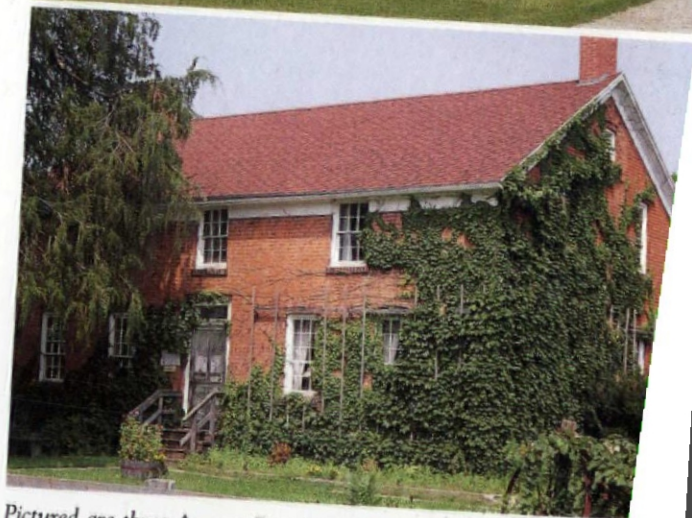
Pictured are three Amana Four-Family houses constructed of different materials: coursed-rubble stone (top), wood frame with cement (middle), and brick (bottom). The early floor plan of an Amana Family (top right) did not include a kitchen, which was in a separate communal building shared by approximately 20 families.
