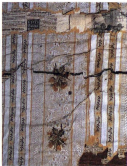
Newspaper was often used as an underlining for wallpaper but provided little protection for the paper as boards expanded and contracted.
