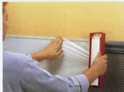
Tape n' Drape is a disposable dropcloth which makes cleanup easier.
