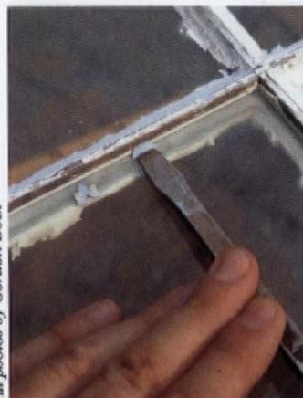
Top: The tiny wheel on a glass cutter (at left) does the scoring. Left: triangle points (being set) and push points. Right: "running down" putty for a finished bevel.
