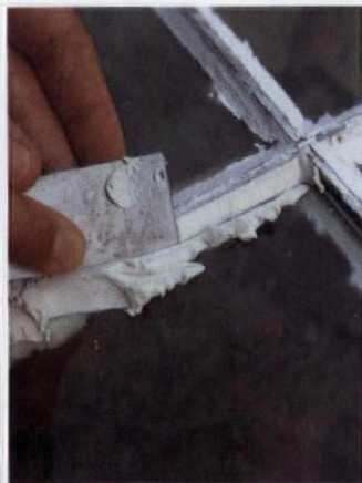
Top: The tiny wheel on a glass cutter (at left) does the scoring. Left: triangle points (being set) and push points. Right: "running down" putty for a finished bevel.
