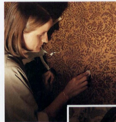
Top: A fiberglass screen serves to protect old wallpaper during the vacuum-cleaning process. Above: After repasting a wallpaper section, excess paste may be dabbed off with a white cotton ball. Right: discrete areas of lost or flaking paint being inpainted.
