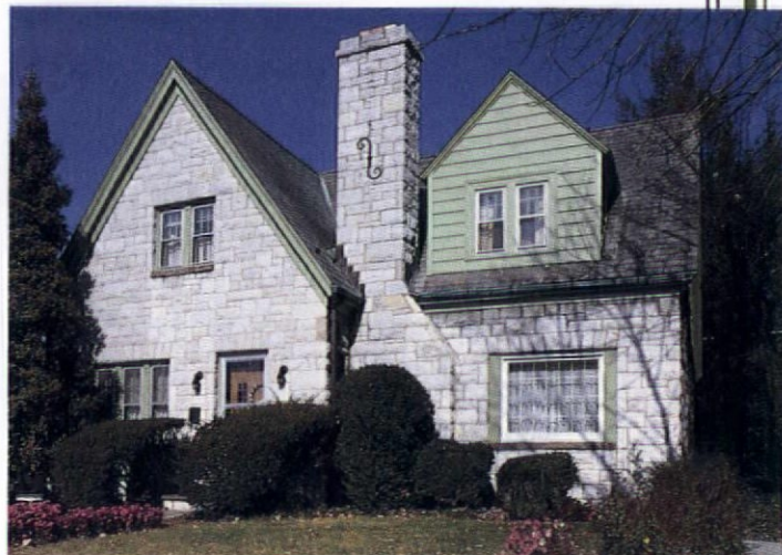
Large clapboarded dormers, such as the one on this Winchester, Virginia, house, made useful additions to steep-roofed buildings.
