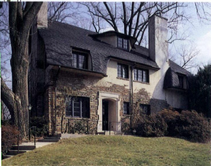
On this picturesque Washington, D.C., home, shingles are manipulated to suggest a thatched roof, and stone walls are exposed below artfully distressed stucco.
