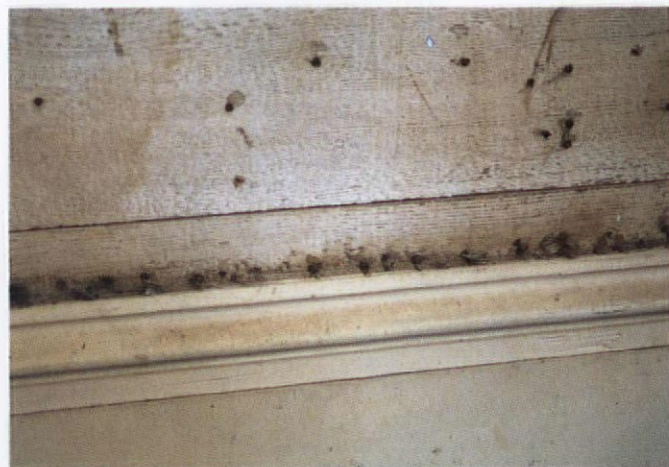
Heavy tack build-up, common at baseboards and ceilings, should be thinned to allow space for new tacks.
