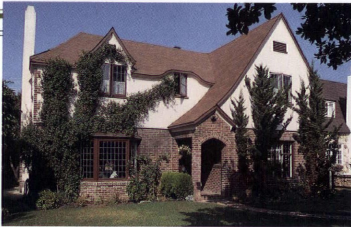
Leaded casement windows and a Tudor arched entryway at the base of a catslide roof make this Coronado, Calif., house English Revival.
