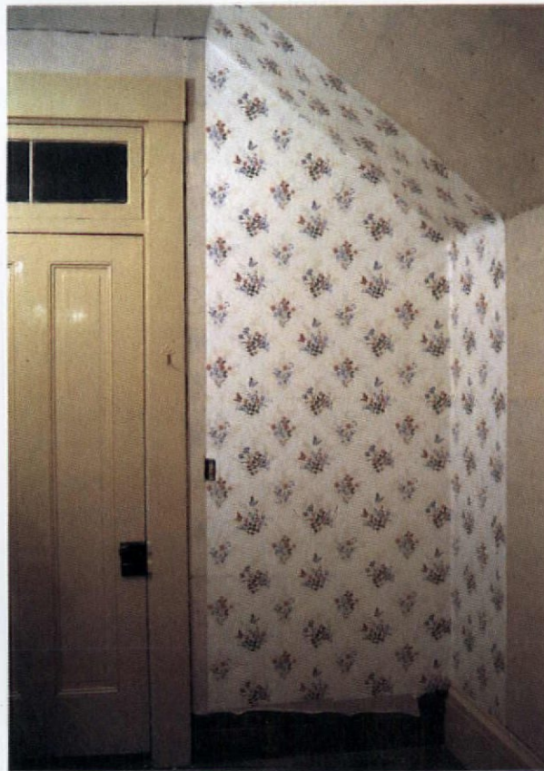
After having been well tacked and shrunk taut with a light application of water, the netting received its new paper, and both are now ready for a long life.
