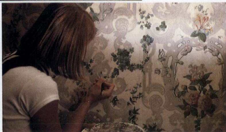
Top: A fiberglass screen serves to protect old wallpaper during the vacuum-cleaning process. Above: After repasting a wallpaper section, excess paste may be dabbed off with a white cotton ball. Right: discrete areas of lost or flaking paint being inpainted.
