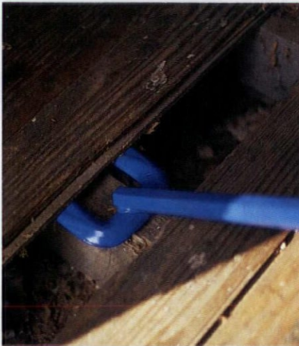
A stripping bar in action.
