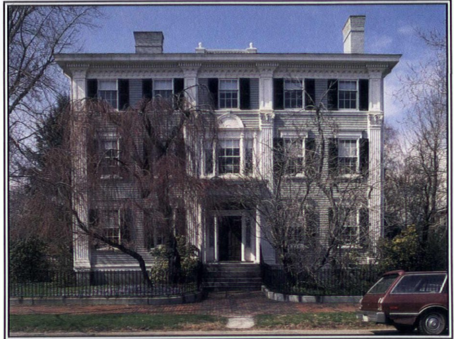
An example of an archeological approach to Colonial Revival is this 1905 house in Ryton, Clark County, Va., top. However, the presence of the covered entry porch and the two side wings are obvious modern elements. Notice the dentil moulding on the cornice and the Palladian window on the attic storey at the gable end. At bottom is the Wheatland-Phillips House in Salem, Mass., built in 1896 (John P. Benson, architect).
