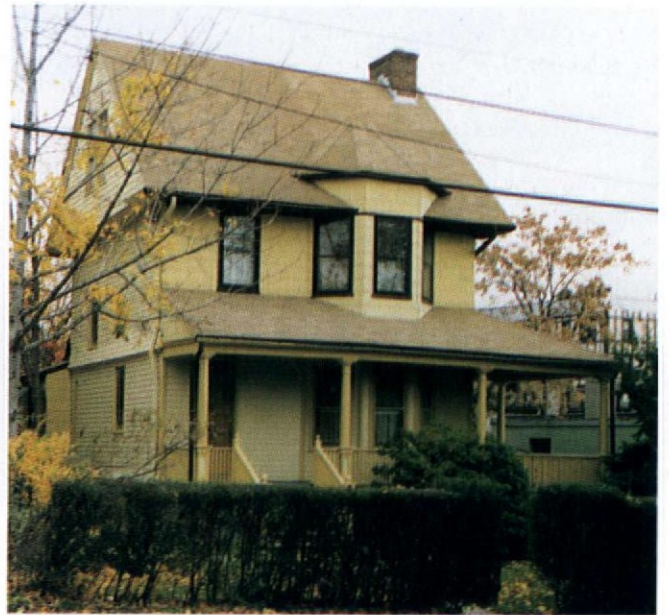
The house as it looks now. We still have to remove the second-floor shingles.
