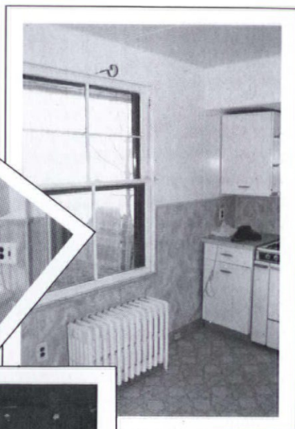
"Old" wall and floor coverings, above.
