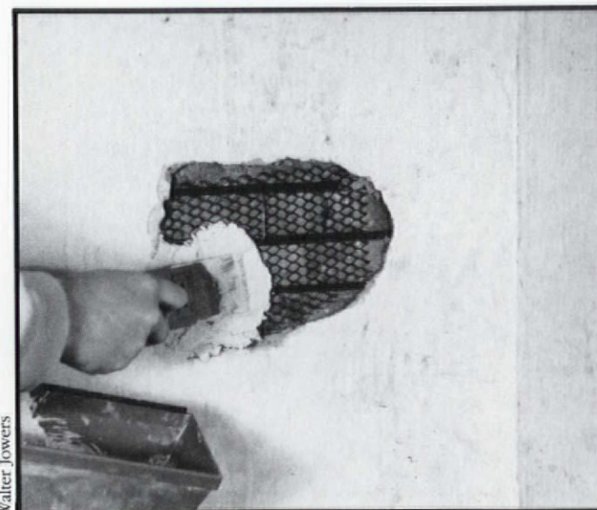
Metal lath has been tied over wood lath to provide reliable keying of the patch plaster.
