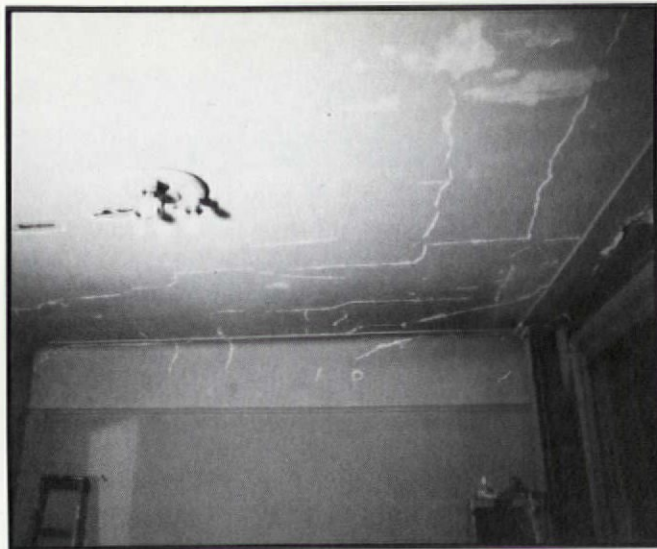
Patching cracks is time-consuming ...
