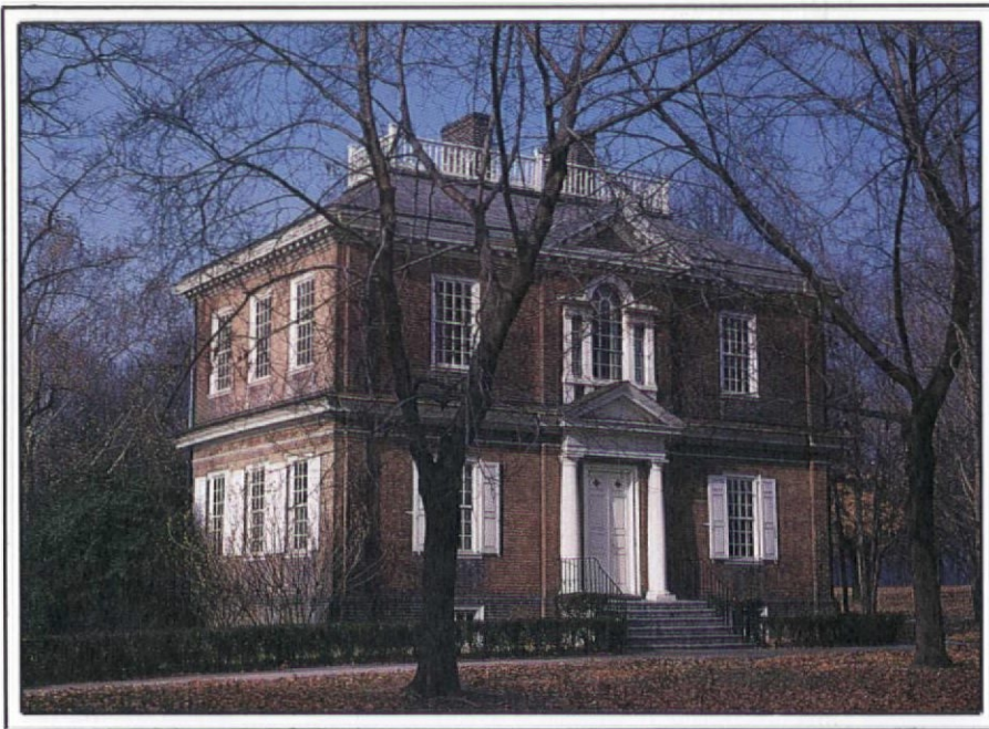
left: Woodford (1756; 1772), Fairmount Park, Philadelphia, Pennsylvania. Originally only one storey high, this compact free-standing Georgian was raised to two storeys. Note the Palladian window.
