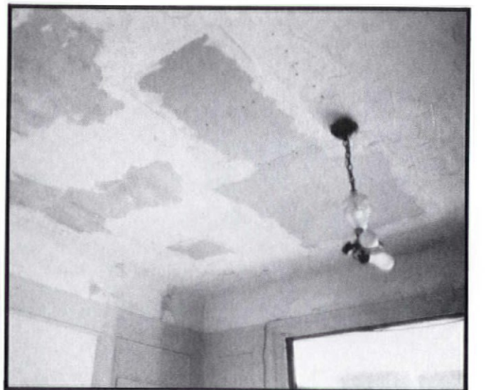
When large chunks of plaster are missing, drywall patches can be used as a base.
