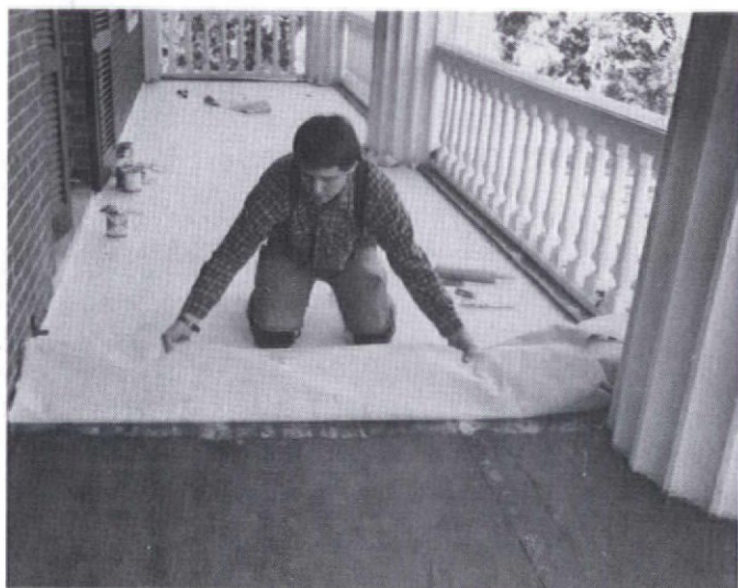
John pulls the canvas back to expose wet adhesive before he proceeds to the next work area.
