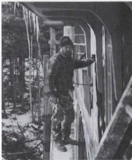
Jim Beyor: (re)building Kragysyde
