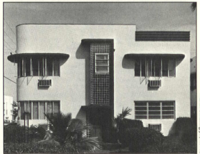
Metal windows helped define the new architecture: here, steel casements in the Miami Beach Art Deco district.
