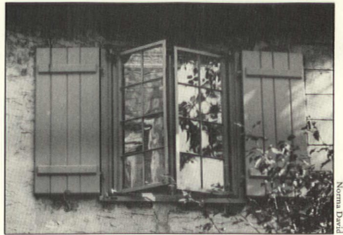
Cottage architecture in the 1920s: stucco walls, batted shutters, and metal casements.
