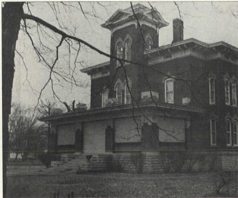
Above: The porch is marked as a later addition by its materials — concrete block and concrete columns. Below: The addition is out of character in proportion as well as in architectural precedent.
