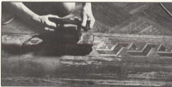
Above: Careful work with a belt sander removes deep scratches. Below: New finish is applied over existing one with a sponge mop. The floor retains its patina while gaining luster.
