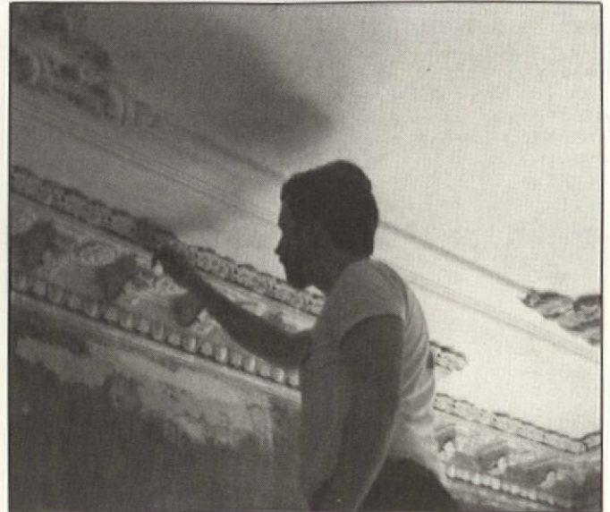
Top left: The work begins. Top right: Dental pick in hand, Greg removes paint from ornate plaster instead of cooking dinner. Bottom left: Atop makeshift scaffolding, Greg applies a new coat of paint.
