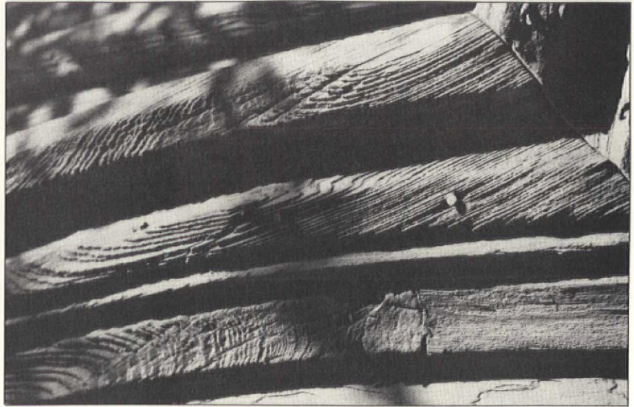
. . . until you get close. Sandblasting left behind wood that has in effect undergone accelerated weathering. Experts believe that pitted, roughened wood like this will deteriorate much more rapidly than normal.
