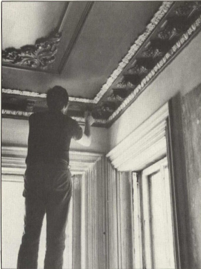
Top left: The work begins. Top right: Dental pick in hand, Greg removes paint from ornate plaster instead of cooking dinner. Bottom left: Atop makeshift scaffolding, Greg applies a new coat of paint.
