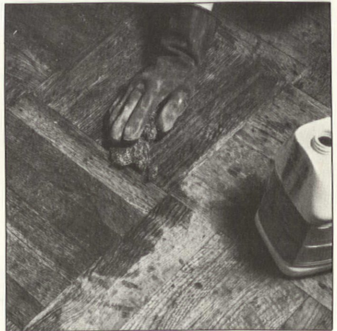
A thorough scrubbing with steel wool and mineral spirits removes all traces of wax and grease. Return to stubborn stains with coarse steel wool and more mineral spirits.
