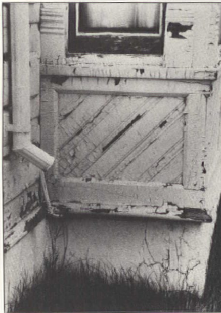
Crazed, alligatored, and blistering paint.
