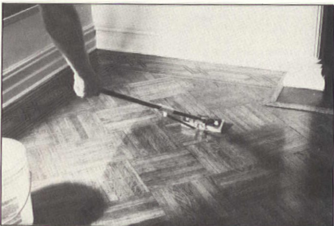
Above: Careful work with a belt sander removes deep scratches. Below: New finish is applied over existing one with a sponge mop. The floor retains its patina while gaining luster.
