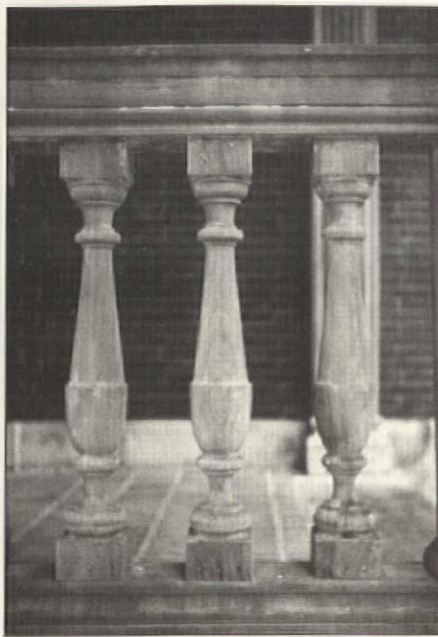
Stripping with chemicals removed the paint without damage.
