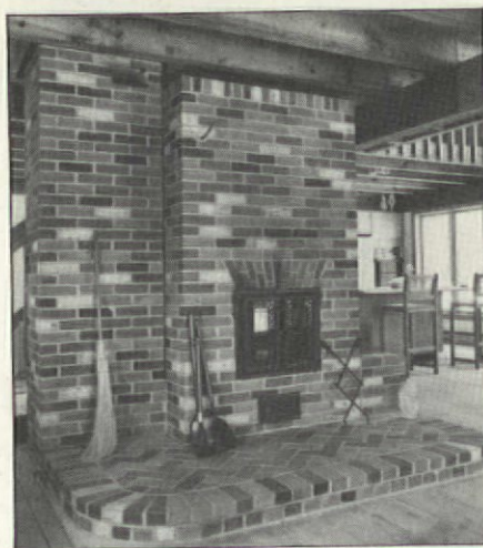
Completed Finnish style fireplace with jack arch and cast iron doors.
