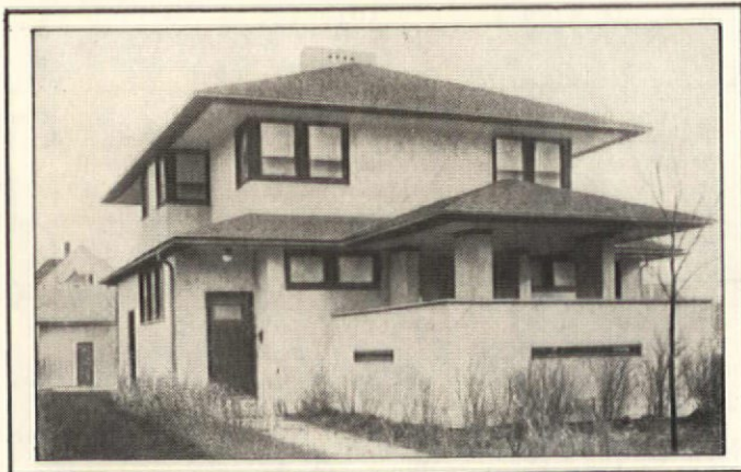
Emphasis on the horizontal line distinguishes houses influenced by the Prairie Style. Broad cantilevered roofs with flat eaves, solid walls with horizontal openings, and windows set in wide horizontal bands all heighten the effect. Stucco or Roman brick were favorite materials. In this example, the porch columns are much thicker than pure engineering would require, adding a note of solidity to the structure.
