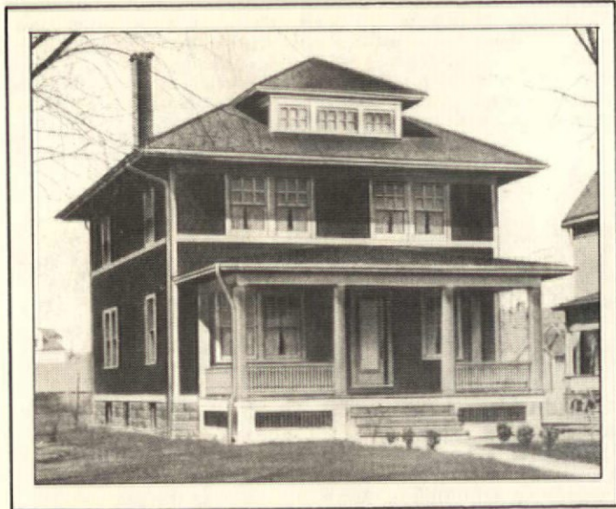
Combining simplicity, economy and versatility, the American Foursquare was one of the most popular house styles in the early 20th century. It's characterized by a two-storey boxlike shape, topped by a low hipped roof. There is usually a dormer in the front portion of the roof, and a porch extending across the full front of the house.
