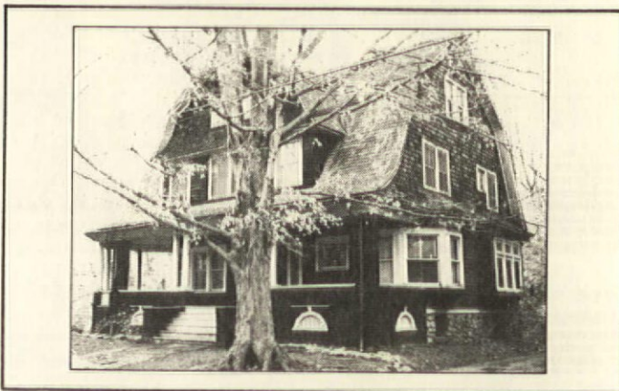
The Dutch Colonial's most recognizable feature is the gambrel roof, which has been used here both for the main roof and for the front dormer. Wood shingles were a favored material for roof and siding. The fieldstone foundation adds a note of cozy informality. Colonial details, such as a Palladian window and classical porch columns, were often added to lend grace notes of elegance.
