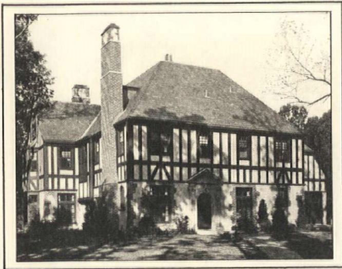
The half-timbering and massive medieval chimneys are the hallmark of the Tudor Revival houses. They often have slate or tile roofs; entrance doors are frequently of heavy plank construction, with only a small window—perhaps protected by bars. The pediment over the front door recalls the attempts by designers in Elizabethan England to adapt Renaissance forms to their medieval buildings.
