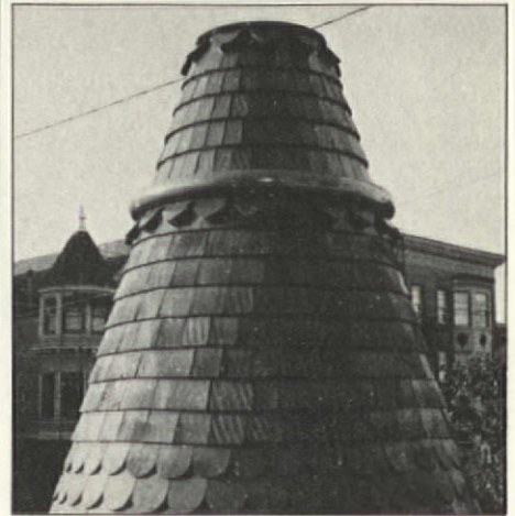
The structure was built on the ground, then hoisted -- so it had to withstand not only wind and weather, but also the stress of being lifted. An intermediate plywood membrane near the top provides extra strength. right top: Curved purlins brace rafters. right: Details are copied from an old photo.
