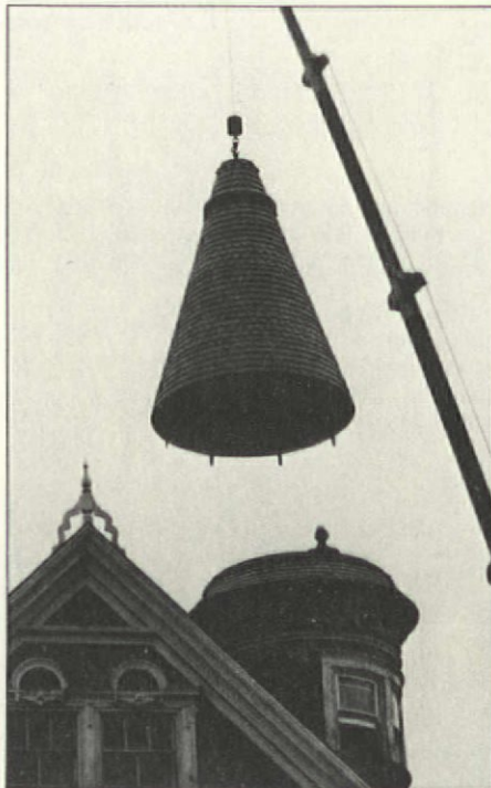
The 100-foot rig arrived at 8 am on a rainy December day. While the boom was stretched, the base of the tower was uncovered, and the rain was getting in. Early on, a chain had been buried in the top of the cone. It was hooked to the cable from the crane arm. Total time elapsed from start to finish: just 30 minutes. (That's Jim Tyler on a temporary platform inside the base.)
