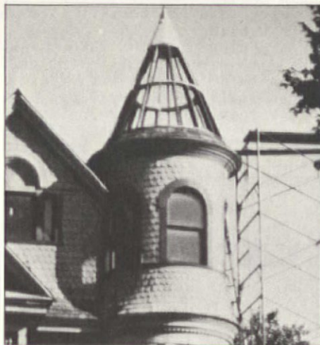
Neil Hiedeman built a new cone-shaped cap in three sections because he couldn't afford to rent a crane to position a finished roof, or enough scaffolding to build it all in place.
