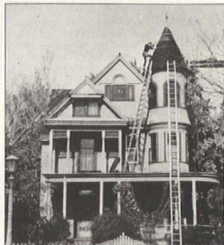
Neil Hiedeman built a new cone-shaped cap in three sections because he couldn't afford to rent a crane to position a finished roof, or enough scaffolding to build it all in place.
