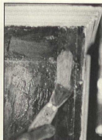
Stripper is removed with a putty knife and solvent.
