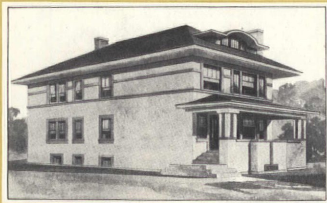
A 1909 Radford plan, this two-family frame house has the horizontal bands, wide flat eaves, and massive-columned porch that are characteristic of the Prairie style. The stuccoed exterior is another style trait.
