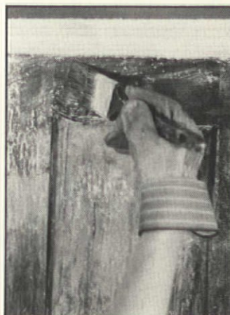
One coat of paint remover is applied for final clean-up.
