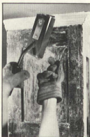
Paint left in joints and cracks is picked out after softening.
