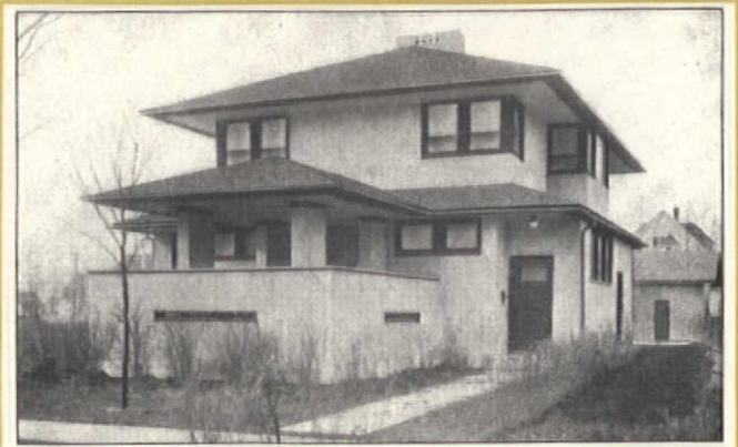
This 1910 stucco house takes the basic American Foursquare shape and adds Prairie-style details: horizontal wrap-around windows, low horizontal lines, open porch with oversize columns and broad roof.
