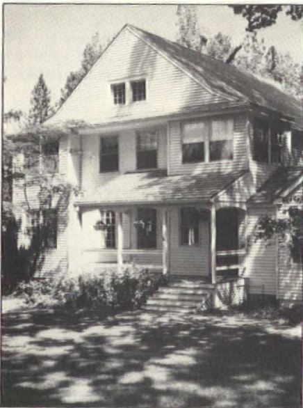
Copper shingles clad the roof of John and Susie Stone's 1904 house in Washington. The Mount St. Helens eruption sped up the formation of a rich patina on the copper shingles.
