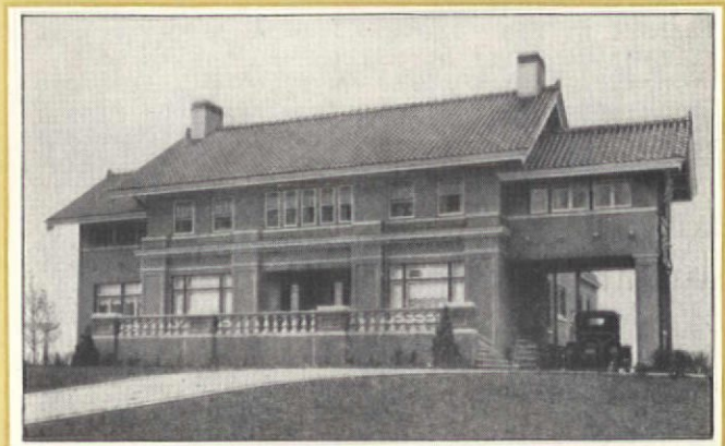
Basically a Georgian shape, this house has some classically influenced details. But Prairie touches show up in the massive pilasters projecting from the facade, as well as the horizontal bands and windows.
