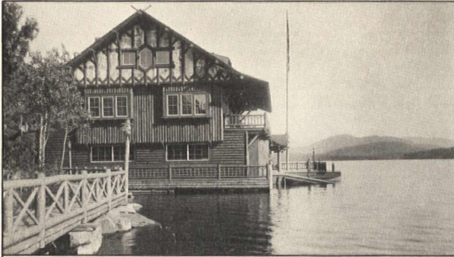
Adolph Lewisohn's camp, built in 1903-4, combined the Adirondack Rustic Style with German architecture. This boathouse was simulated log construction; its upper storey used birch bark to simulate stucco. (That's Mr. Lewisohn himself on the pier.)
