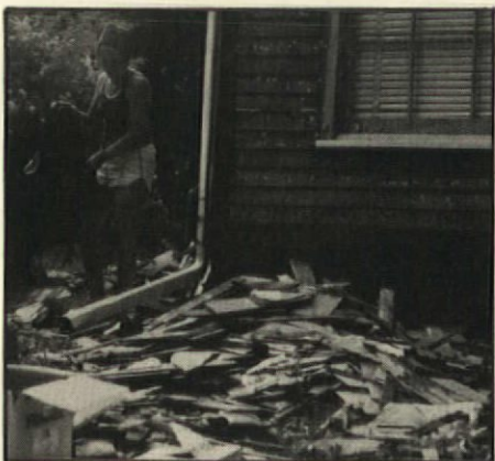
Top: Ridgely gathers some of the asbestos, wood, and paper that she and Robert ripped off the house. The row of black dots on the bottom clapboard are nails about to be pulled; the white dots are puttied nail holes. Right: The back of the house gets a coat of paint.
