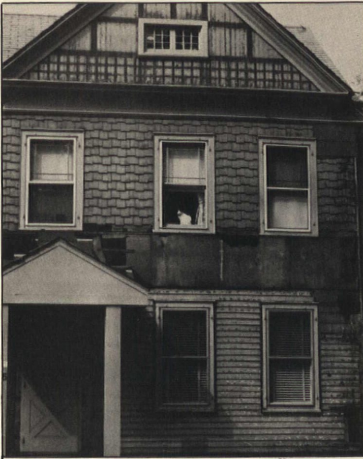
After un-muddling the house, they discovered some surprises, such as these phantom traces of ornamentation on the top storey.
