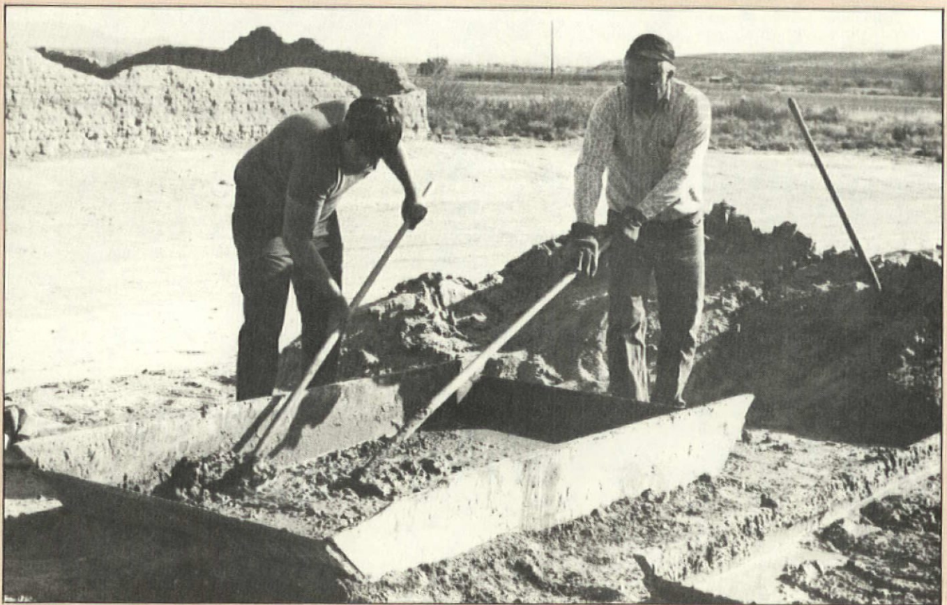
These two men are mixing the mud from which adobe bricks will be made.
