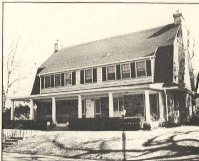
Tuscan columns elegantly contrast with the rough stone and shingle siding of this Revival house.
