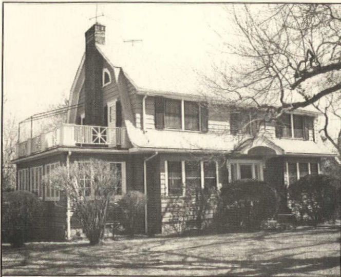
This typical plan-book Dutch Colonial Revival house, dating from around 1930, has a shed dormer across the front.
