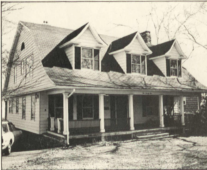
When porches became fashionable in the early 19th century, it was easy to place columns under the already-hanging, flared eave of a gambrel roof. This use of the eave became a common feature of Dutch Colonial Revival houses. (Note the echo of the roof's flared eaves in the three dormer roofs.)
