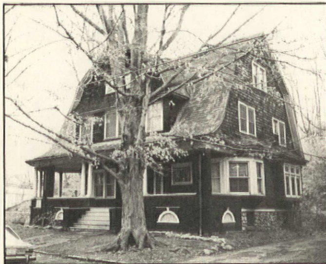
This turn-of-the-century, brown-shingled Revival house has a gambrel-shaped dormer and features a stained glass hall light, Palladian-influenced columns, and porch vents. Like so many houses in this style, it is a combination of rugged natural materials and classical details.
