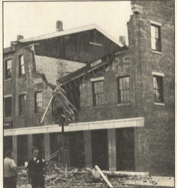
. . . the roof, floors, and front facade collapsed in a cloud of dust. Interior remuddling had seriously weakened the structure. The final insult occurred when workers poured concrete over the old wood floors. At that point, the building just gave up.
