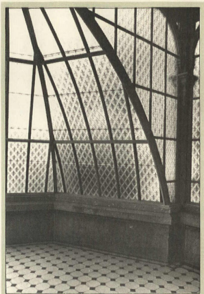
The leaded diamond shapes are created by the slightly corded surface of the acrylic window panes. Centered in each of the diamonds is a blue fleur-de-lys. (Note the way the panes overlap horizontally on the half-dome.)
