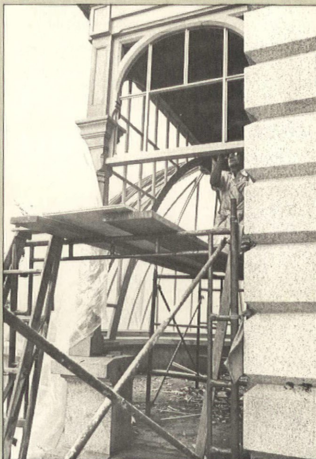
The millwork was built according to measured drawings made by Richard Bergmann. He used the surviving pieces of the conservatory as the basis for his designs.
