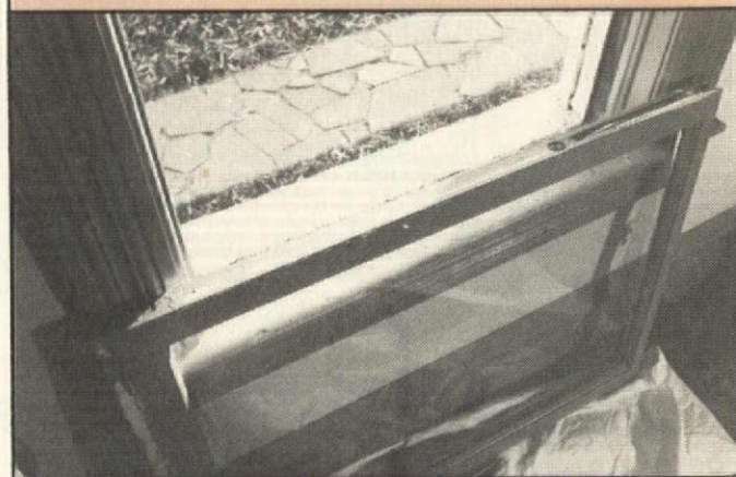
Above: Outside, a thin pry bar is carefully worked under the sash to break the paint film. Paint along the edges is then removed with a heat gun. Below: Here's the lower sash after being removed from the frame. Note the old sash cord in the upper right corner of the sash.
