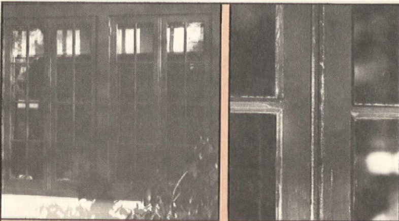
Casement windows are hard to weatherstrip. Those at left were rarely opened, and so were permanently caulked shut (right). Roll-type caulk can also be used for seasonal sealing.
