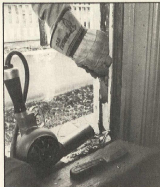
The heat gun is used to remove built-up paint from the sash run and center parting bead. The upper sash is almost always painted shut. Use a putty knife or a Red Devil "Windo-Zipper" to break the paint seal.
