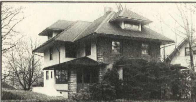
Because of its small ell and the resulting complications of the roofline, this house is technically not a Foursquare. Yet you can see how the architect took the basic American Foursquare design, added Prairie-style eaves and small ells and wings, and came up with a large suburban home.
