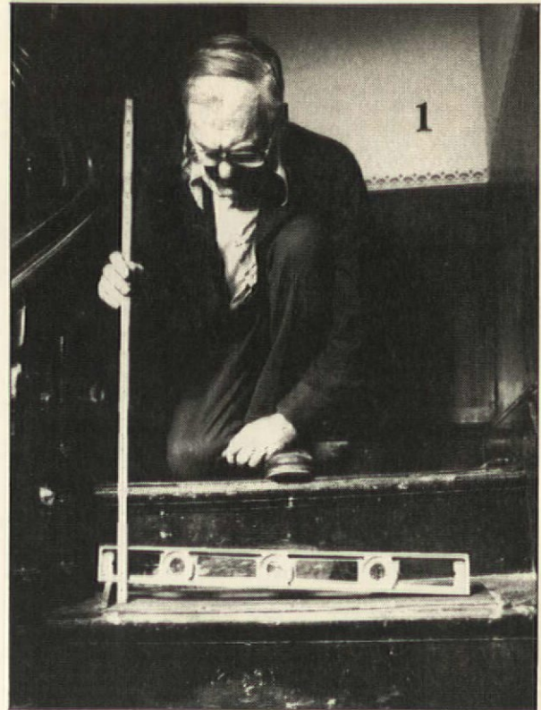
Above, retired master stairbuilder Harry Waldemar checks the level of the stair at the Old-House Journal offices. It had dropped 1-1/2 inches over a two-foot run, due partly to interior building settlement. Below, note treads pulling out of their housings in the wall string. "Wainscot" is just grained plaster.
