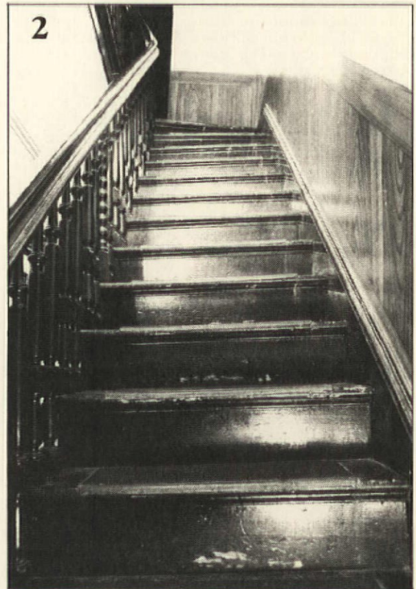
Above, retired master stairbuilder Harry Waldemar checks the level of the stair at the Old-House Journal offices. It had dropped 1-1/2 inches over a two-foot run, due partly to interior building settlement. Below, note treads pulling out of their housings in the wall string. "Wainscot" is just grained plaster.
