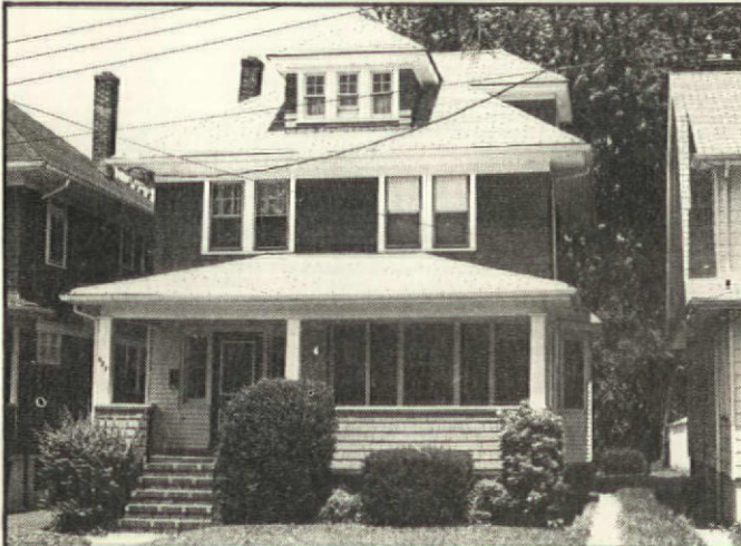
Here is the American Foursquare in one of its most familiar variations: Shingled exterior with dormers on three sides.
