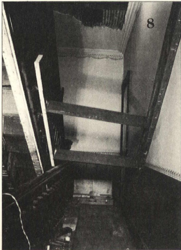
6 Plaster and wood lath were removed along the entire soffit under the stair. In the photo above, the cylinder braces are revealed. Ours is a typical row-house cylinder stair, or well stair. Below, the stair is braced against the partition wall opposite it. This operation pushes the steps back into their housings.
