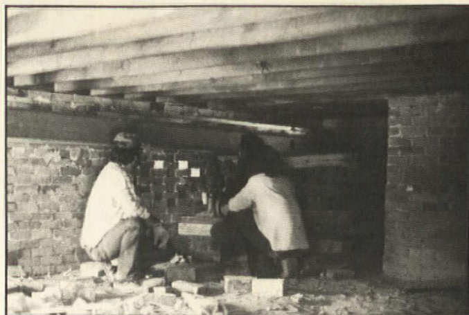
A mover operates one of the jacks under Tricia Greiss' house.
