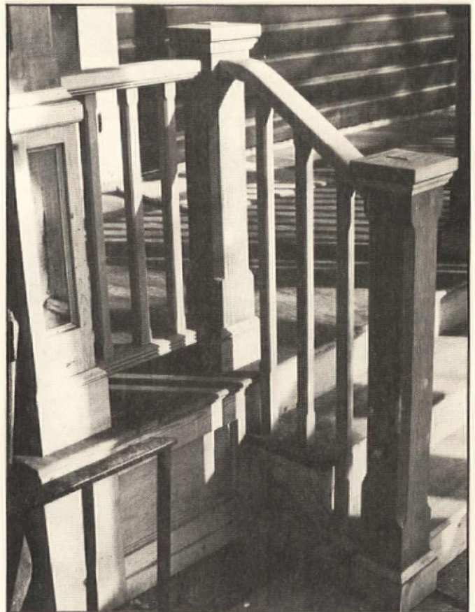
BETTER NEWEL CAP: Solid cap provides no opportunity for open joints. Porch would be better off, however, if it had latticework to vent the crawl space.
