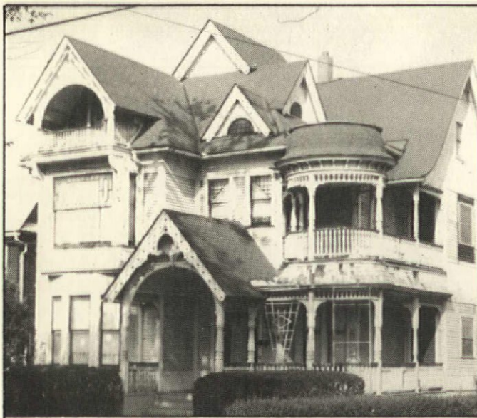
This "Queen Anne" illustrates how sash painted a darker color than the trim makes the windows look as if they are receding into the facade. Notice that the trim is lighter than the body color, although the body color is also light. The dark roof, probably a red or green, anchors the entire building nicely.
