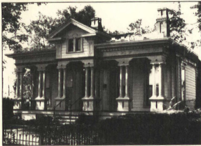
After Mr. Mosca's paint analysis, the Kemper House (Indianapolis) was painted light tan with salmon trim; decorative mouldings are red, sash and porch floor are dark brown, pilasters are light grey.
