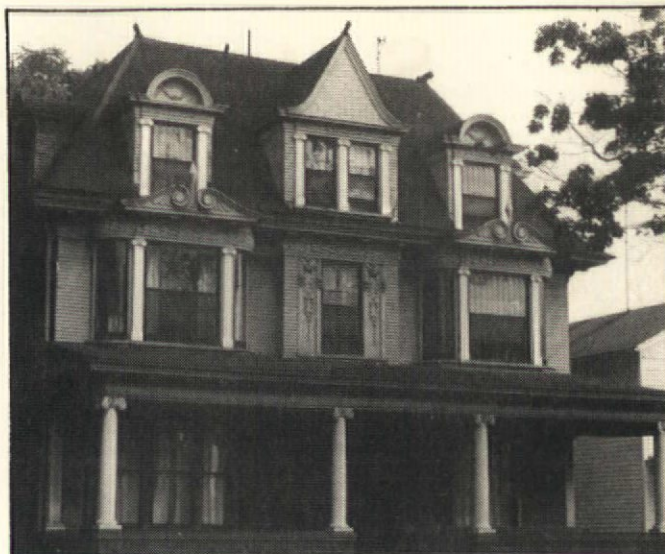
Elements of Queen Anne and Colonial Revival can be seen in this turn-of-the-century house. Notice how all the "classical" details (the Doric columns and pilasters) are painted white while the body and sash are darker.
