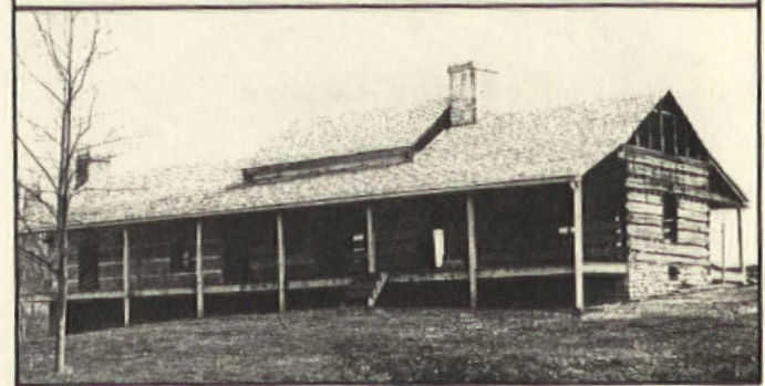
THE OLD WASH PLACE, Anderson County, Kentucky. Before restoration, above: The original portion, with the raised roof, was built as a 1-1/2 storey single pen. The pen on the left was added next, creating a saddlebag house. The double pen on the right was added later. It's uncommon to find all three building forms in one house. Below: During restoration.
