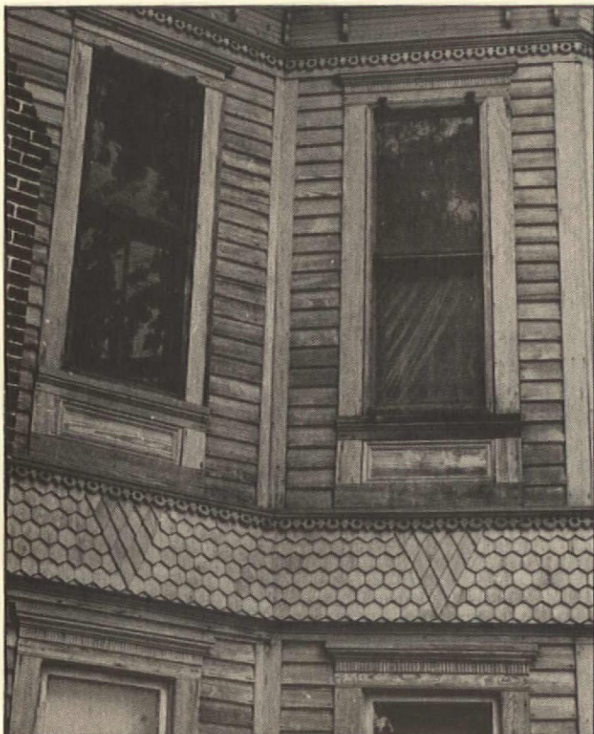
View Of Windows And Fancy-Butt Shingles
