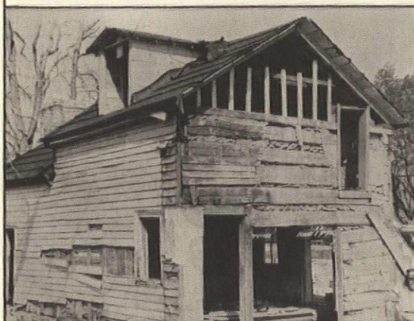
FOREST RETREAT TAVERN during restoration. Note beaded siding (top).
