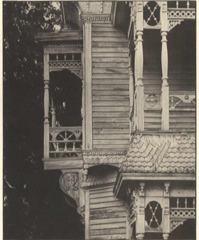
Bedroom Balcony And Second-Storey Porch
