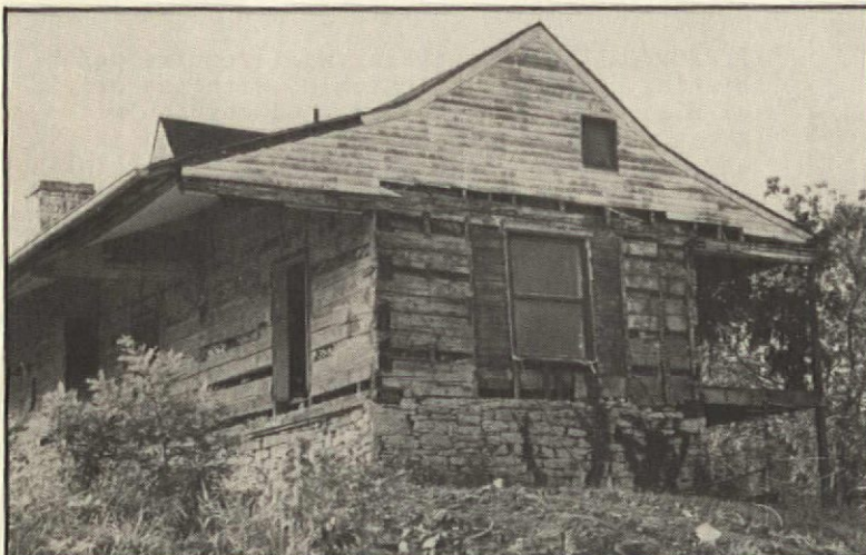
THE OUTLINE of an original chimney was revealed during restoration of the Old Wash Place. The cavity had been filled with a window--not uncommon. Right: The reconstructed chimney. Note wooden blocks wedged between logs in the chimney end. Also notice the long top log in the gable ...evidence that the porch is original.
