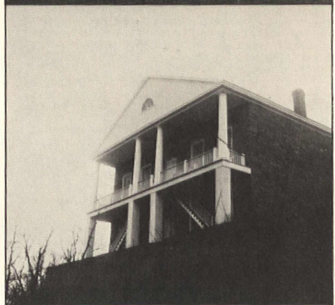
THIS EARLY COURTHOUSE, a random-rubble stone building in Greek Revival style, is also in the Register. Notice the pedimented portico with second-storey wood columns over brick and stone pillars on the first storey. Built 1848, Thebes, Illinois.
