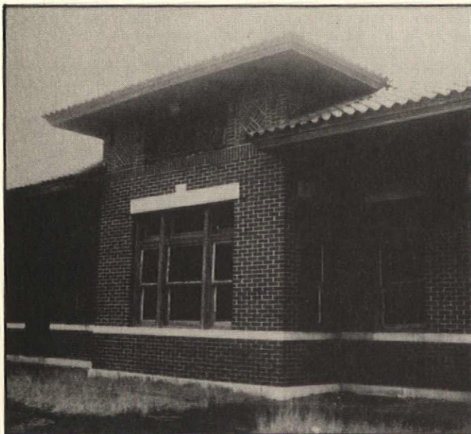
THE MISSOURI-PACIFIC DEPOT at Charleston, Missouri, is an example of a later building (1917) that has been listed. It's a typical small railroad station from the early 20th century at a once-busy transfer and trade center. Notable features include a hipped terra-cotta tile roof.
