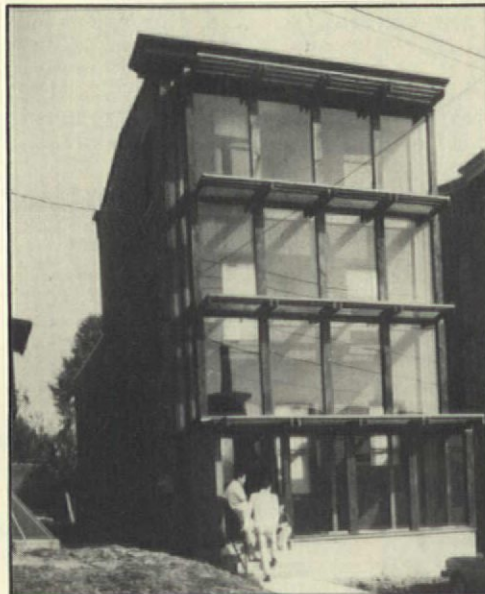
TECHNOLOGICAL TRASHING: The facade of this handsome house has been hidden behind an ugly glass wall that is supposed to act as a solar heat collector.
