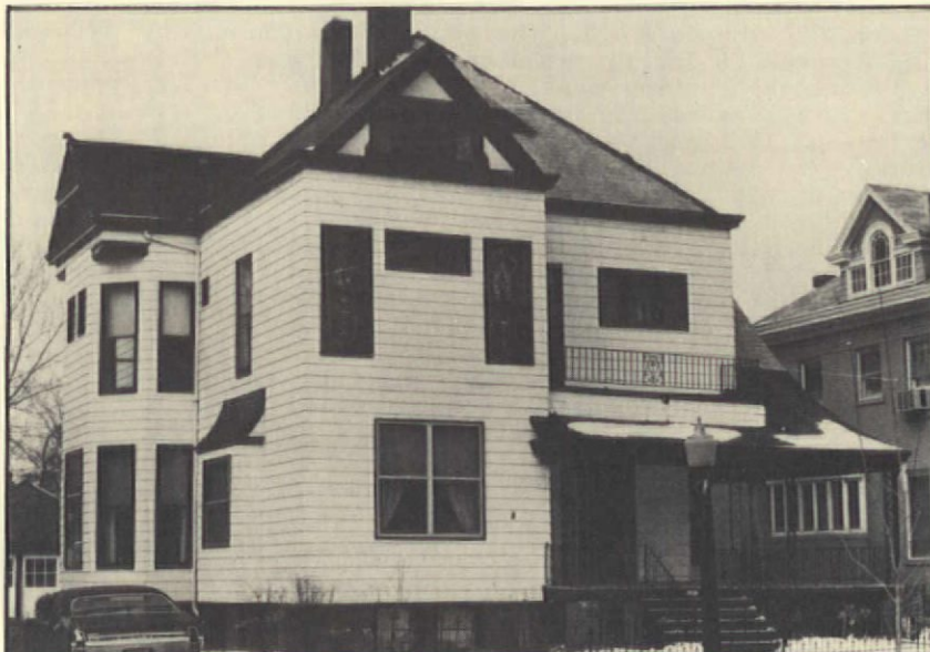
The aluminum siding had covered detailing, and the house has a flat monotonous look. Notice the incongruity of the modern wrought iron on porches.
